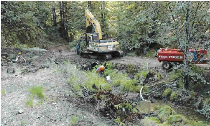
FIGURE 199. For larger streams, pump trucks, large pumps or multiple small pumps can be used to pump streamflow around project work sites. Here, a pump truck is used to temporarily divert flow in a fish bearing stream where dual culverts are being replaced with a rsilcar bridge. Young fish were removed from this fish bearing stream before project work started.
