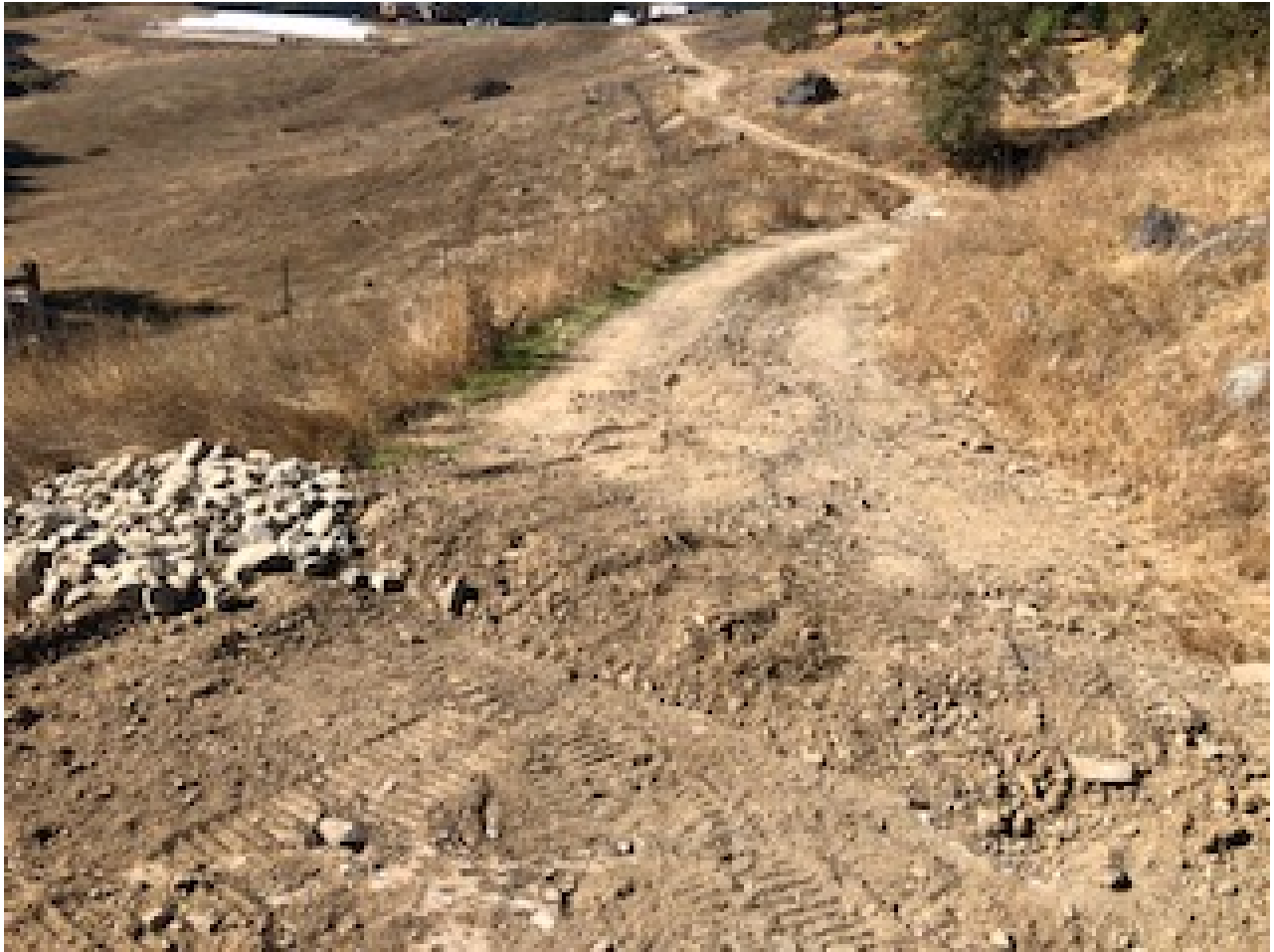
Figure 10: Installation of WB-7 in the foreground showing the waterbar and the riprap armoring at the outlet.
