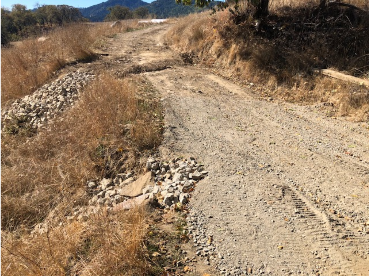
Figure 8: Facing west toward residence, roadbase RB-1 and waterbar WB-4 upslope.
