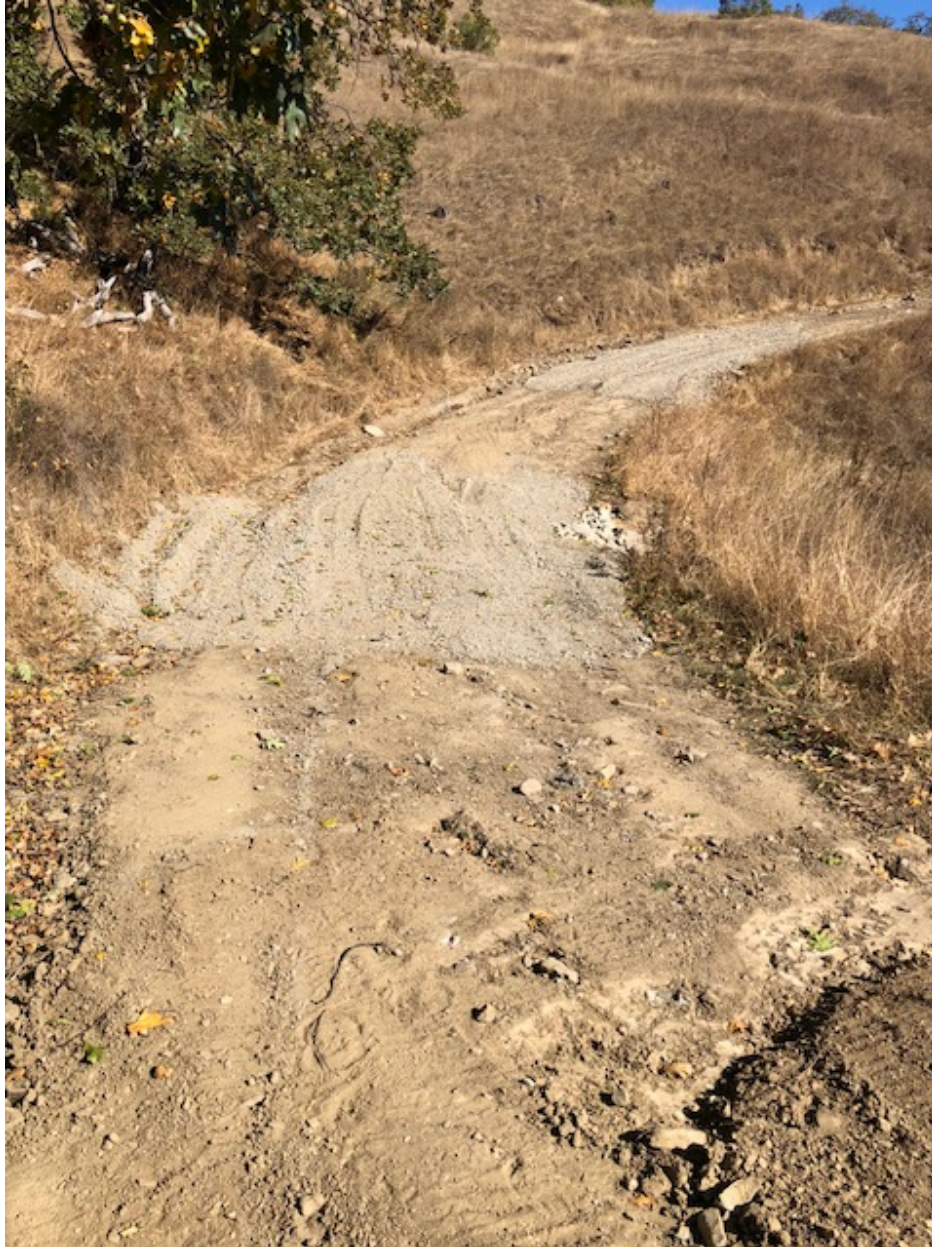
Figure 7: Installation of roadbase at the sites of stream crossings. RB-1 in foreground, RB-2 in background.
