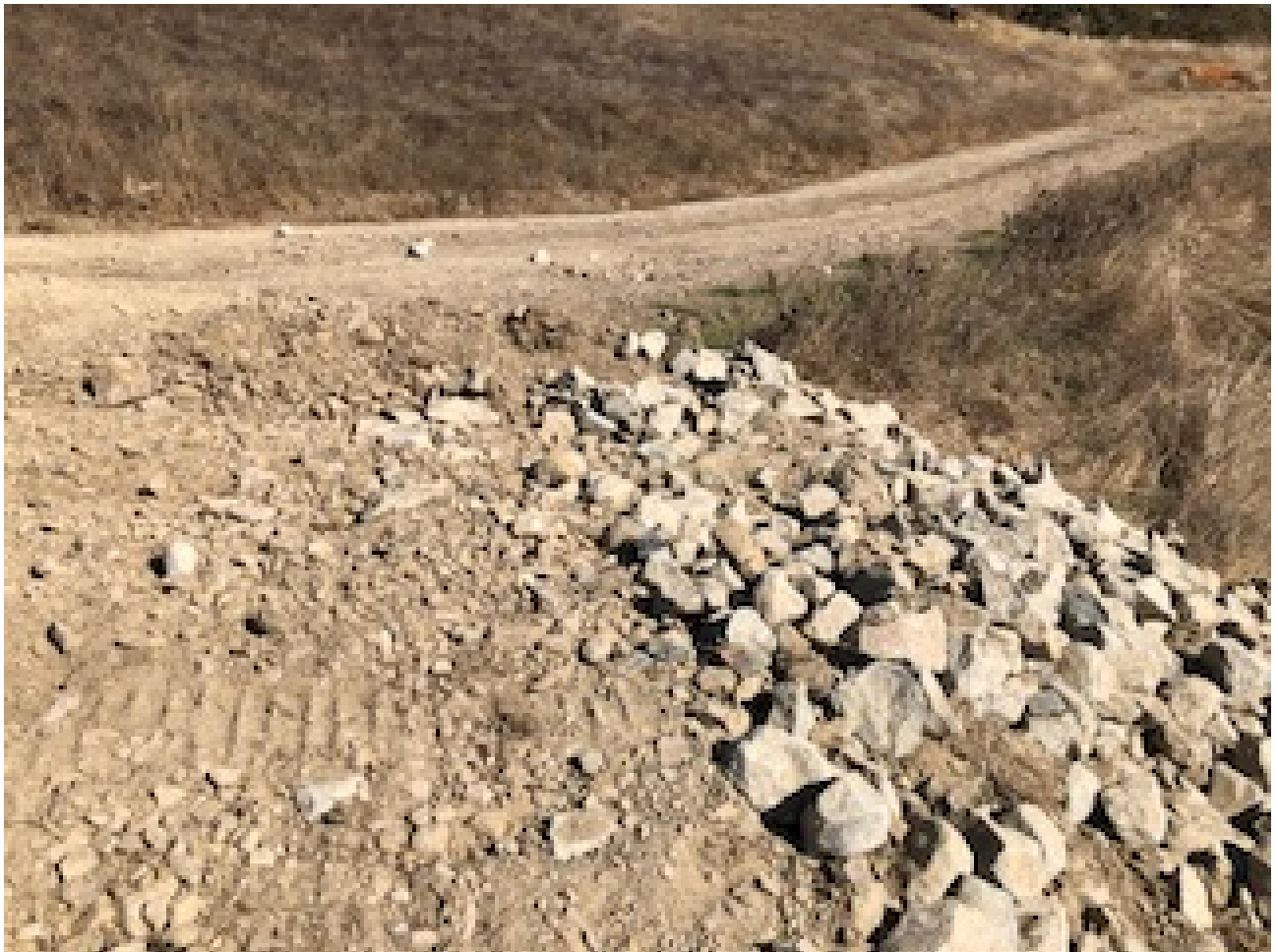
Figure 2: Close up photo of the riprap armoring of WB-1 outlet.
