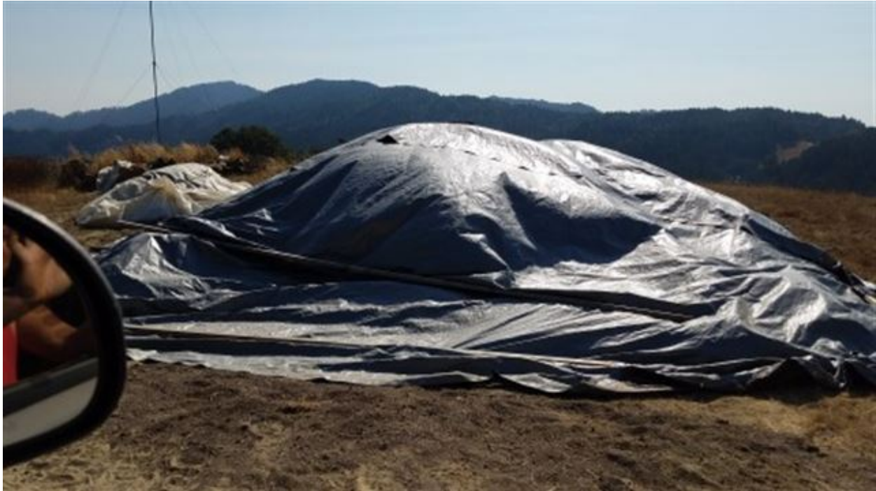
Soils removed from CA-3 at staging area to the east of the solar shed
