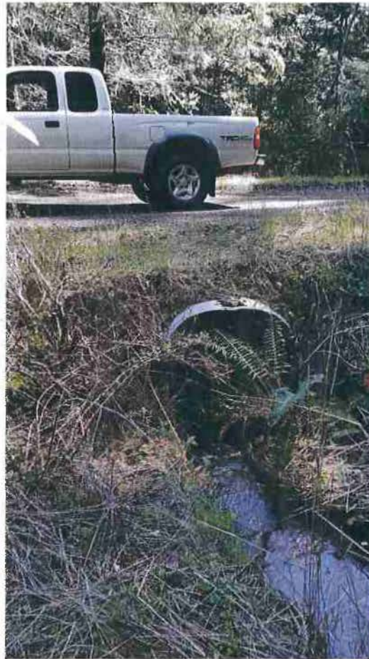
Figure 22. Photograph showing road point RP21 which is a 48 inch culvert on a class II watercourse in good condition.
