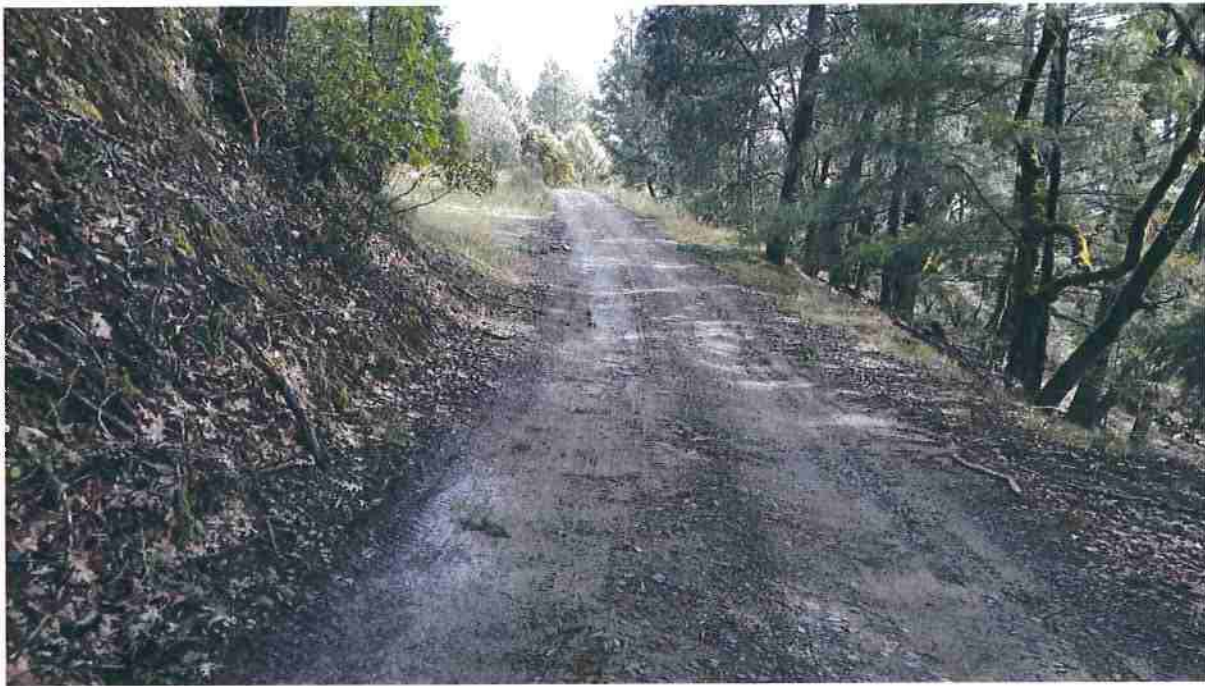
Figure 46. Photograph showing a steep section of roadway where the road slope is between 16 and 20% Located between RP51 and RP50. The slope is short and there are good pullouts on either side of the steep short steep section. The pullout located at RP51 can be seen on the left just before the steep section.
