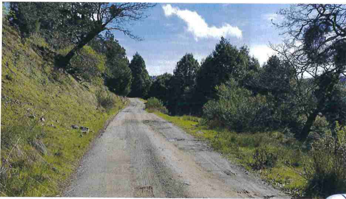
Figure 27. Photograph showing road point RP25, a good pullout north-east of a narrow section of roadway (RP26).
