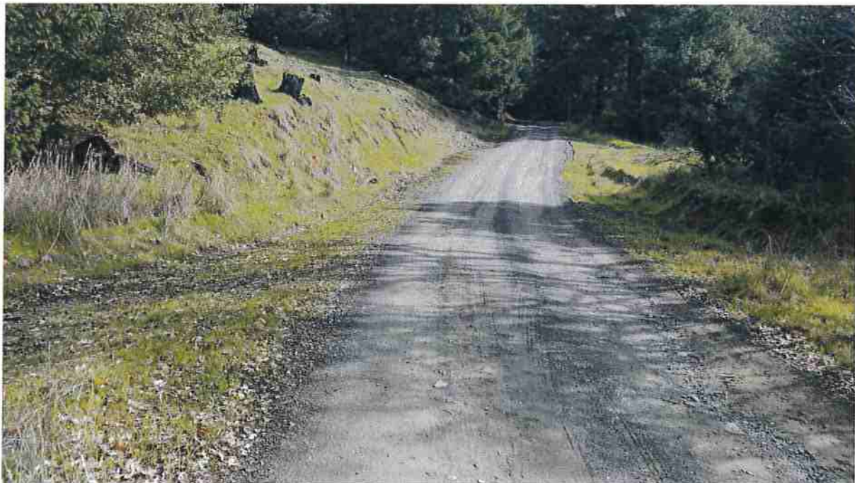
Figure 45. Photograph showing a pullout and gate located at road points RP50 and RP49.
