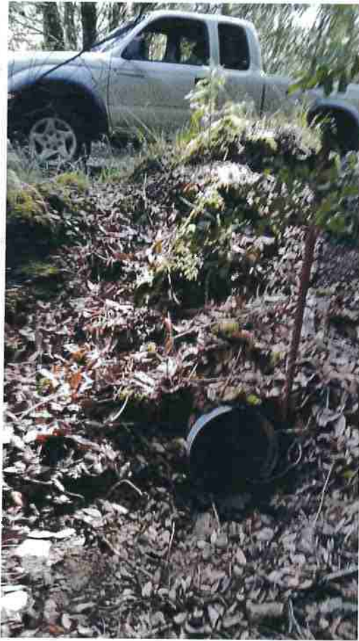
Figure 33. Photograph showing road point RP35 is a 12" culvert in good condition on a class III watercourse
