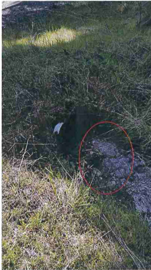
Figure 19. Photograph showing road point RP18 which is a 24 inch culvert on a class III watercourse that needs debris cleared from the inlet. The culvert is in good condition.
