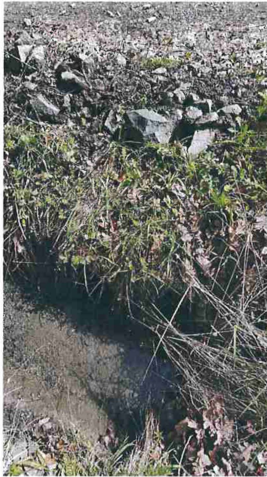
Figure 8. Photograph showing road point RP6 which is a drainage relief culvert..
