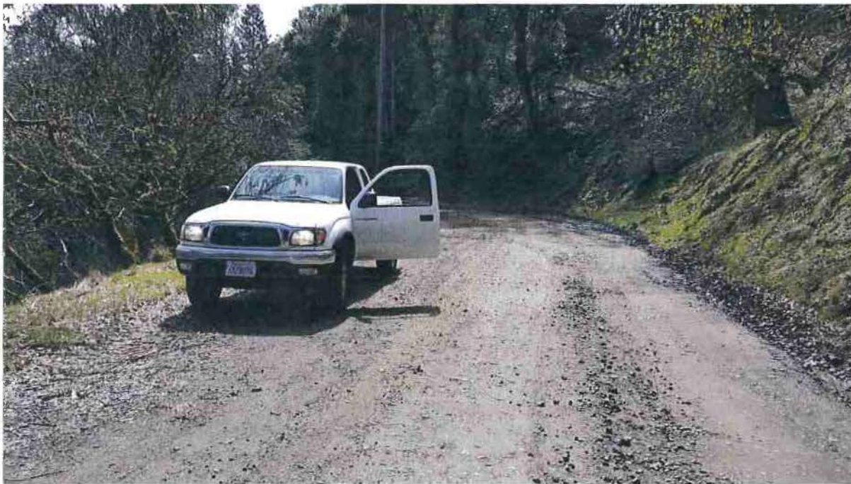
Figure 2. Photograph showing road point RP1 which is a good turnout.
