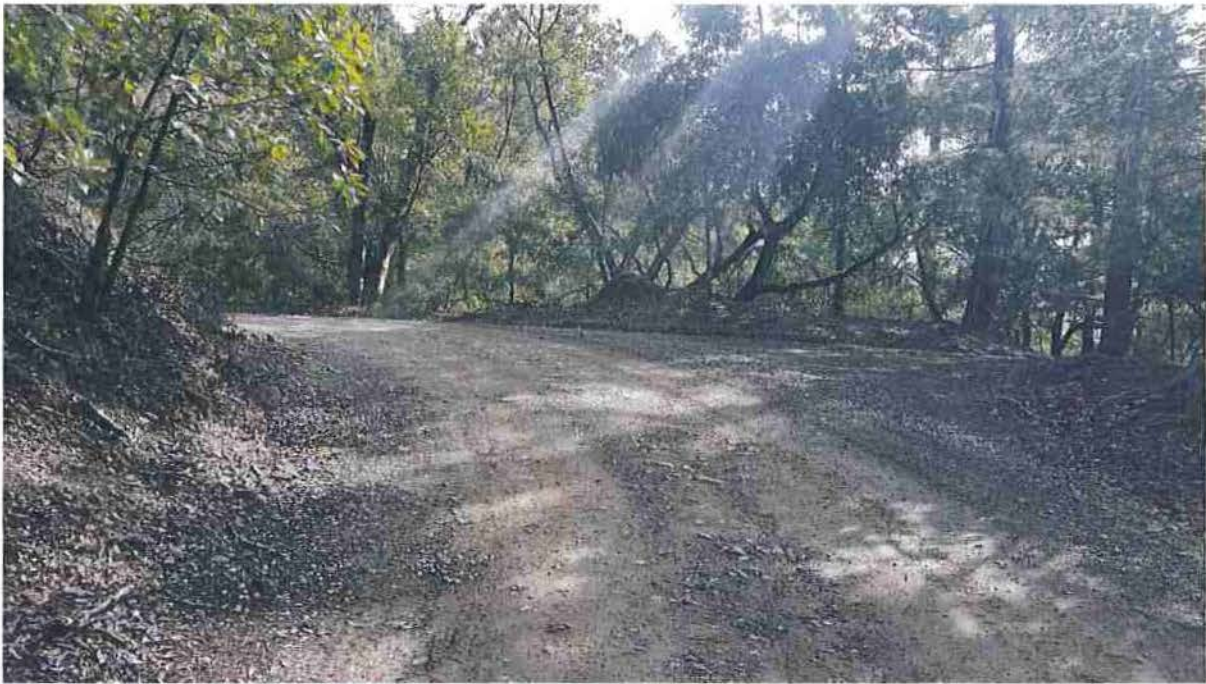
Figure 42. Photograph showing a good pullout located at road point RP45.
