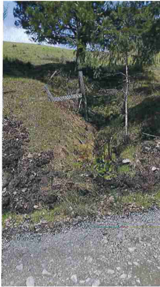
Figure 4. Photograph showing the class three stream that is diverted to road point RP2 which is an onstream culvert in good condition. The inside ditch catches the class III stream and diverts it to the culvert. Future work on the culvert will need a CDFW permitting.
