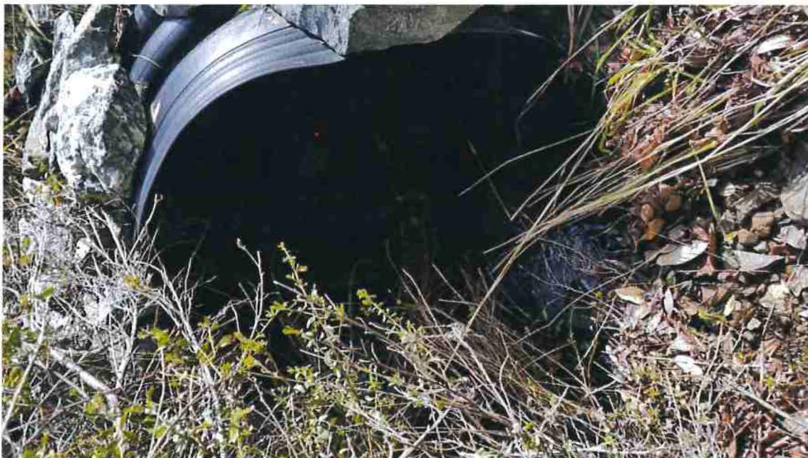
Figure 31. Photograph showing road point RP32 showing a onstream culvert in good condition on a class II watercourse.
