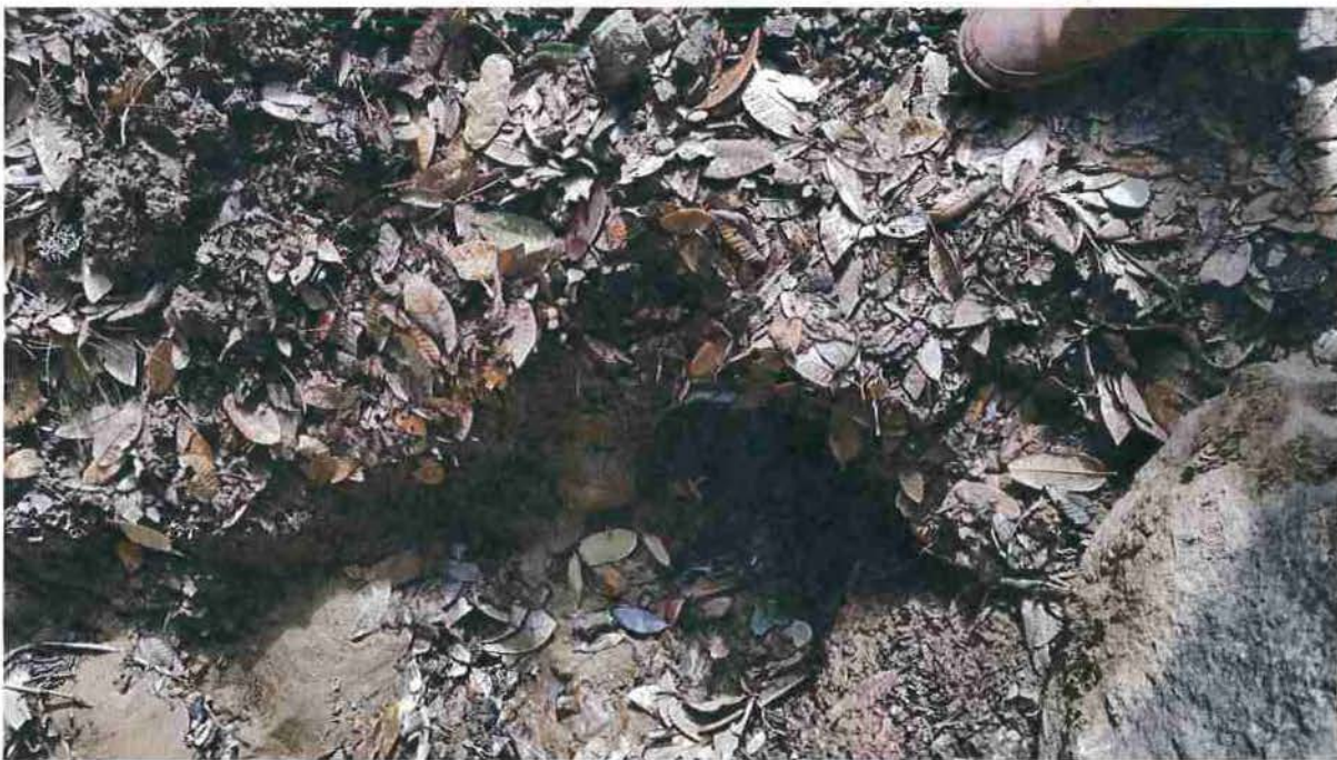
Figure 3. Photograph showing road point RP2 which is an onstream culvert in good condition. The inside ditch catches the class III stream and diverts it to the culvert.
