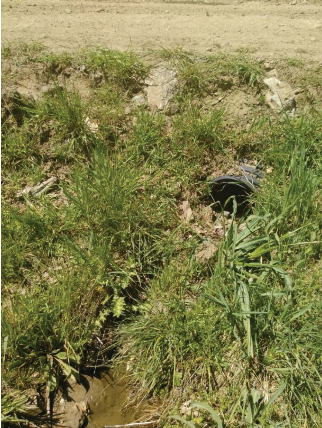
Outlet of CV-1 from downstream
