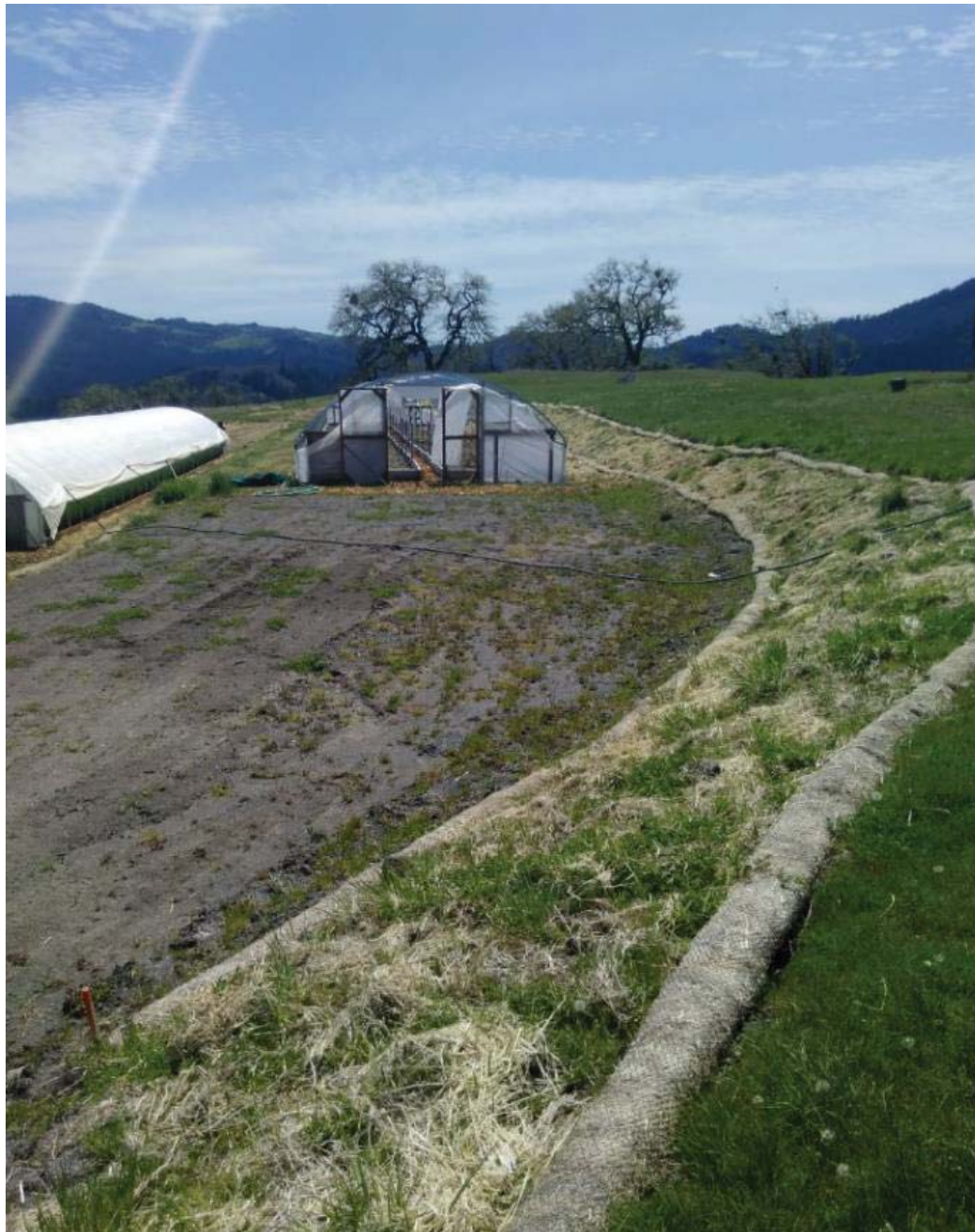
Upper greenhouse on the west side of CA-5. Slope is revegetated, strawed and lined with waddles. Aisles and front of greenhouse covered in bark.
