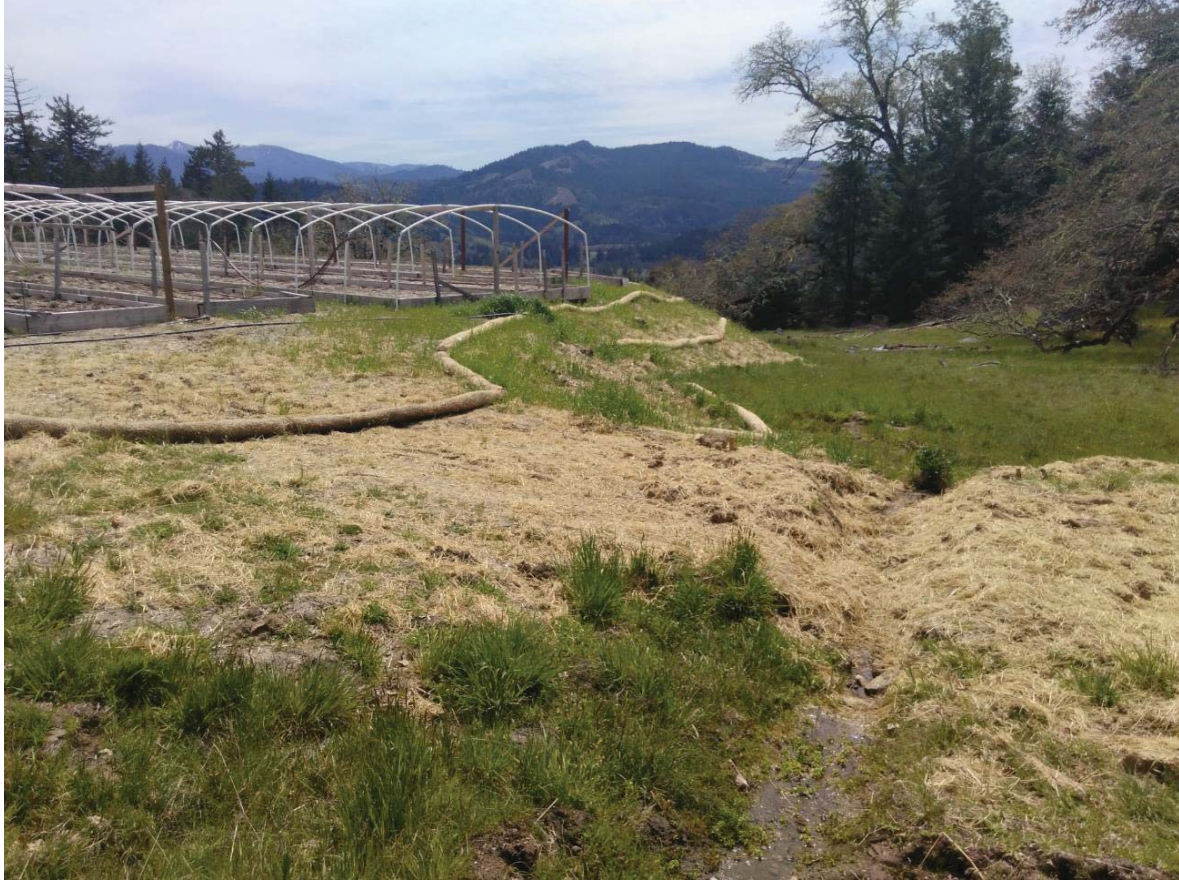
Class III drainage that formerly had a 4" culvert installed at access driveway. Culvert has been removed and road has been decommissioned. Retake of OP-3
