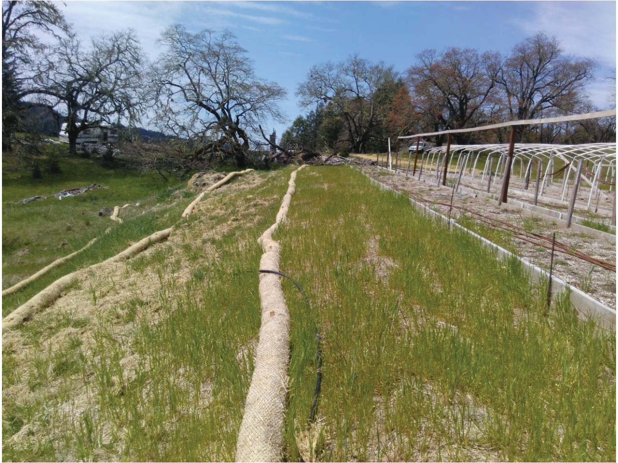
Strawing, waddles, and revegetation of southern edge of CA-3
