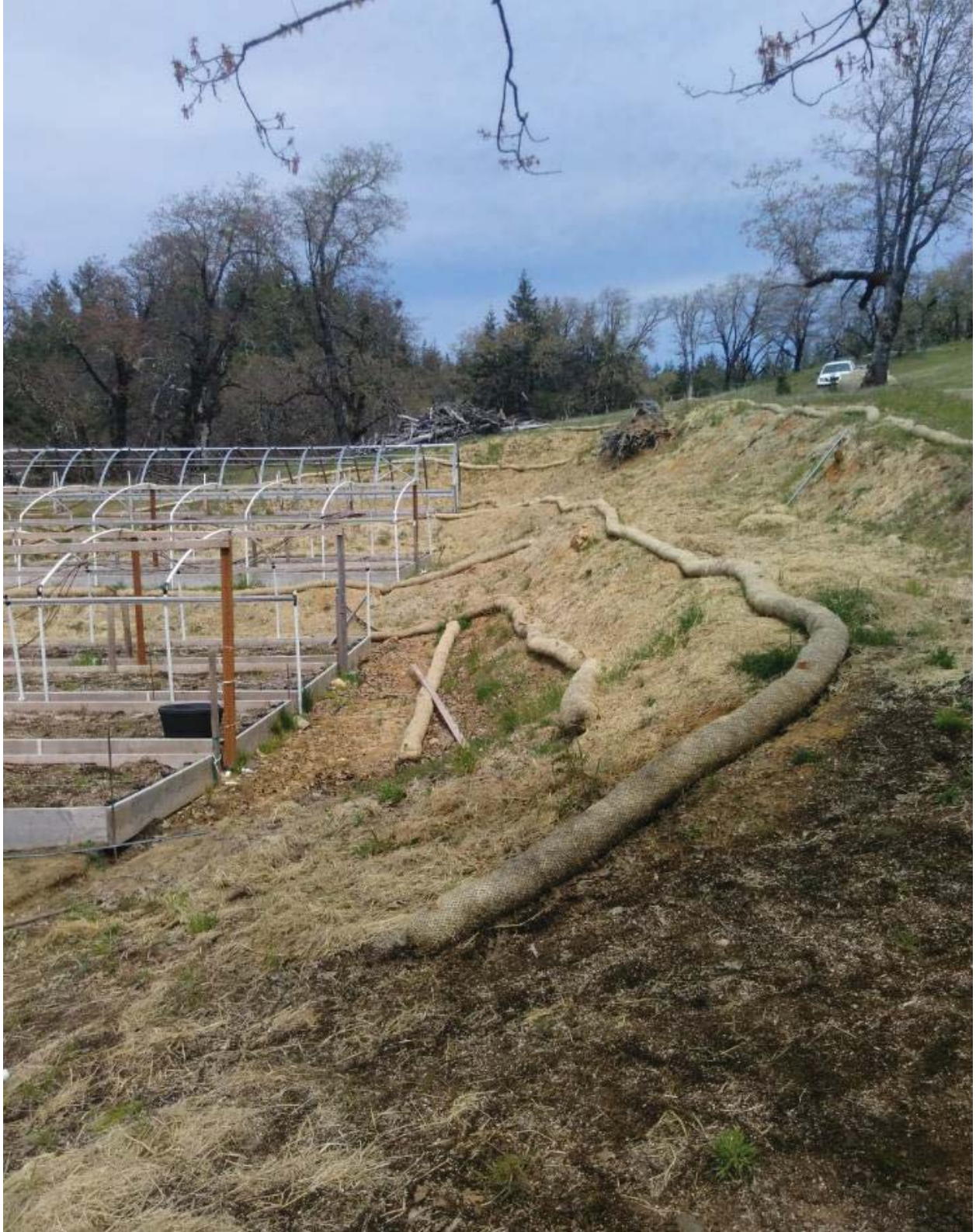
View from the SW corner of CA-2
