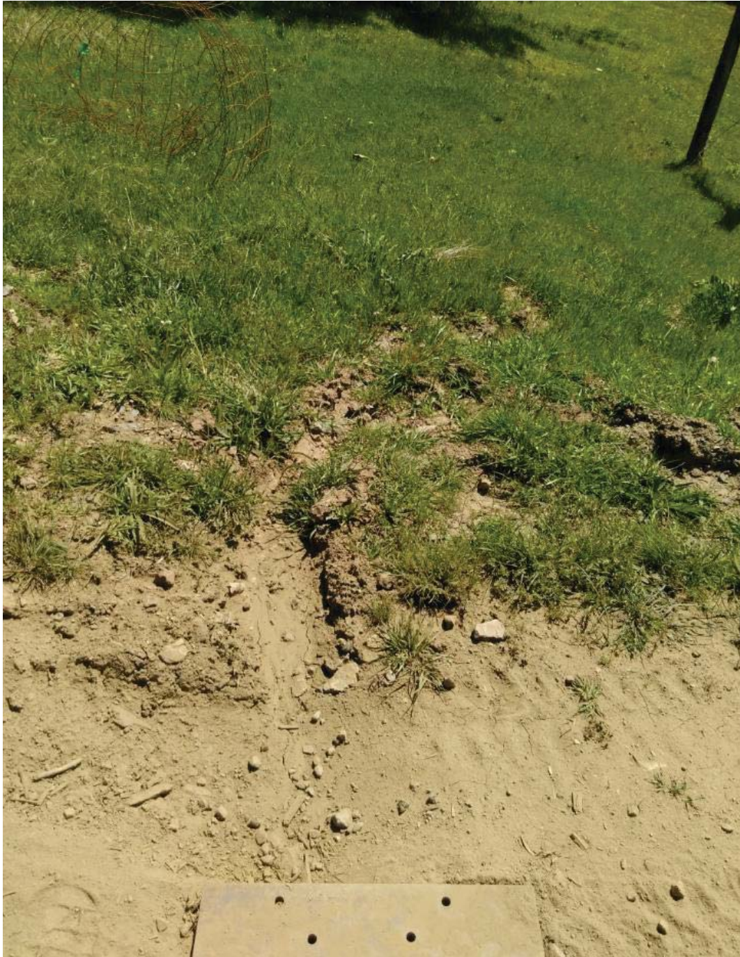
CV-3. Outlet of the dip that conveys the seep across access road
