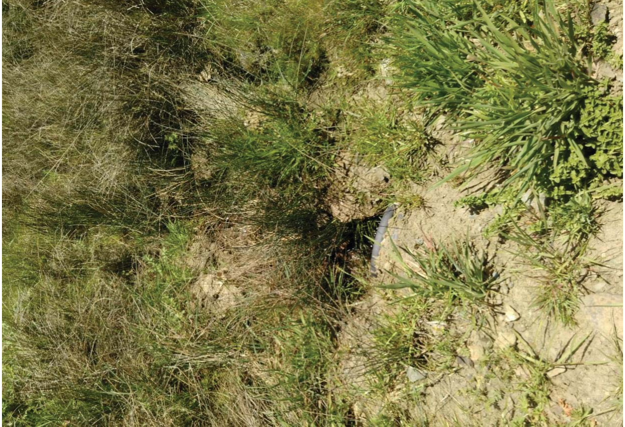
Outlet of CV-2 viewed from above
