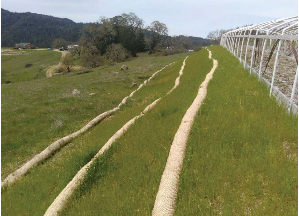
Downslope of CA-1 showing waddles and native vegetation
