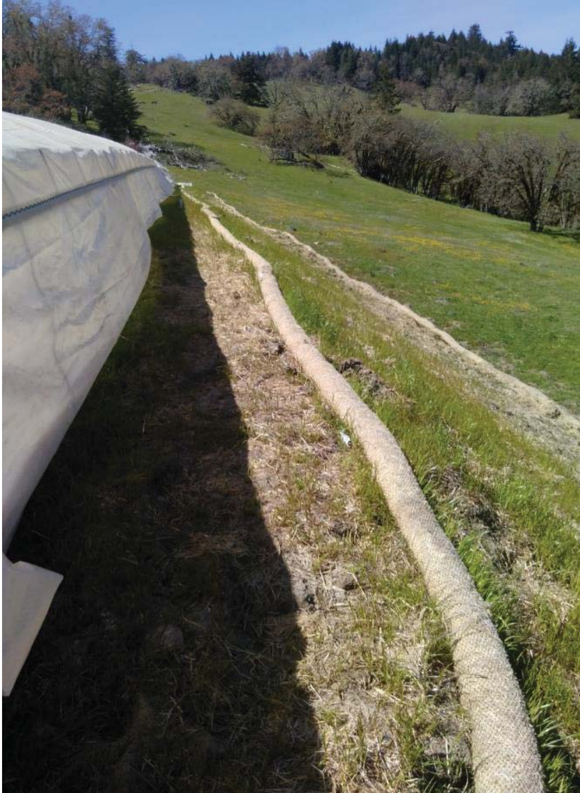
Waddles, straw and revegetation on the north edge of CA-6
