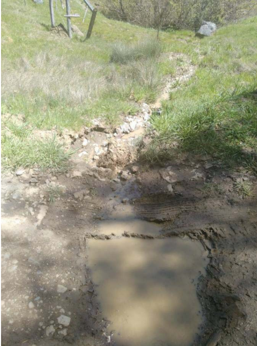
AC-1. Looking downhill from roadway. Inadequate drainage of access road and contributing hillside seeps causing erosion and sediment transport. Road improvements and armored crossing proposed.
