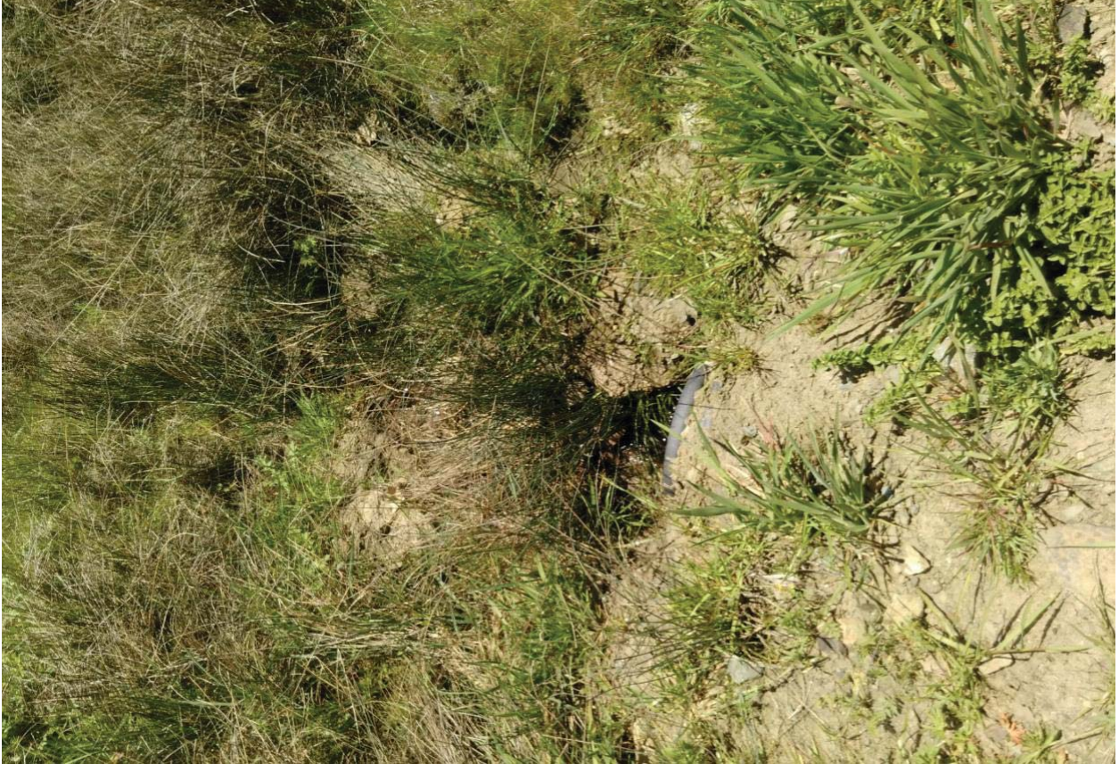
Outlet of CV-2 viewed from above
