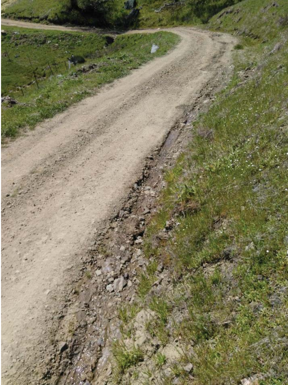
Road segment to be improved and hydrologically disconnected. CV-2 is visible in the background at the bend in the road.
