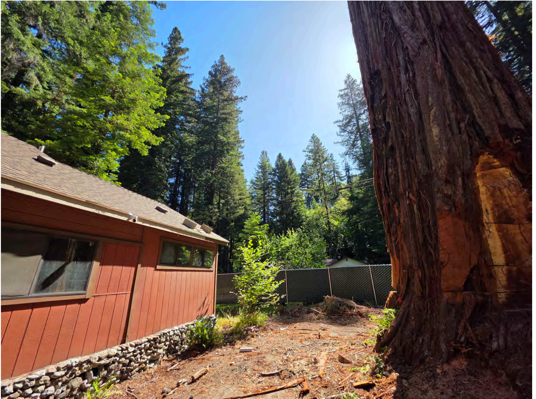
Viewing easterly. (photo date 05/19/2026)
