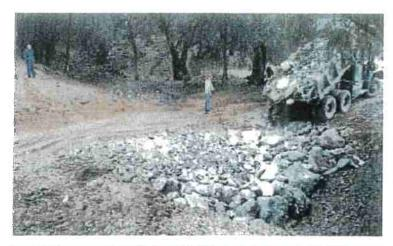
FIGURE 121D. West graded rock armor to then be chiled into the structure and spread across the breadin of the U-shaped stream crossing, and about the chird the way up the roadbed, so that streamfow will only flow over or come in contact with resistant armor material. The armor must be spread and compacted across the design width of the expected flood flow channel width so peak flows with not flank the armored structure.
