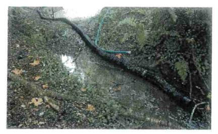
FIGURE 107. Flex pipe stream diversion around a road construction site. The inlet to this 6 inch diameter flex pipe inlet collects clear streamflow from a retention dam above the project site and gravity feeds it around the project area and back into the natural channel downstream from construction work (see photo).
