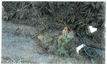
FIGURE 198. Sand bag retention dam on this small stream was used to pend streamflow so it could be pumped around a culvent installation site. The green intake hose is exceed to keep out tooks and debris while the red pump hose extends several hundred feet around the project work area.
