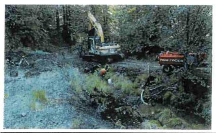
FRIURE 199. For larger streams, pump trucks, large pumps or multiple small pumps can be used to pump streamflow around project work sites. Here, a pump truck is used to temporarily direct flow in a fish bearing stream where dual culverts are being replaced with a railcar bridge. Young fish were removed from this fish bearing stream before project work started.
