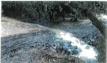
FIGURE 121E. Two weeks after this authored fill was constructed, a storm flow event occurred and the structure maintained its function and integrity. The road approaches had not yet been compacted or surfaced with road rock.
