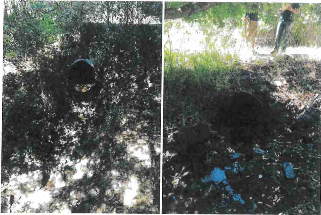
Pictures 6 and 7: These are pictures taken at Map Point 3, the existing 42-inch culvert proposed to be upgraded to a 54-inch diameter culvert. The picture on the left shows the outlet and the picture on the right shows the inlet. Photo date Sept. 2016.
