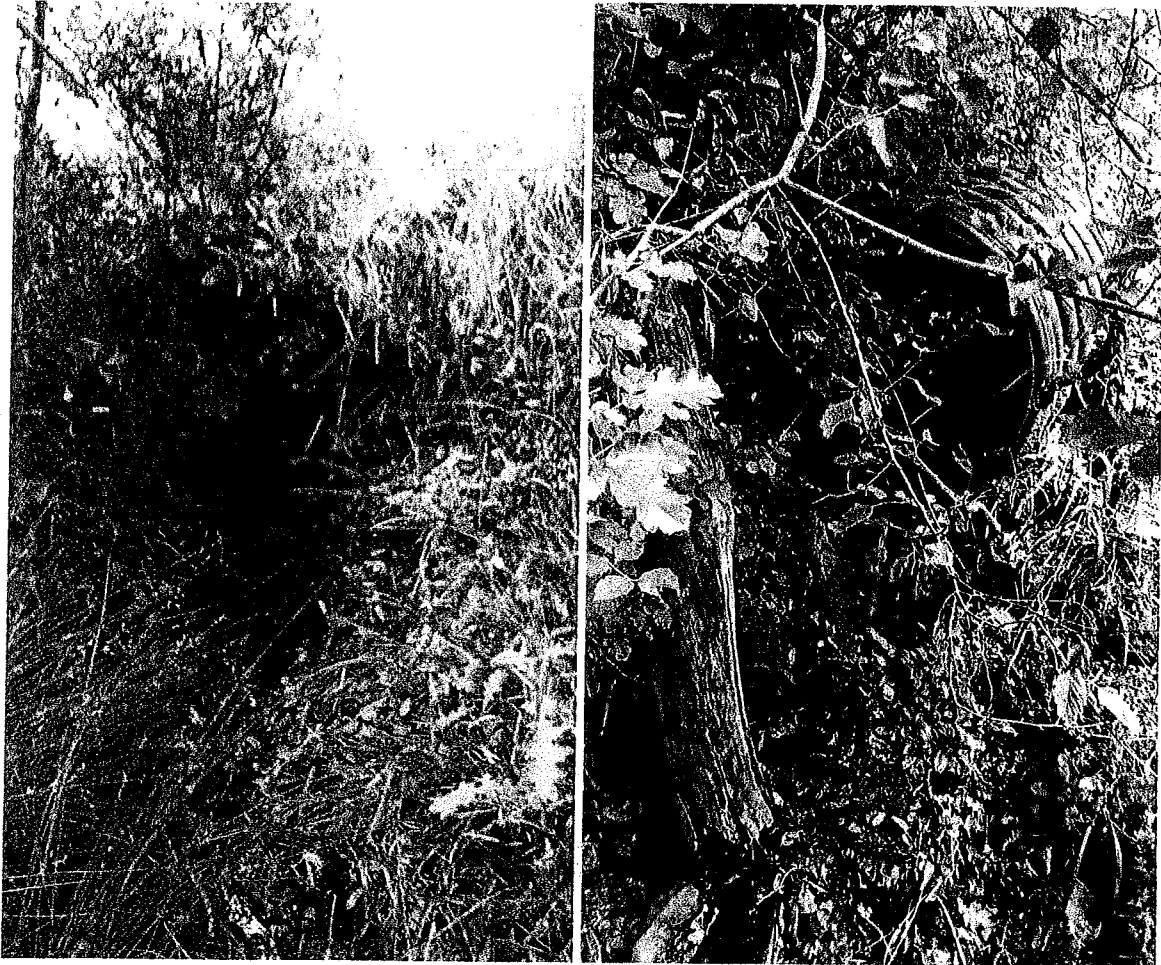
Pictures 11 and 12: These are pictures taken at Map Point 6, the existing 24-inch culvert proposed to be upgraded to a 36-inch diameter culvert. The picture on the left shows the inlet and the picture on the right shows the outlet. This is a "Low" priority site. Photo date 4/19/17.
