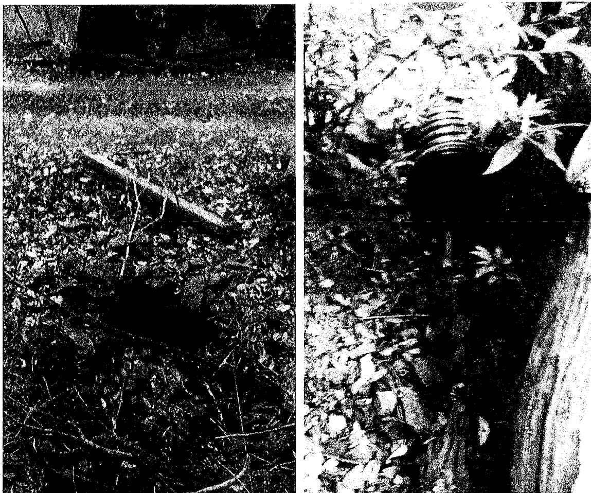
Pictures 13 and 14: These are pictures taken at Map Point 8, the existing 12-inch culvert proposed to be upgraded to a 36-inch diameter culvert. The picture on the left shows the inlet and the picture on the right shows the outlet. This is a “Low” priority site. Photo date 4/19/17.
