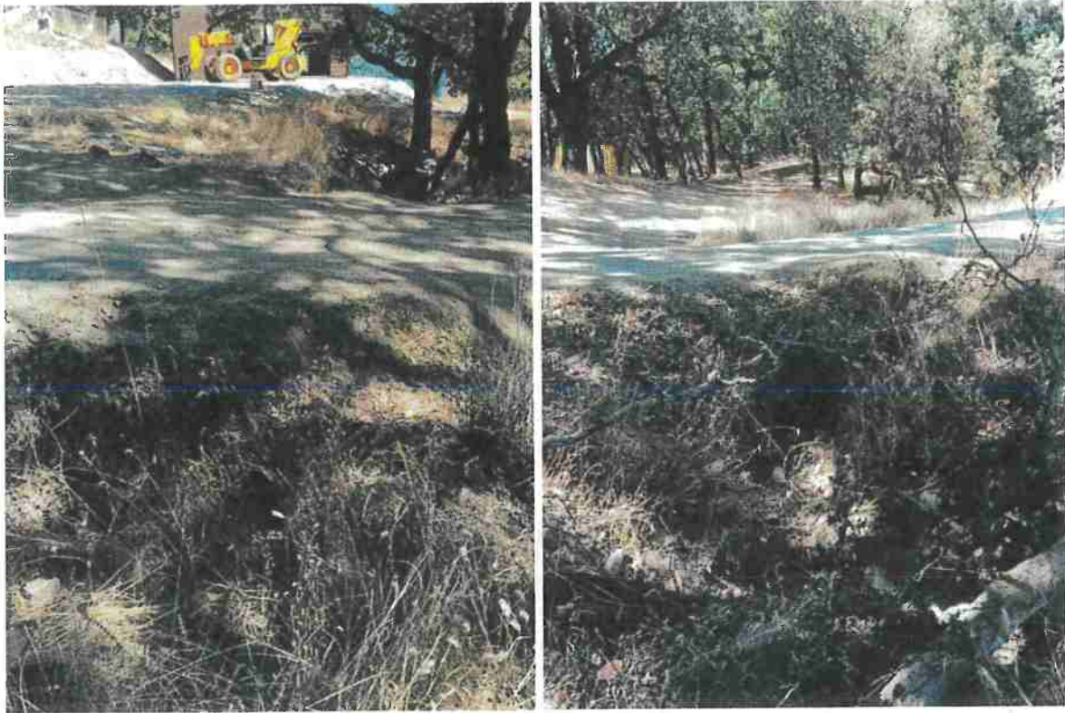
Pictures 4 and 5: These are pictures taken at Map Point 2, the existing 12-inch culvert proposed to be upgraded to a 24-inch diameter culvert. The picture on the left shows the inlet and the picture on the right shows the outlet. Photo date Sept. 2016.
