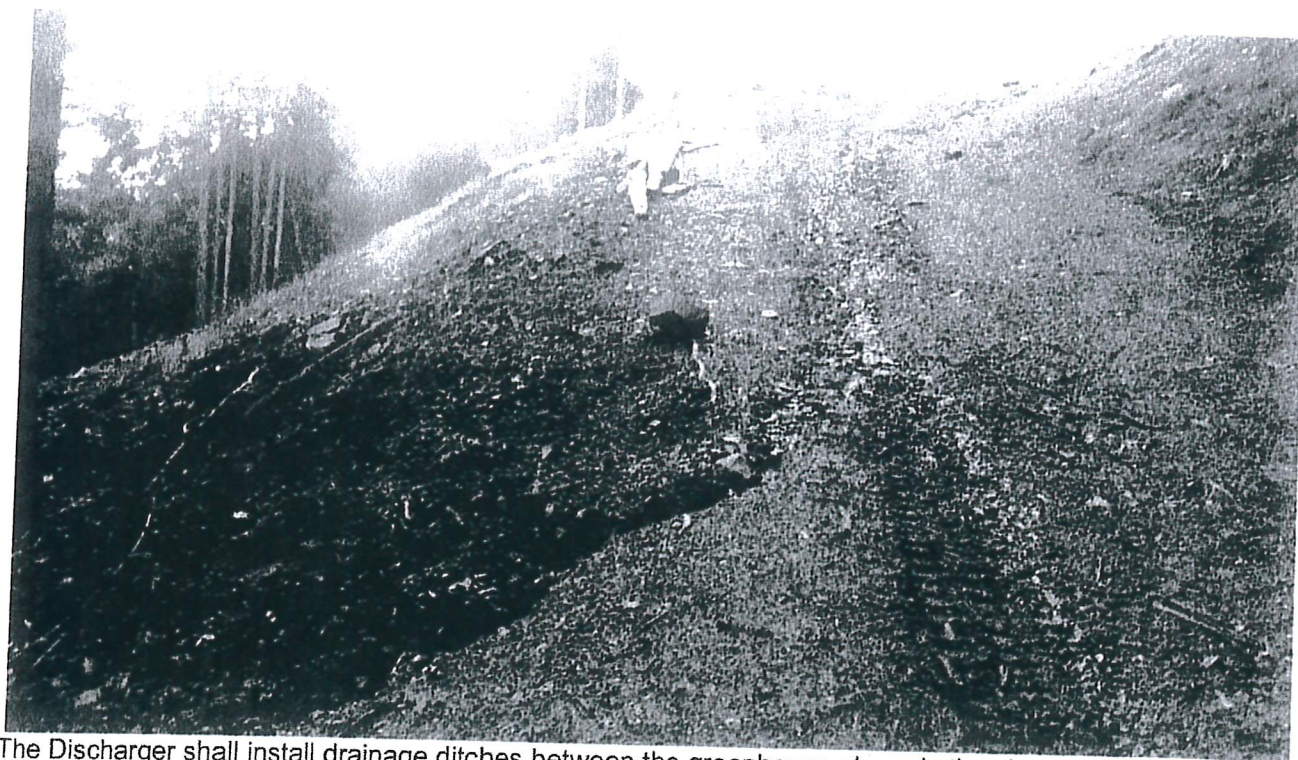
Road Point 10: Install a waterbar here to drain the road and surface flows coming from the greenhouses around the corner to the left in the photo. This segment of road, between Road Point 4 and Road Point 6 also needs to be rocked.
