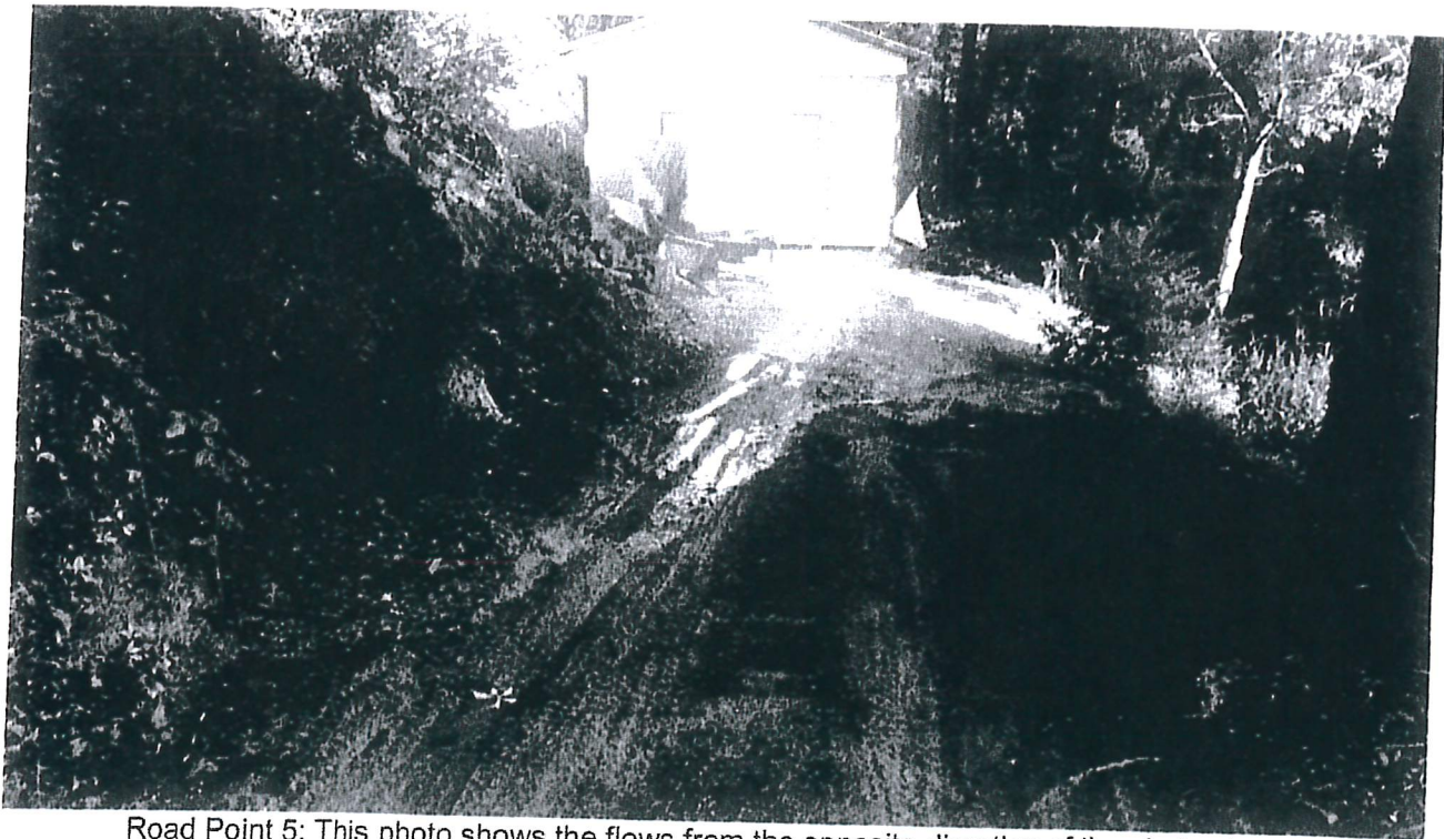
Road Point 5 looking towards Road Point 4: This picture shows road surface flows coming from the outlet flows of DRC 4 draining down and across the roads surface. The Discharger shall install an inside ditch along the cutbank on the right of the road in the photo to capture the surface flows coming from DRC 4 and install a ditch relief culvert where the water crosses the roads surface.
