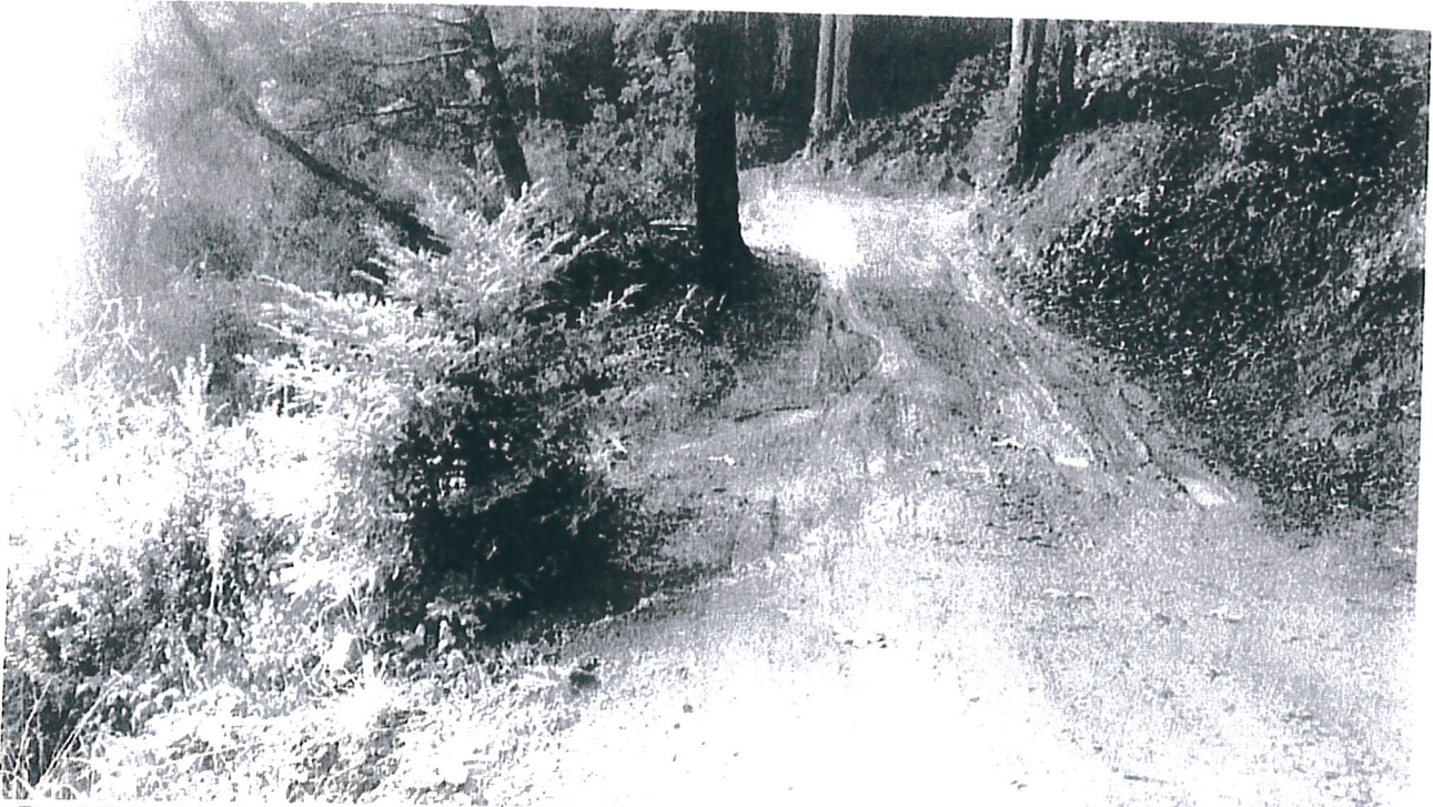
Road Point 5 looking towards Road Point 4: This picture shows road surface flows coming from the outlet flows of DRC 4 draining down and across the roads surface. The Discharger shall install an inside ditch along the cutbank on the right of the road in the photo to capture the surface flows coming from DRC 4 and install a ditch relief culvert where the water crosses the roads surface.
