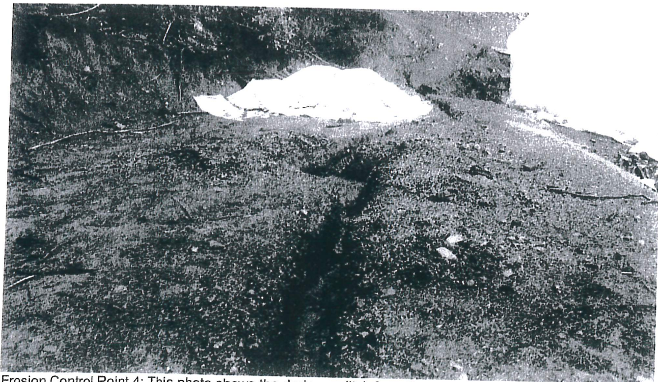
Erosion Control Point 4: This photo shows the drainage ditch from the cultivation area. The Discharger shall remove or properly contain all potting soils located near these drainage ditches and spread chipped slash or woody debris over any remnant soils.
