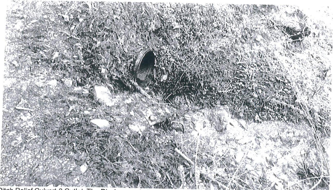
Ditch Relief Culvert 3 Outlet: The Discharger shall rock armor the outlet of this ditch relief culvert per attached specifications.
