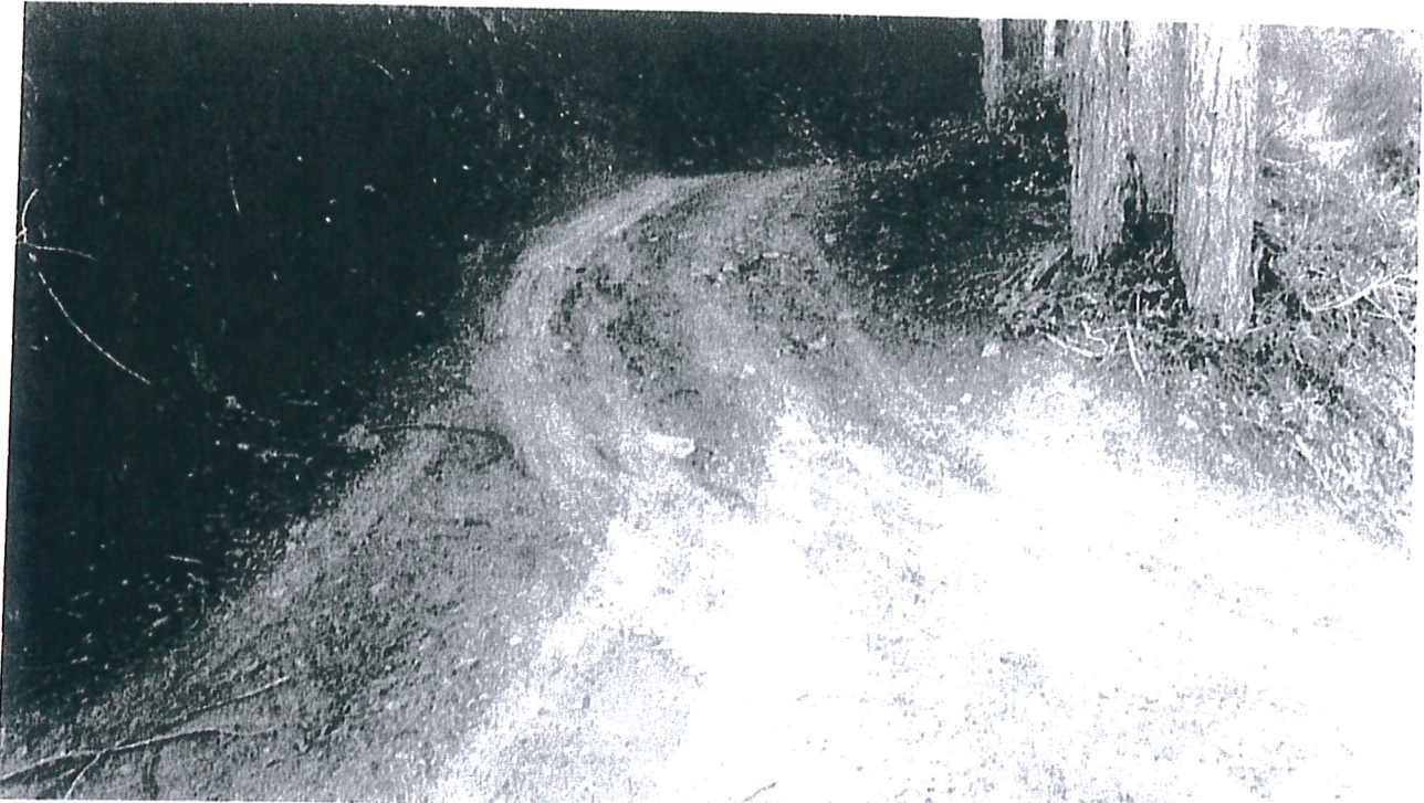
Road Point 4 looking at road surface erosion on the road up to Road Point 6. The Discharger shall rock armor the road up to Road Point 6.
