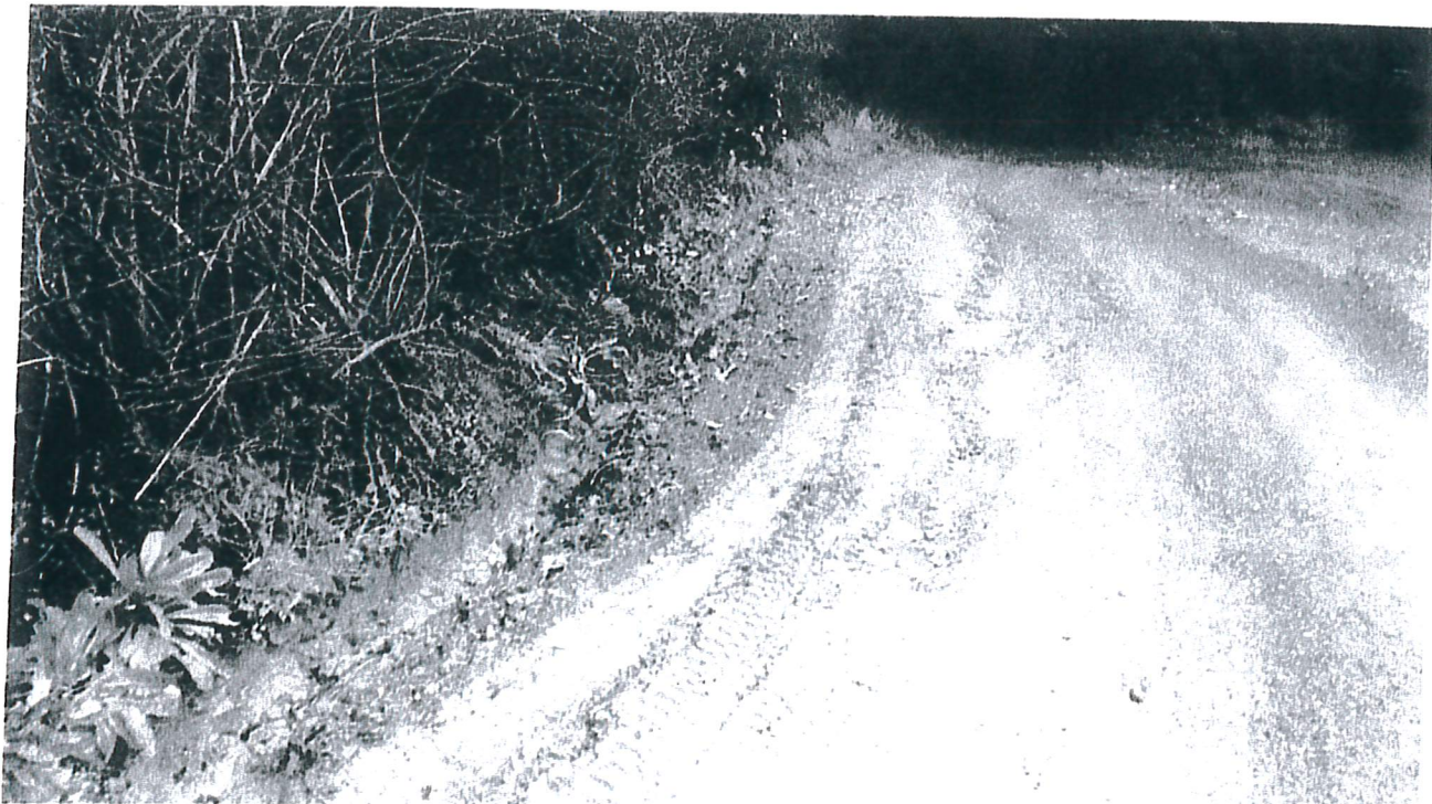
Road Point 3 towards Road Point 2: The Discharger has created a makeshift inside ditch as shown in the photo. The Discharger shall fully develop the inside ditch, rock the adjacent road and install waterbars across the road to divert surface flows into the inside ditch.
