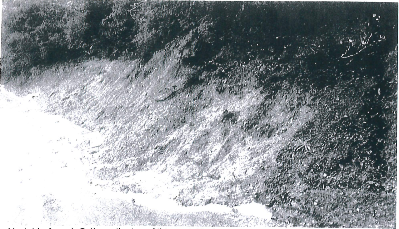
Unstable Area 1: Butress the toe of this unstable feature per attach specifications and install erosion control measures to help slow and prevent sediment delivery to drainages. Use straw bales or fiber logs in the drainage ditch below the unstable area and place straw bales or fiber logs around the base of the slumped bank. Picture taken 1/18/2017
