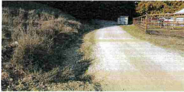
Figure 6: Road Segment C - 24" inboard ditch culvert inlet and current road surface.
