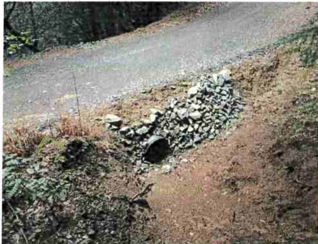
Figure 11: Current Conditions of 36" CPP inboard relief culvert
