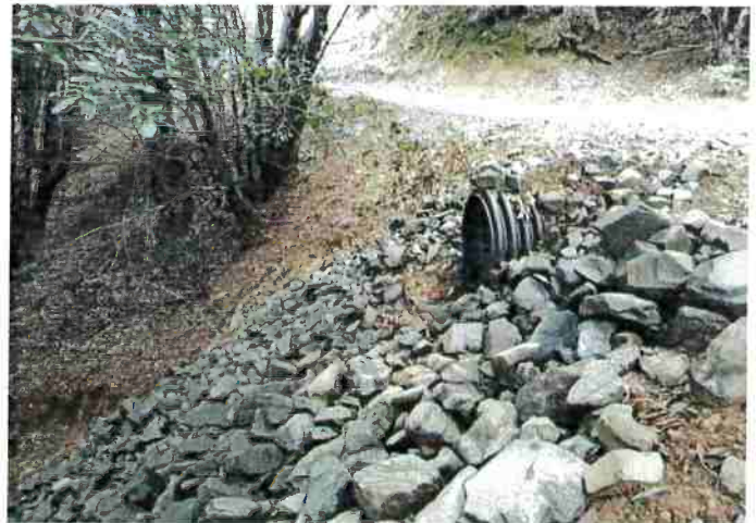
Figure 11: Current Conditions of 36" CPP inboard relief culvert
