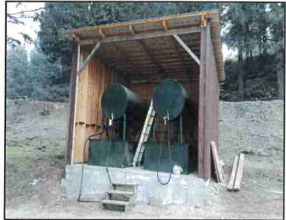
Figure 5: Fuel tanks with containment
