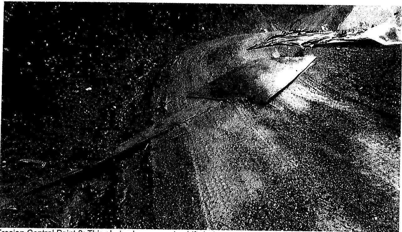
Erosion Control Point 3: This photo shows a makeshift drainage ditch crossing the road. The Discharger shall install a drainage ditch relief culvert where the boards are located that drain into the inside ditch on the left side of the photo. The Discharger shall also rock armor the inlet and outlets per attached photos.
