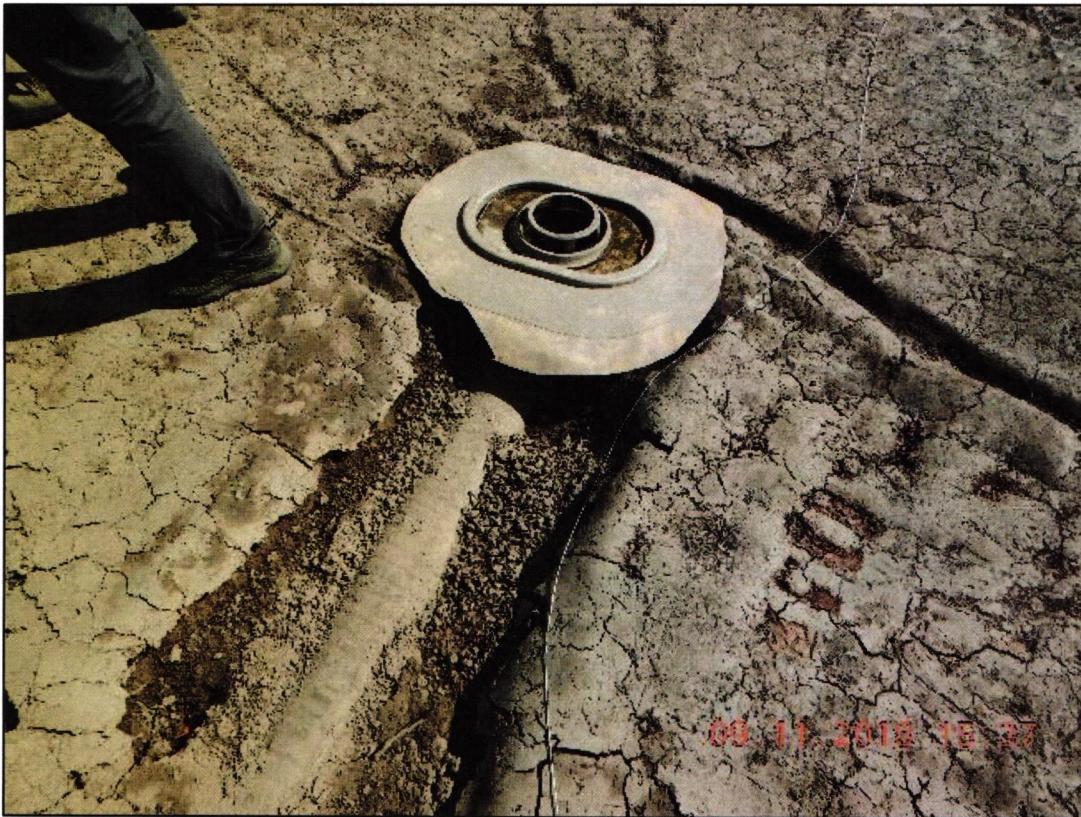
Photo 36: Bladder water receiver
