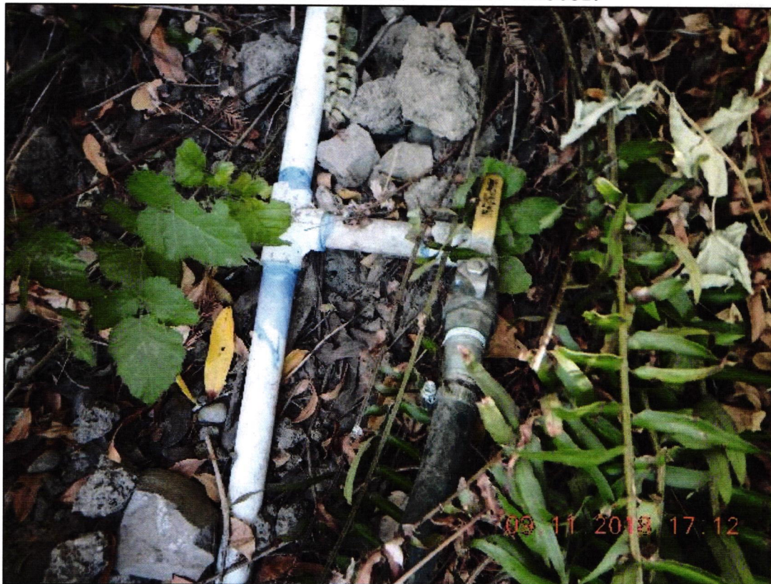
Photo 10: POD1 - Valve for Domestic or Catchment Area
