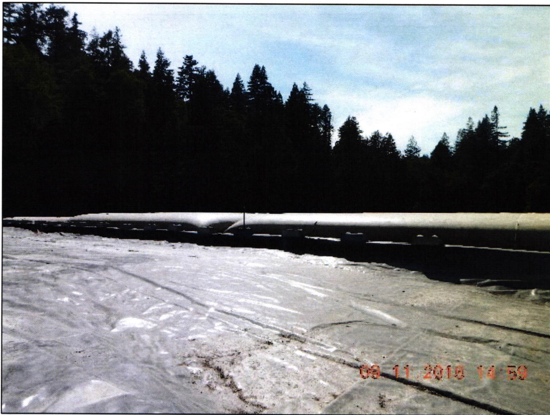
Photo 33: POS 1-14 - Bladders near collection area (210,000 gal. each)
