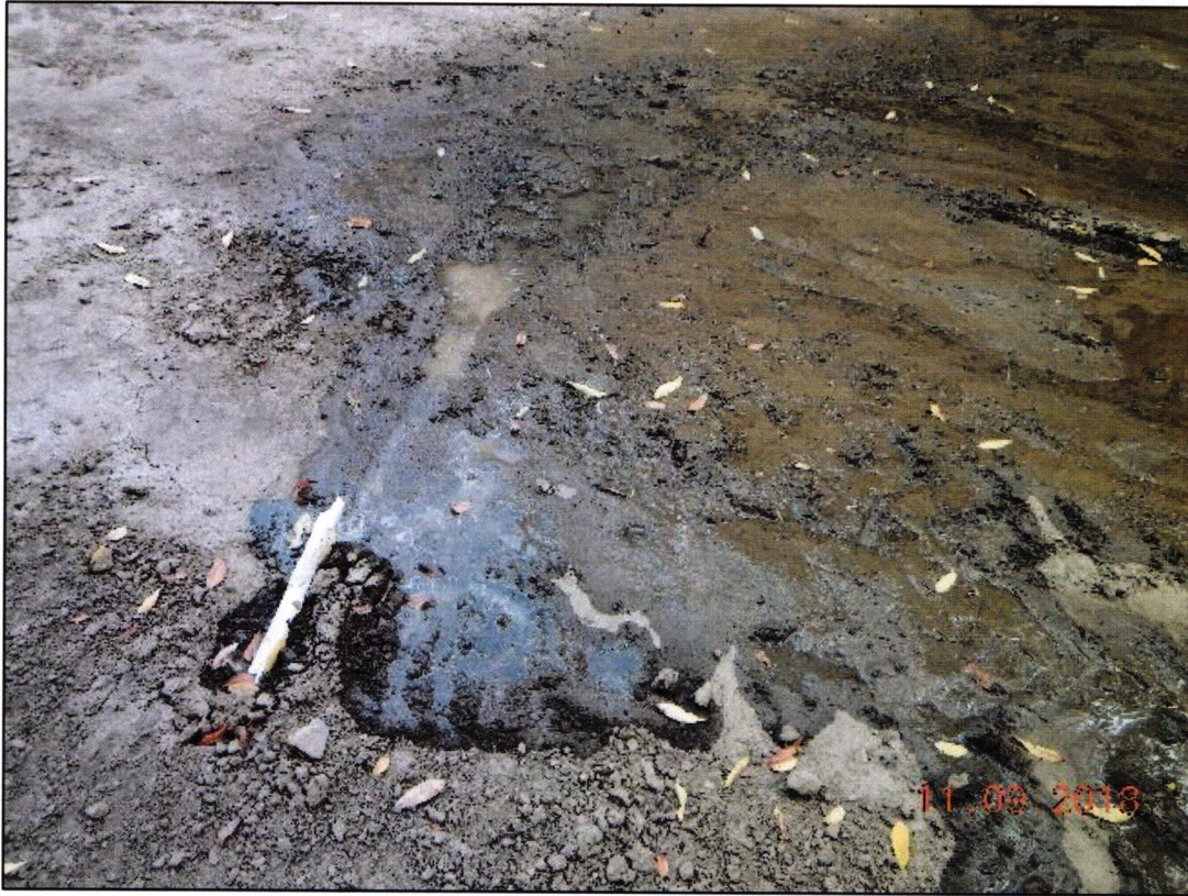
Photo 13: POD1 – Broken Pipe.
