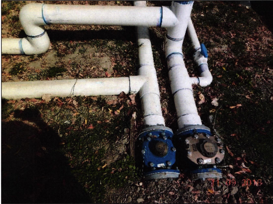
Photo 19: POD2 - Inlet pumps with meters.
