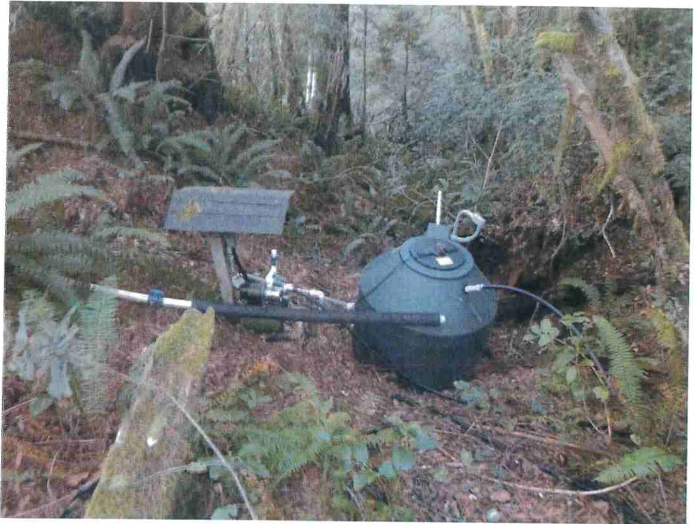
Picture 4: 300 gallon settling tank approximately 30' downhill from the POD. Photo date: 01/17/2018
