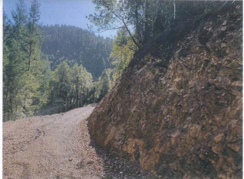
Picture 9 & 10. Rocky cut-bank demonstrating that the road was reconstructed from a "cut and fill" to "full-bench" road prism. This signficantly improves the stability of the road particularily given its proximity to a Class III watercourse. Photo date 2-1-2021
