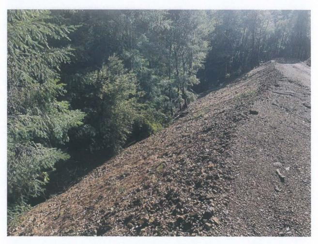
Picture 11. Reconstructed road's fill-slope proposed to be replanted. Photo date 2-1-2021
