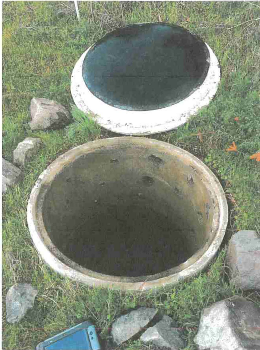
Picture 14: This is a photograph of the existing point of diversion (POD #1) located on a grassy hillside. The structure consists of a perforated 3' diameter by 4' deep concrete cistern. This structure diverts a combination of surface water and shallow ground water for domestic use. Photo date: 12/06/2016
