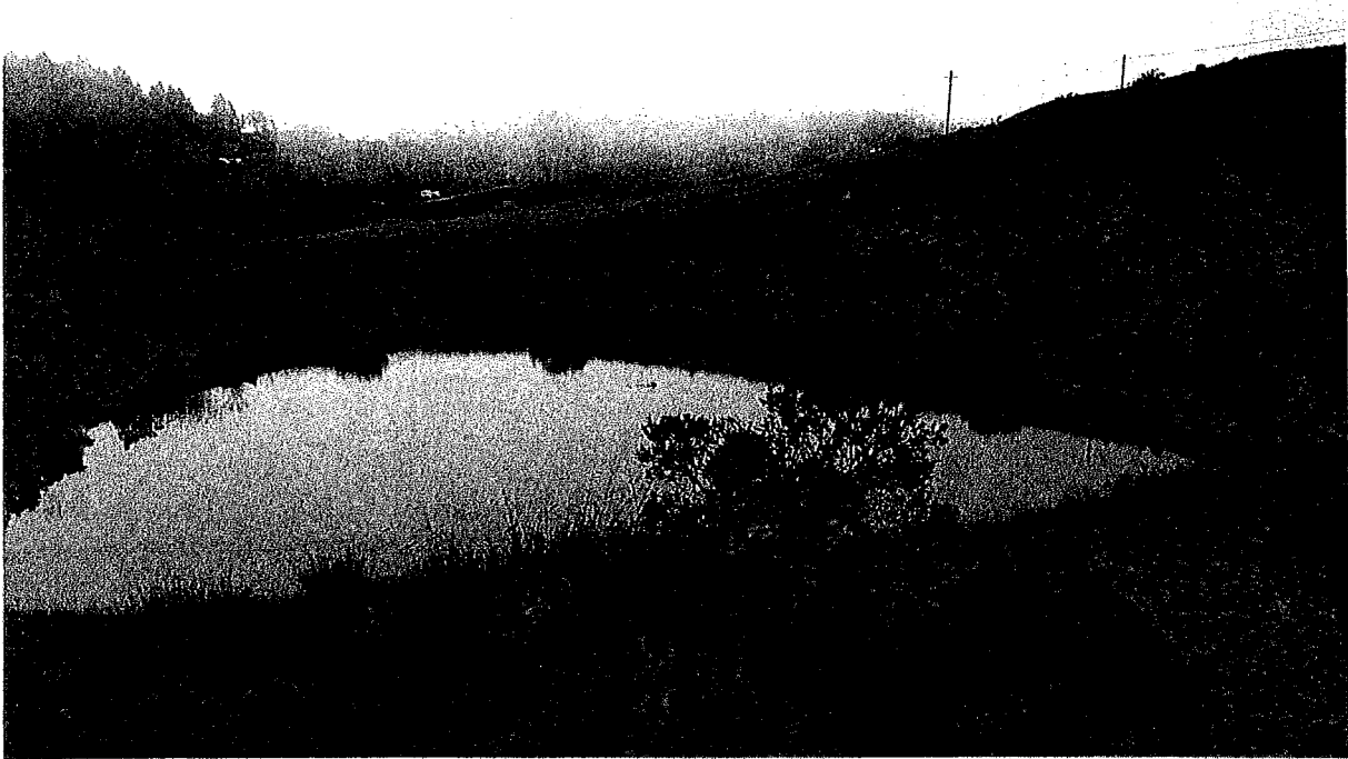
Picture 13: This is a photograph of the off-stream pond on the property, POD #2. This location is utilized as a source of irrigation water. The pond measures 222' long, 188' wide and 20' at its deepest point. The estimated pond volume is approximately 1.5 million gallons and the Discharger uses approximately 40% of the volume for irrigation. Photo date: 11/15/2016
