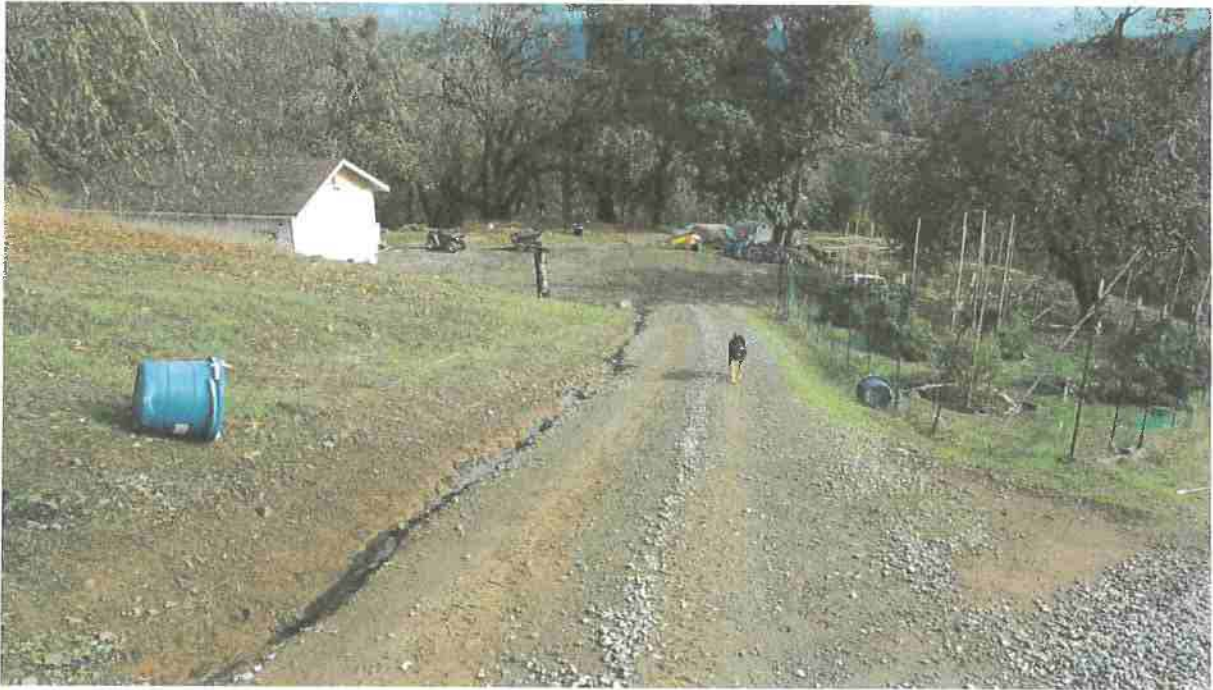
Picture 2: This is a photograph of the emergent groundwater eroding the seasonal road. This erosion does not deliver to a watercourse. The concentrated surface flow reaches the landing below and dissipates. This erosion will be mitigated by bypassing the emergent groundwater as mentioned in Picture 1. Photo date: 11/15/2016
