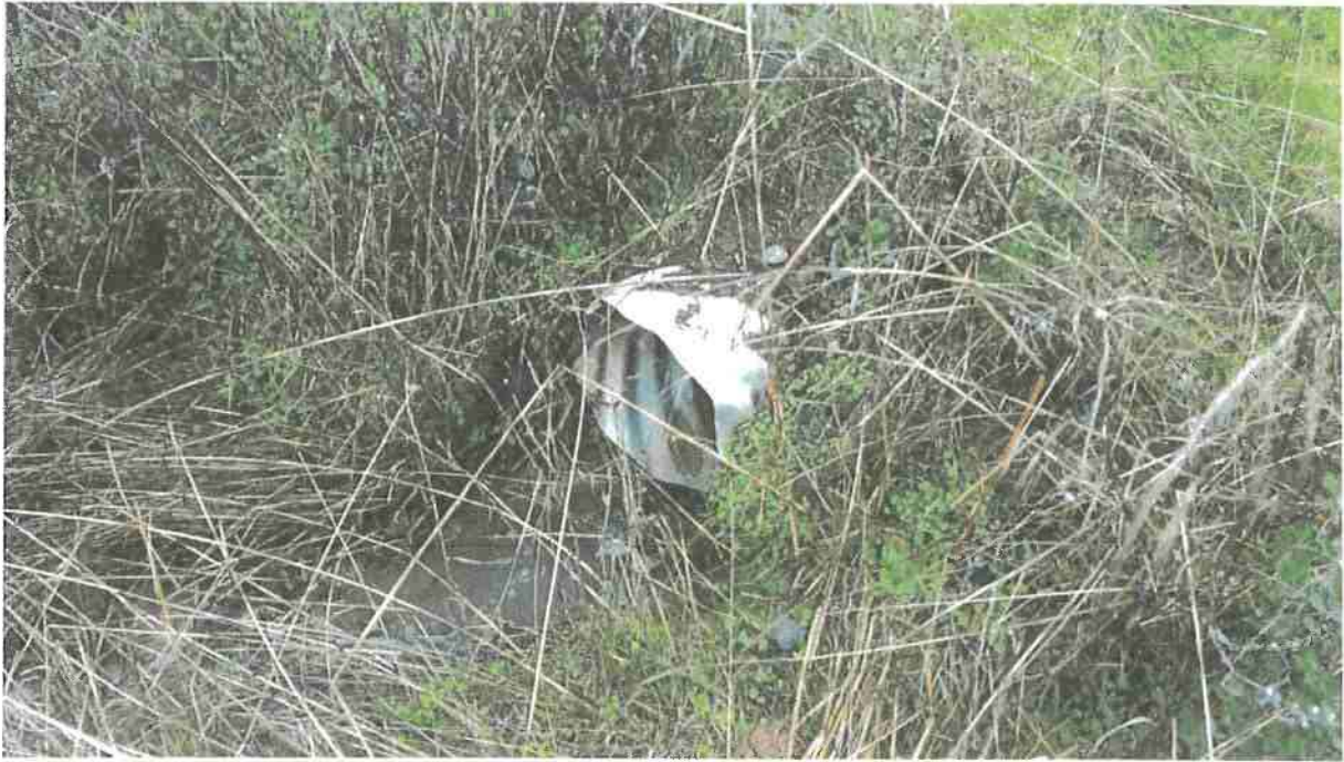
Picture 4: This is a photograph of the outlet of the existing 12" diameter CMP located at SC #1. The Discharger shall install a minimum 18" diameter culvert per specifications attached with this document. Photo date: 11/15/2016
