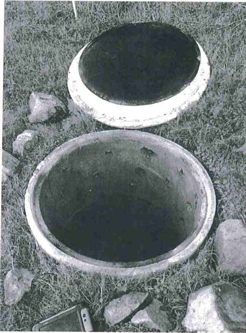
Picture 1: This is a photograph of the existing point of diversion (POD #1) located on a grassy hillside. The structure consists of a perforated 3' diameter by 4' deep concrete cistern. This structure diverts a combination of surface water and shallow ground water for domestic use. Photo date: 12/06/2016
