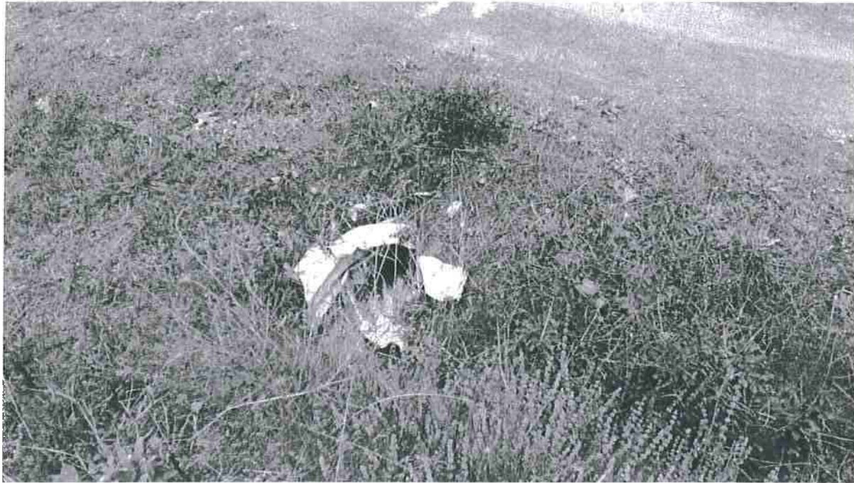
Picture 9: This is a photograph of the inlet to the existing 12" diameter CMP located at SC #1. This culvert facilitates the crossing of an unnamed Class III watercourse under a seasonal road. The applicant shall upgrade this location to a minimum 18" diameter culvert per specifications attached. Photo date: 11/15/2016
