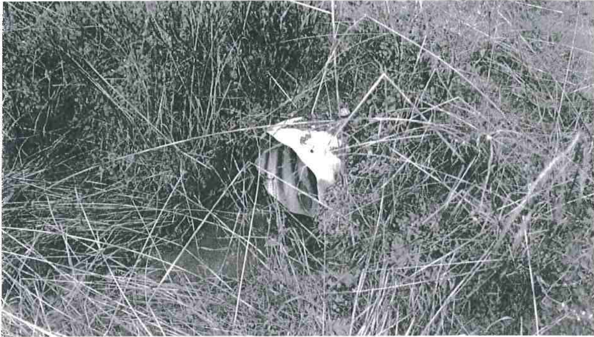
Picture 10: This is a photograph of the outlet of the existing 12" diameter CMP located at SC #1. The applicant shall install a minimum 18" diameter culvert per specifications attached with this document. Photo date: 11/15/2016
