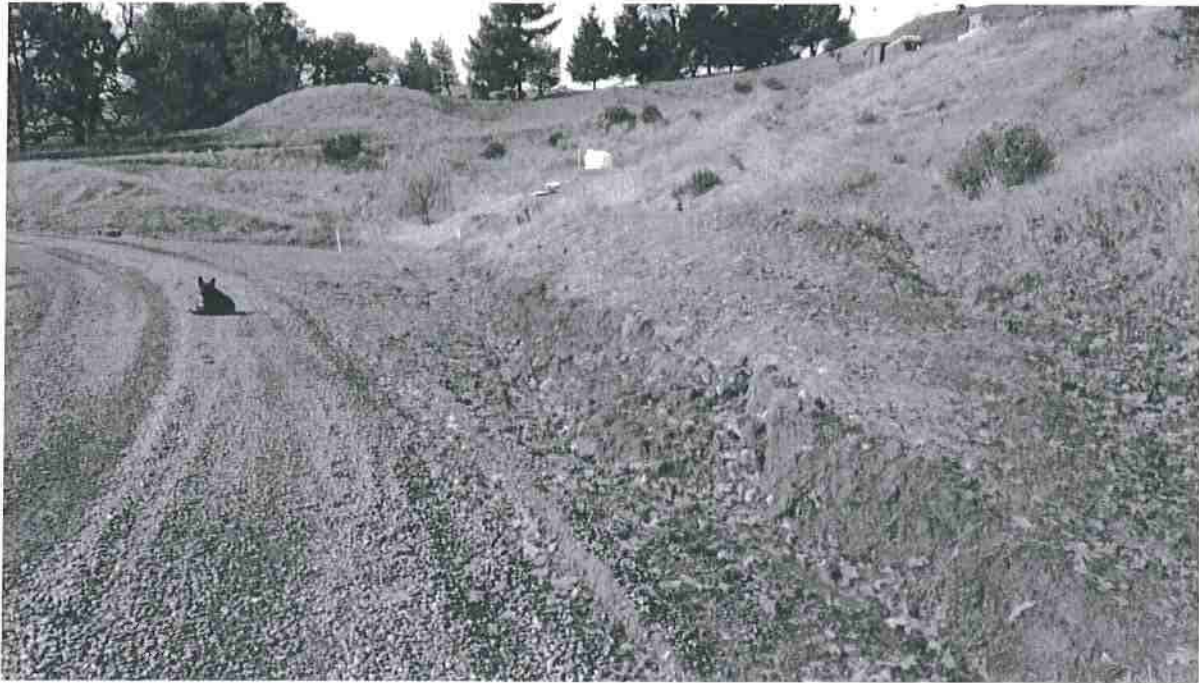
Picture 7: This is a photograph of the filled in pond site. The grassy flat in the left of the photo is where the pond once was. The white pole on the flat marks the point where groundwater reaches the surface. At the inboard edge of the road is surface runoff from the emergent groundwater. The applicant would like to collect and bypass this emergent groundwater so it safely reaches the head of a Class III watercourse 200' to the south. Photo date: 11/15/2016
