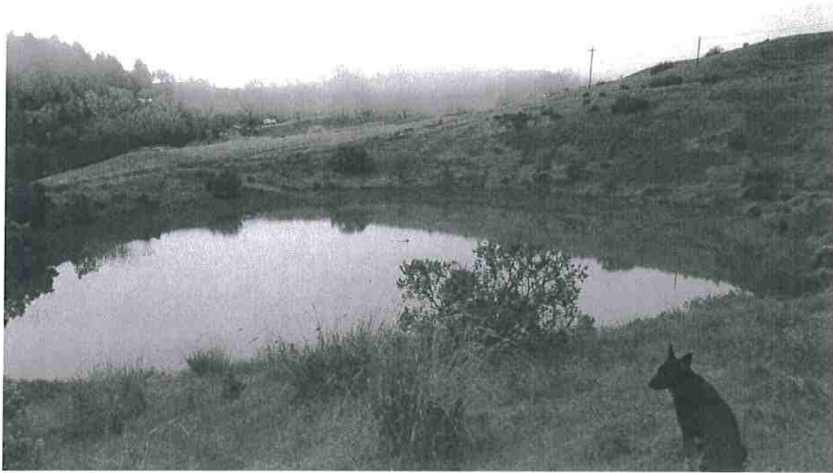
Picture 4: This is a photograph of the off-stream pond on the property, POD #2. This location is utilized as a source of irrigation water. The pond measures 222' long, 188' wide and 20' at its deepest point. The estimated pond volume is approximately 2.5 million gallons and the applicant uses approximately 40% of the volume for irrigation. Photo date: 11/15/2016
