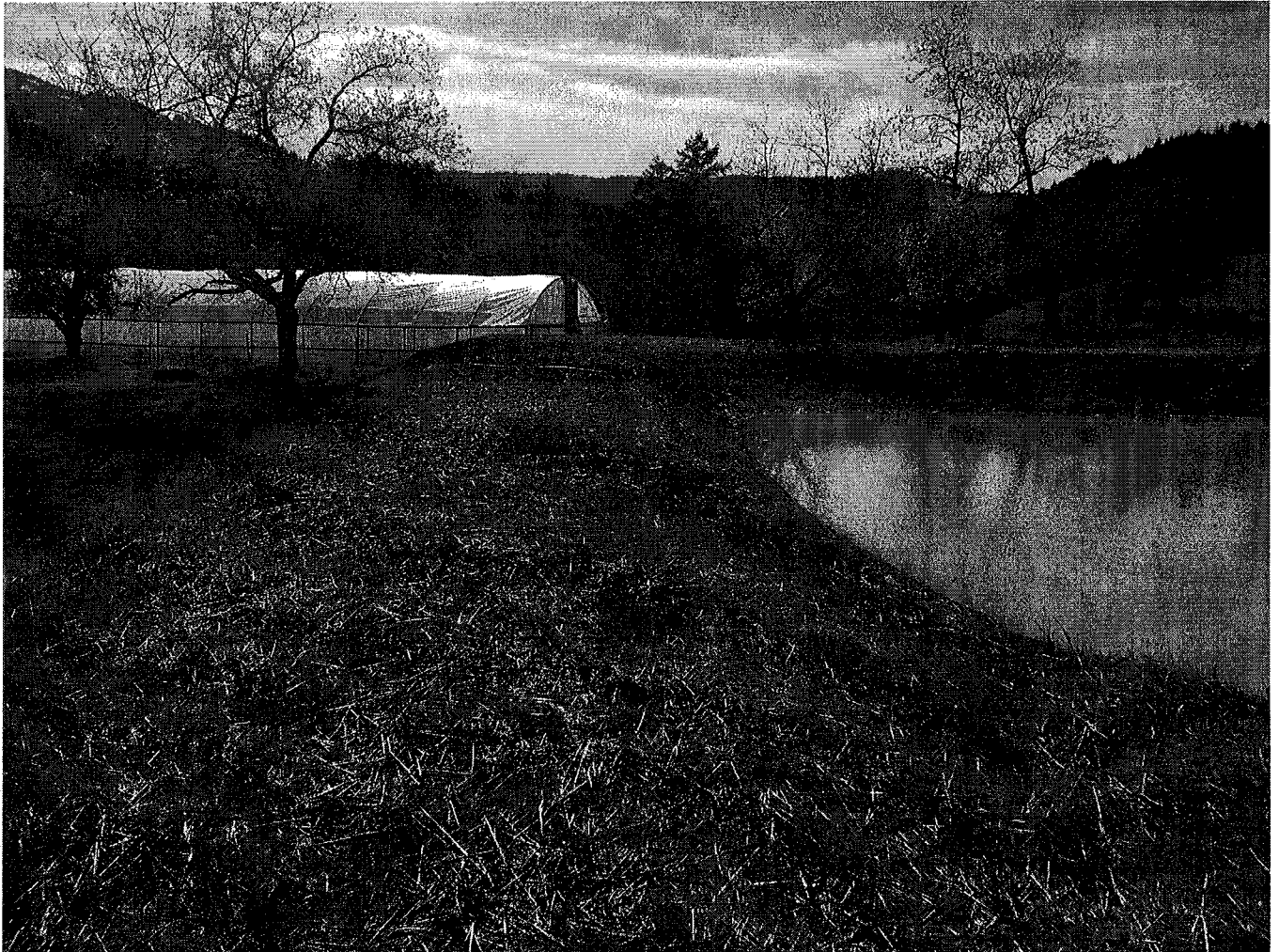
Picture 9: Pond embankment and crest facing west. The width of the crest at freeboard height is approximately 10-12 feet. The Photo date 4-9-2016.
