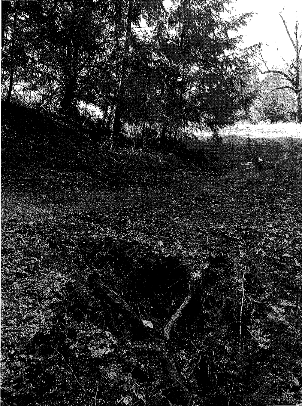
Picture 12: Photo of outlet of Class III dirt ford crossing on secondary access road. This crossing is presently head cutting. The pond could contribute surface flow to this crossing and therefore the crossing needs to be upgraded to a Rock Ford. Photo date 4-9-2016.
