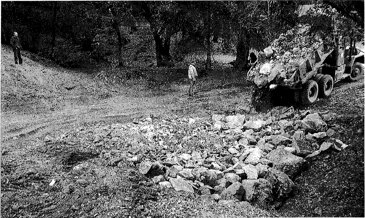
Picture 2 of 4: Well graded rock armor is then backfilled into the structure and spread across the breadth of the U-shaped stream crossing, and about one-third the way up the roadbed, so that streamflow will only flow over or come in contact with resistant armor material. The armor must be spread and compacted across the design width of the expected flood flow channel width so peak flows will not flank the armored structure.
