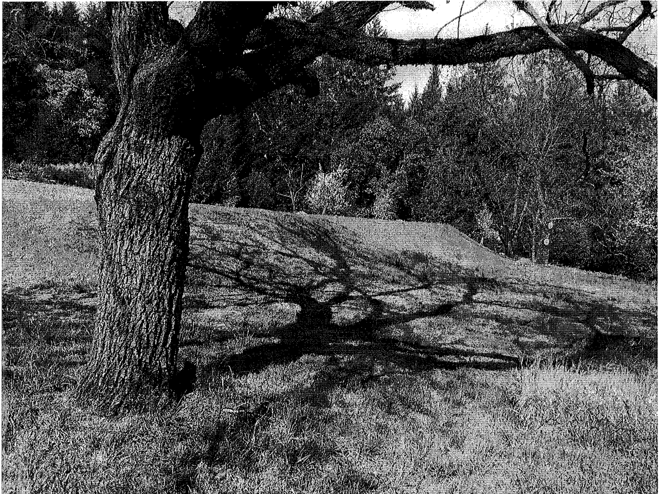
Picture 10: Photo of pond's southern outer embankment face, which is approximately 2.5:1~2:1 slope steepness. Photo facing east. Photo date 4-9-2016.
