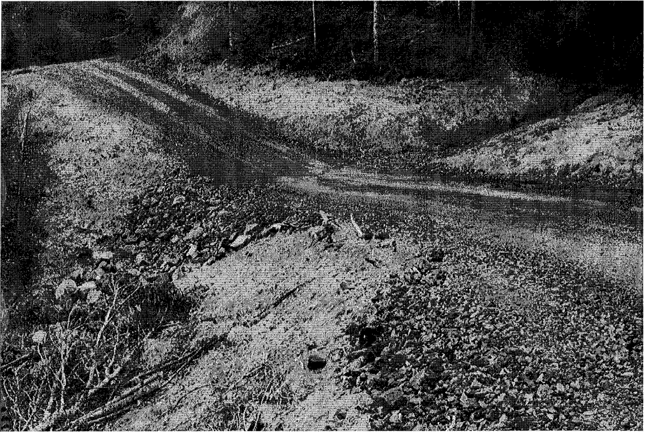
Example of a well-constructed rock ford with armored fill
