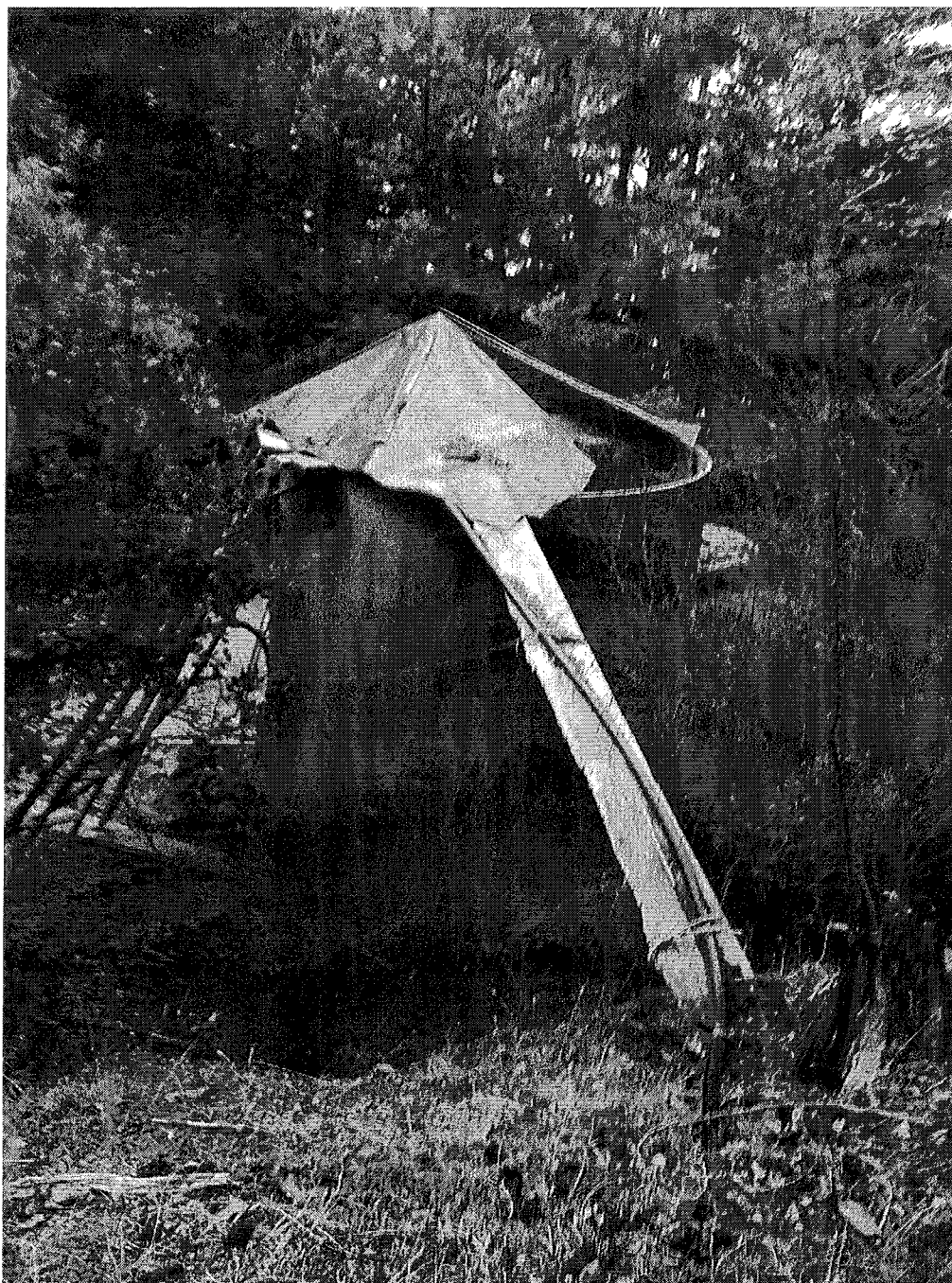
Picture 3: This is a photo of the 2,000-gallon water tank located approximately 200 feet west of the POD. Water diverted from the spring is piped to this storage tank for pumping upslope to the 25,000 gallon holding tank. Photo date 4-9-2016.
