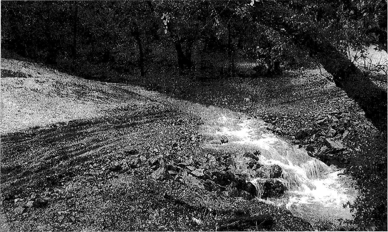
Picture 3 of 4: Two weeks after this armored fill was constructed, a storm flow event occurred and the structure maintained its function and integrity. The road approaches had not yet been compacted or surfaced with road rock
