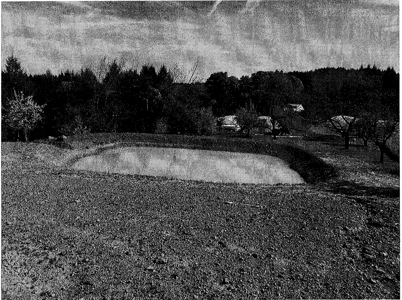
Picture 5: Off-stream pond looking southeast. The pond was constructed between 1998 and 2005. In 2014, the pond was grown over with small trees and shrubs and only holding approximately 10-15% of its capacity. In hopes of increasing/improving water holding capacity, the applicant enlarged the pond and compacted the impoundment structure and embankment face followed by slope stabilization. In 2016, the pond filled entirely from rain water and just barely overtopped into the spillway, which is located at left of photo near apple tree. Photo Date 4-9-2016.
