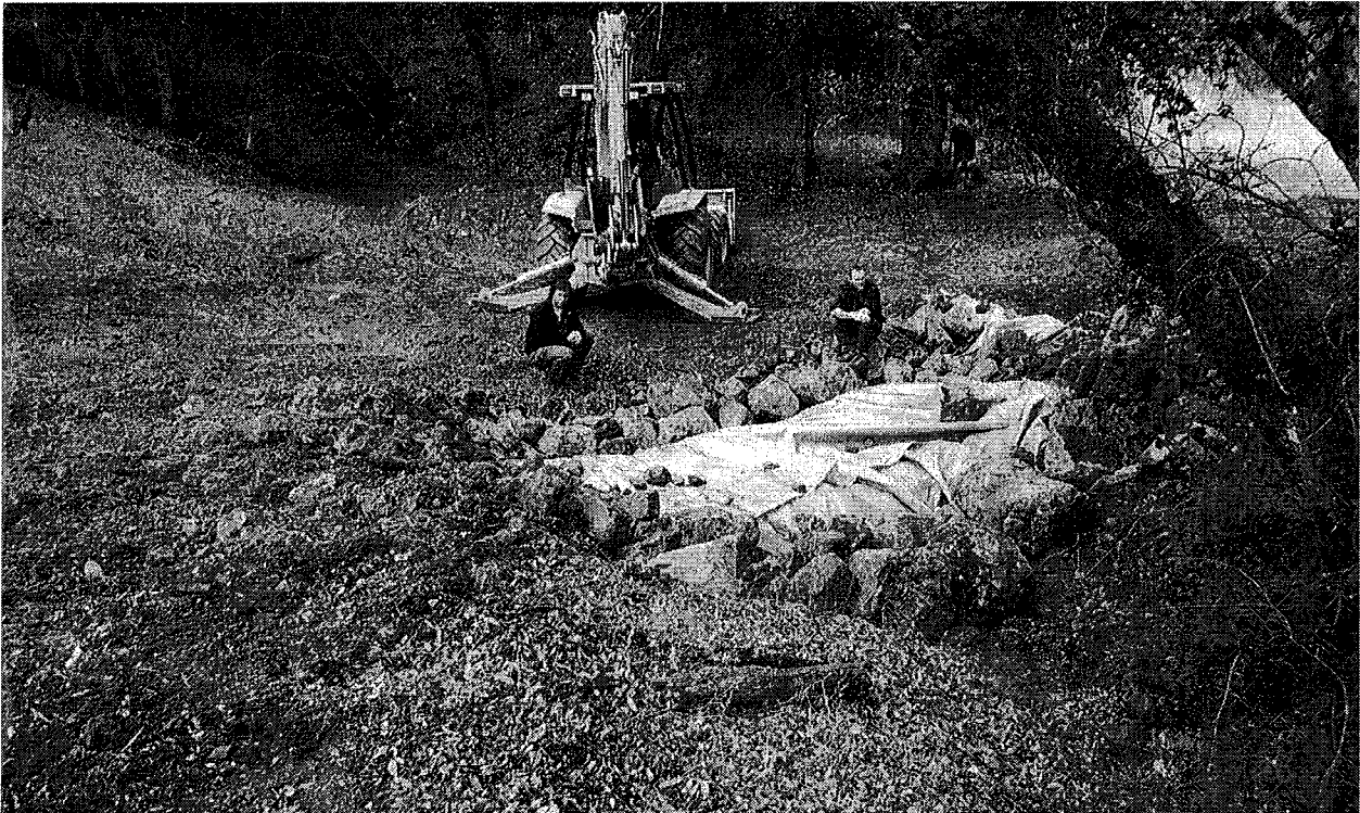
Picture 1 of 4: An excavator or backhoe is used to dig a broad keyway across the base of the fill, where the fill intersects the natural channel, and another broad keyway at the top of the fill, where the top edge of the road surface is planned. The largest rock goes in the lower keyway, and coarse armor is also placed in the upper keyway across the full width of the design spillway where streamflow will flow over the fill and down the armored fill slope. Filter fabric, or a filter layer of small rock, is placed on the underlying soil to prevent erosion or winnowing of soil beneath the armor.
