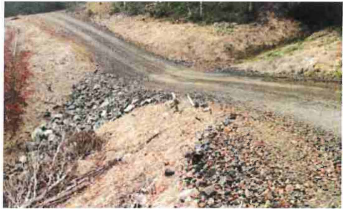
FIGURE 120. This armored fill crossing of a steep, ephemeral stream was constructed to provide a low maintenance crossing. The crossing has been deeply dipped to reduce the volume of road fill and to eliminate the potential for stream diversion. The fill slope has been heavily armored through the axis of the crossing to contain flood flows and prevent down-cutting. Armored fills cannot be used on fish bearing streams.
