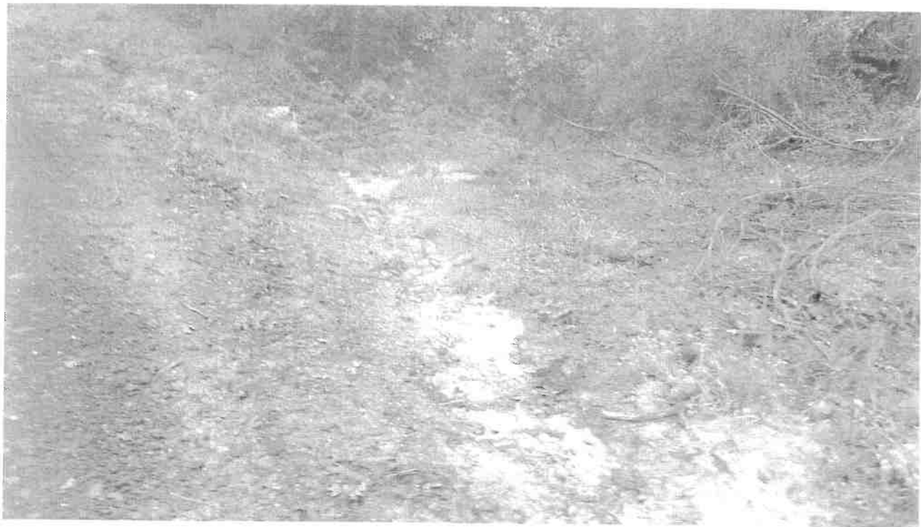
Site 08 – Top photo: Looking East up the inside ditch to Site 10. Sediment fines are present in the inside ditch. Bottom photo: Looking West from Site 08 with the watercourse crossing culvert inlet at Site 07 visible in the background with sediment fines in the inside ditch leading into the inlet of the watercourse crossing.
