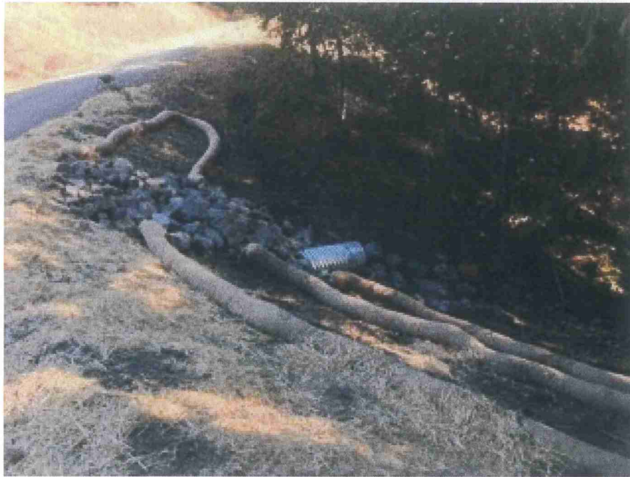
Picture 4: Crossing #1's outlet in the process of Erosion Control being applied. (photo was provided by the Applicant on 11-12-2020.
