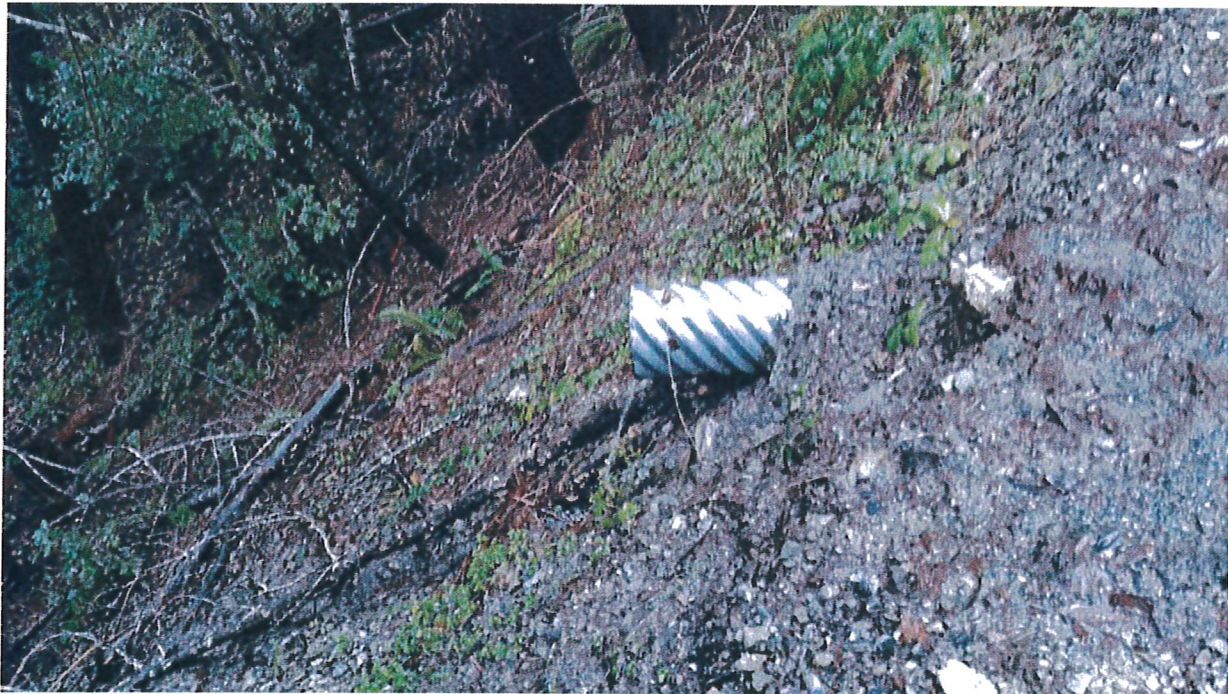
Ditch Relief Culvert 1: Plugged 12" diameter inside ditch relief culvert that has a plugged inlet and no rock armoring of the outlet. The Discharger shall unplug the entire culvert or replace it with an 18" diameter culvert and rock armor the outlet per attached specifications.
