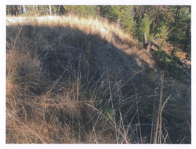
Picture 4: Perched fill located along Cultivation Site 2's eastern periphery, which shall be pulled back to a minimum 2:1 slope steepness. Photo date 10-14-2020.
