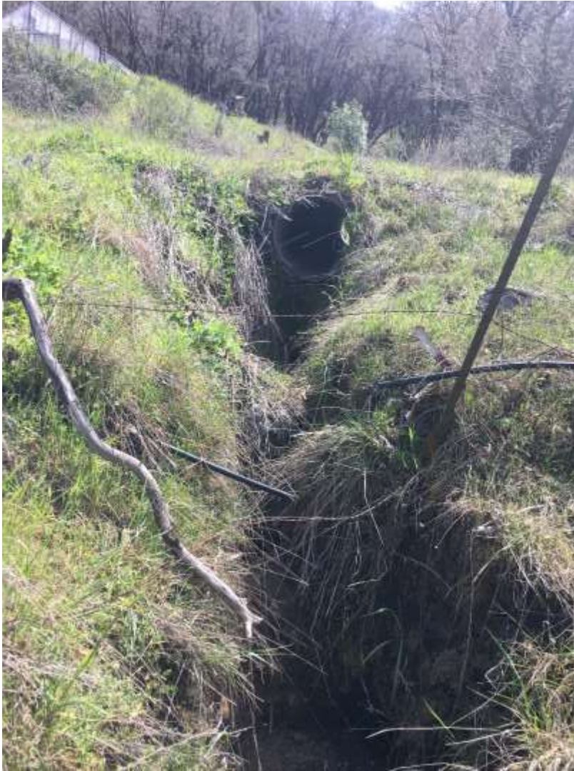
Photo 11. Downstream of Class III culvert with some erosion issues
