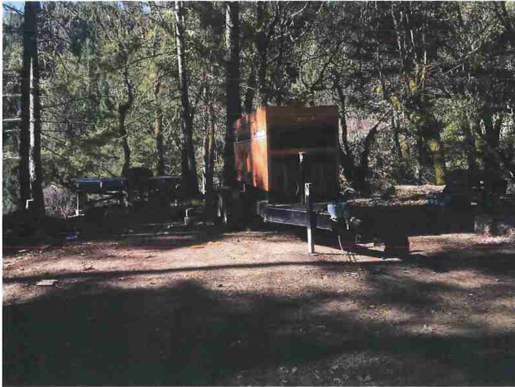
Figure 9: RP12: Generator needing fuel containment structure.
