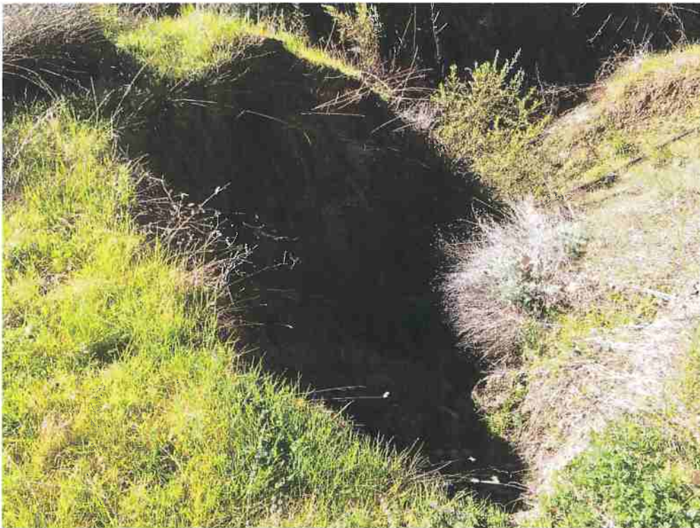
Figure 10: RP13: Existing eroded crossing. Remove fill and install a rocked ford.
