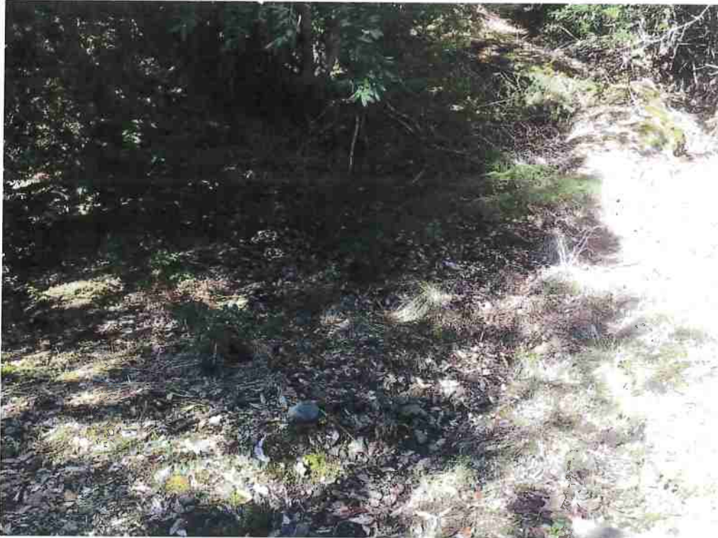
Figure 11: RP 14. Existing eroded crossing. Remove fill and install a rocked ford.
