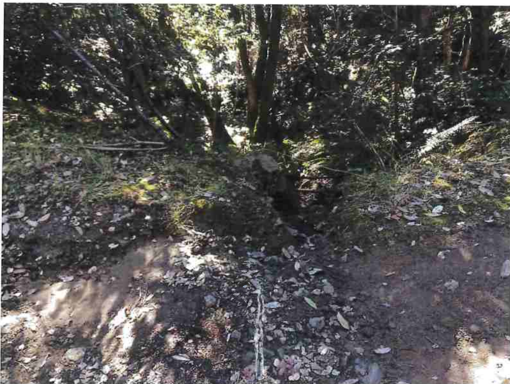
Figure 12: RP15. Existing eroded crossing. Remove fill and install a rocked ford.
