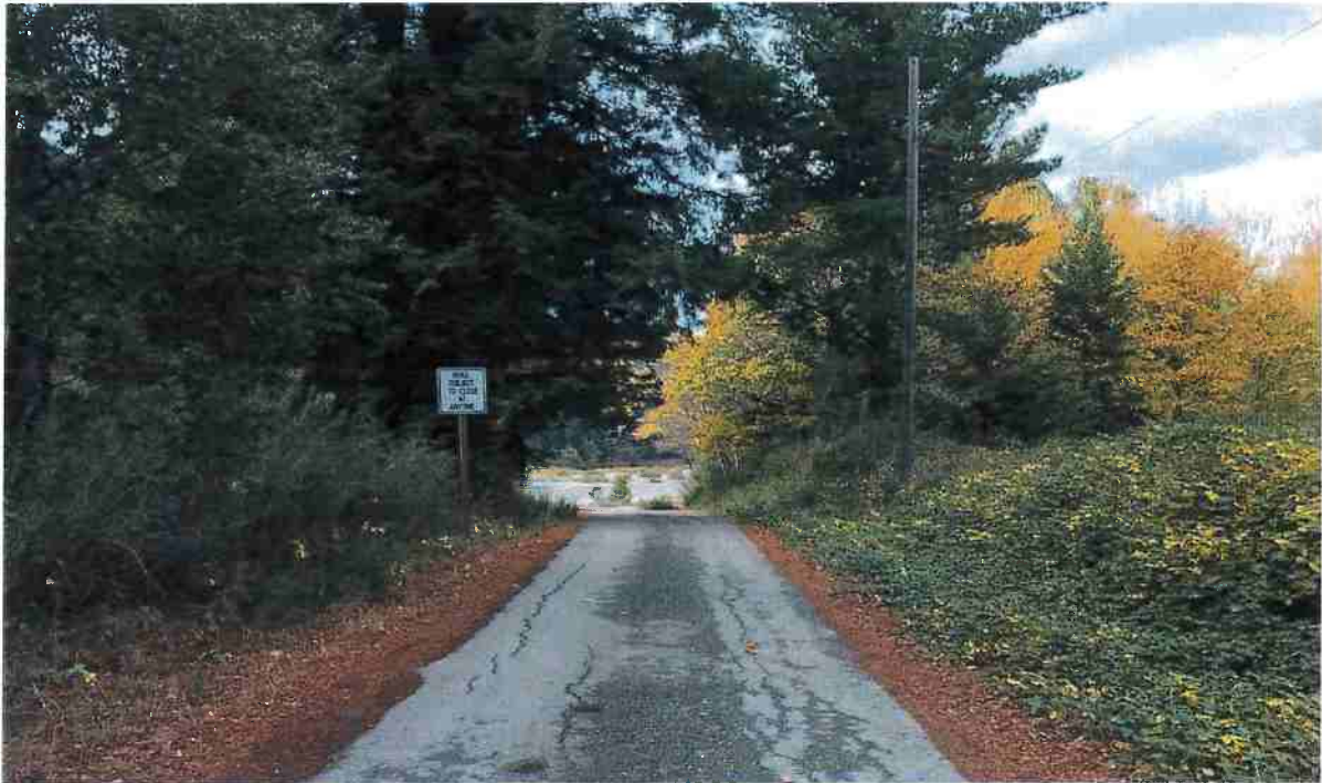
Photo No. 6. Failing asphalt travel way approximately 14'-wide. The sign reads, "Road Subject to Closure at Any Time." No inter-visible turnouts.
