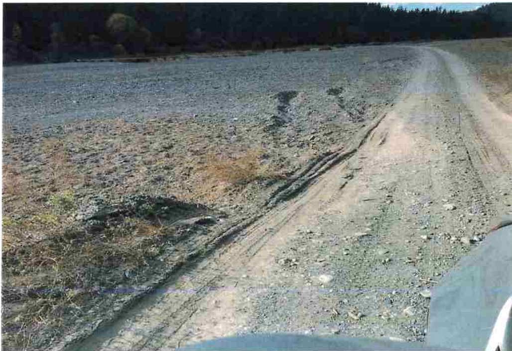
Photo No. 2. 14'-wide travel way across floodplain/gravel bar, unconsolidated shoulders. Tracks are evidence of vehicles getting stuck in the gravel off the travel way.
