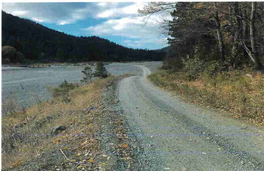
Photo No. 5. Looking back down to the floodplain/gravel bar, travel way is 12', inadequate shoulder, gravel surface.
