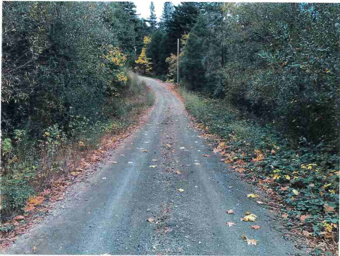
Photo No. 9. 12'-wide travel way, no shoulder, gravel/dirt surface, no inter-visible turn outs.
