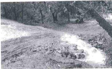
FIGURE 121E. Two weeks after this amound fill was constructed, a storm flow event occurred and the structure maintained its function and integrity. The road approaches had not yet been compacted of surfaced with road rock.
