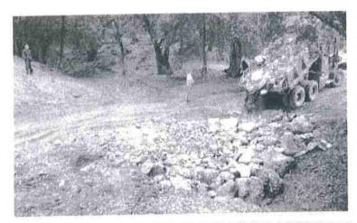
FIGURE 121D. Well graded took armor is then buckfilled into the structure and spread across the breadth of the U-shaped stream crossing, and about one-mind the way up the readbed, so that streamflow will only flow over or come in contact with resistant armor material. The armor must be spread and compacted across the design width of the expected flood flow channel width so peak flows will not flank the armored structure.
