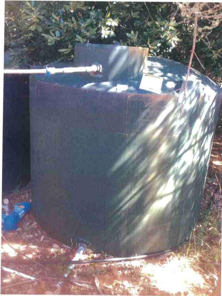
Photo 2: One 3,000 gallon poly water storage tank. Photo date 8-15-16
