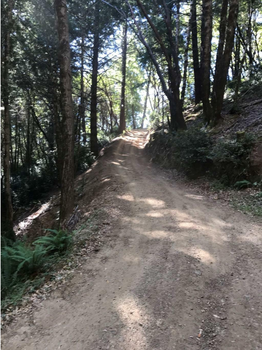
Photo 3. View from Observation Point 2(a) looking south up steep grade where water bar should be installed.
