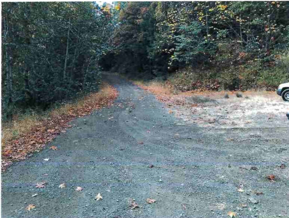
Photo No. 14. Looking west from the gate. 15'-wide travel way, no shoulder, gravel surface.
