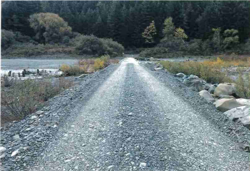
Photo No. 1. 11'-wide, one-lane, low water bridge and approach, no shoulder, gravel surface.
