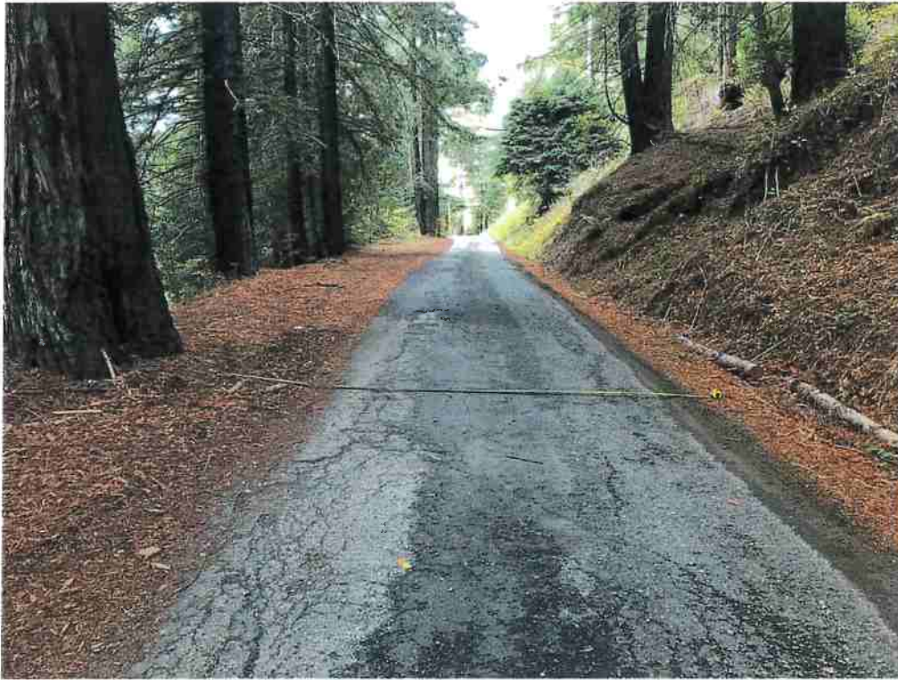
Photo No. 7. 13-wide travel way, degraded asphalt surface, with inter-visible turn outs.
