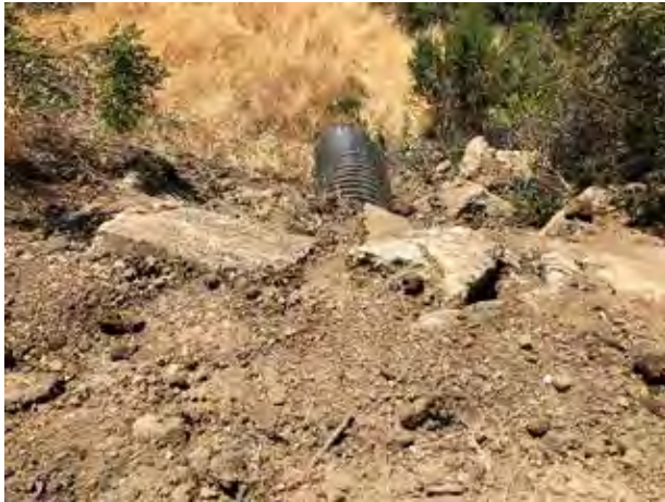
Photo #179 Red Rock Rd Looking @ 18" Culvert Out
