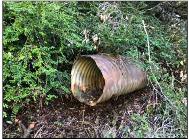
Photo #14 Fish Canyon Rd Damage Old 30" Culvert To Be Disposed Of.
