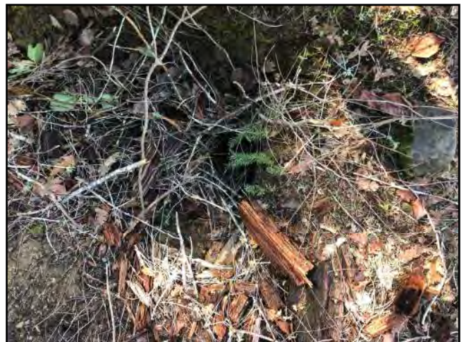
Photo #36 Fish Canyon Rd Clogged 18" Culvert In
