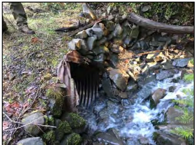
Photo #12 Fish Canyon Rd Damage 36" Culvert In
