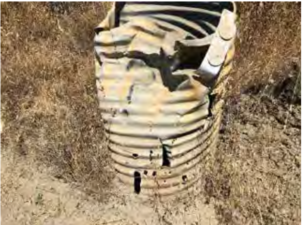
Photo #216 Red Rock Rd Looking @ 18" Culvert Inlet
