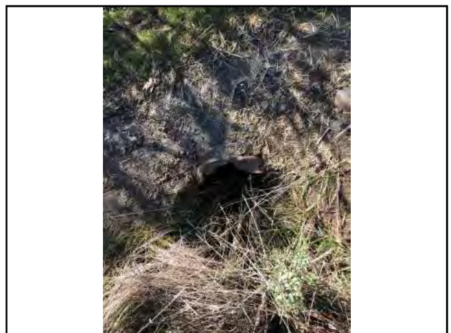
Photo #72 Road H @ Driveway Partially Clogged and Rusty 12" Culvert In
