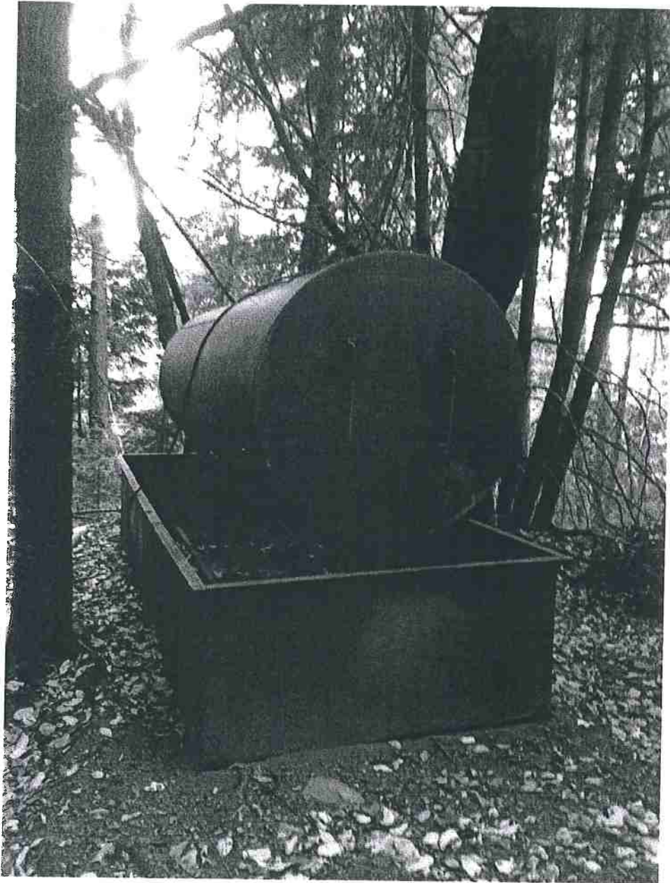
Photo 20: Diesel storage tank with secondary containment. Photo date 8-29-16
