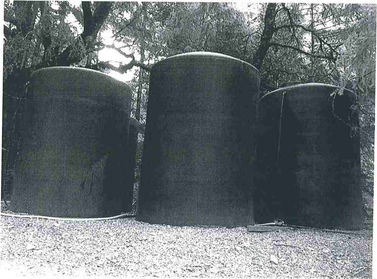
Photo 13: Five 5,000 gallon poly water tanks, one obstructed from this view. Photo date 8-29-16
