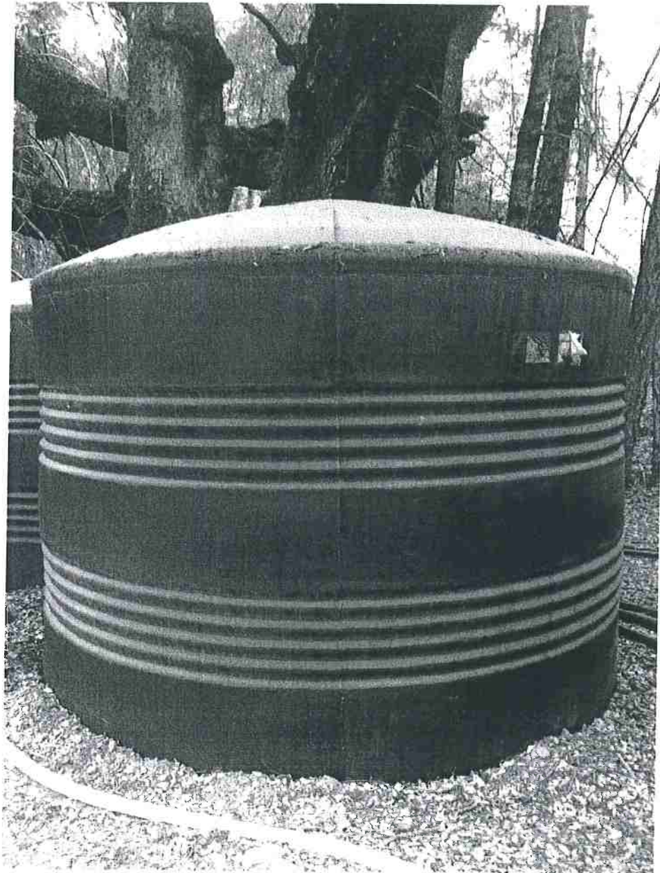
Photo 15: Two 2,500 gallon poly water tanks. Photo date 8-29-16
