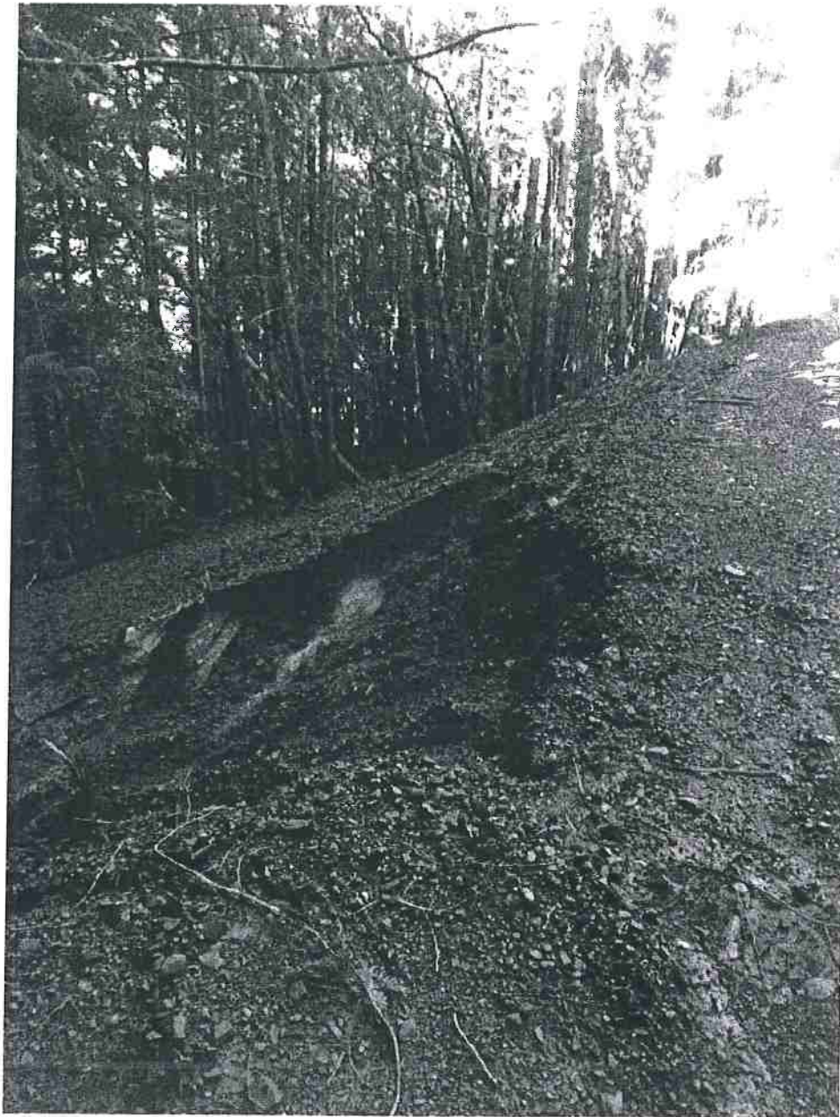
Photo 17: Erosion on fill slope of pond #1. Photo date 1-24-17
