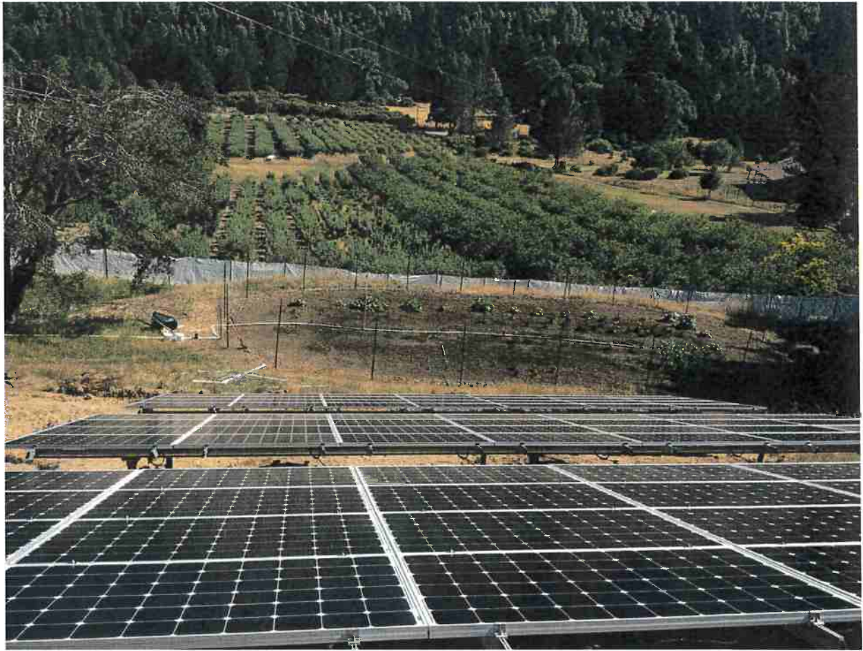
Whitethorn, CA: A 20 kW ground mount grid-tied system powering the home and operations of a local Quince farm.
