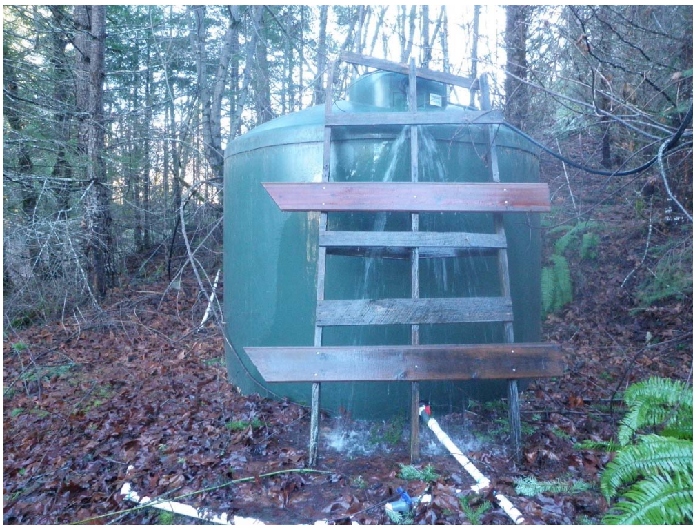
Photo 26 – View of leaking 3,000 gal water tank (Photo December 2018).
