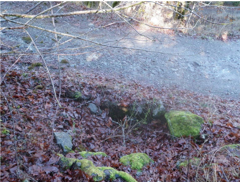
Photo 12 – View of 18-inch diameter culvert inlet at SC #4 (Photo December 2018).
