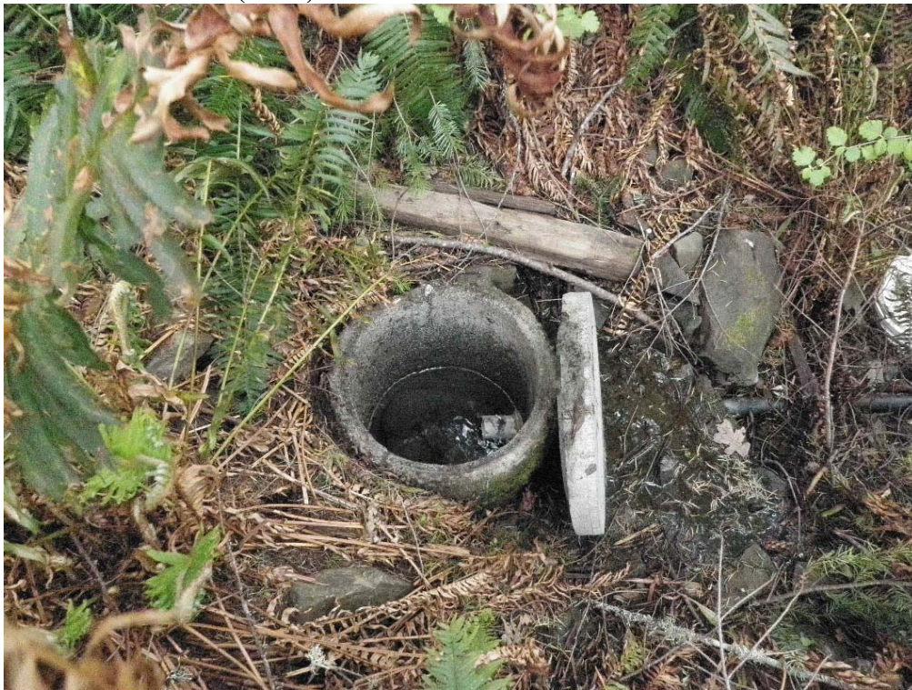
Photo 1- POD- view of concrete cistern located on a Class II stream. The diversion structure is embedded in the stream channel (Photo April 2016).
