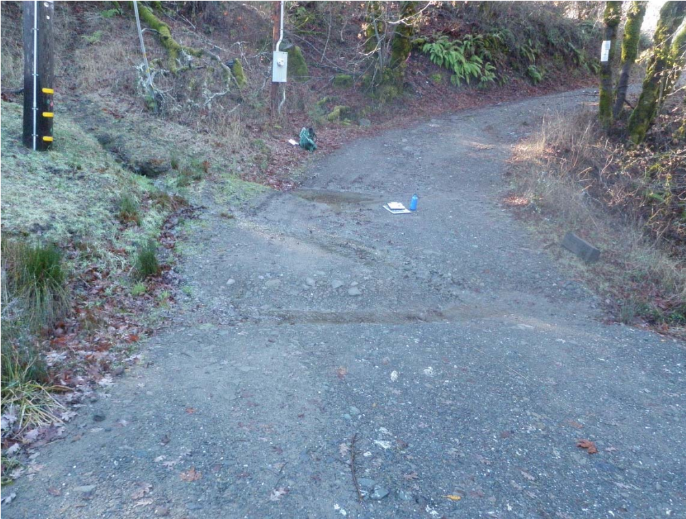
Photo 11 – View of SC #4 looking perpendicular to the road. There are two small Class II watercourses which confluence at the road each conveyed across the road by different means (18-inch dia. culvert and no drainage structure) (Photo December 2018).
