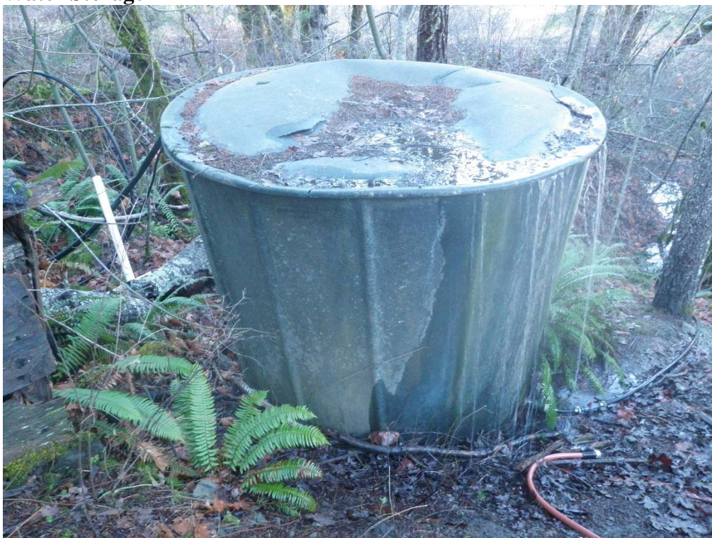
Photo 22 – View of leaking 1,000 gallon water tank downstream of POD (Photo December 2018).
