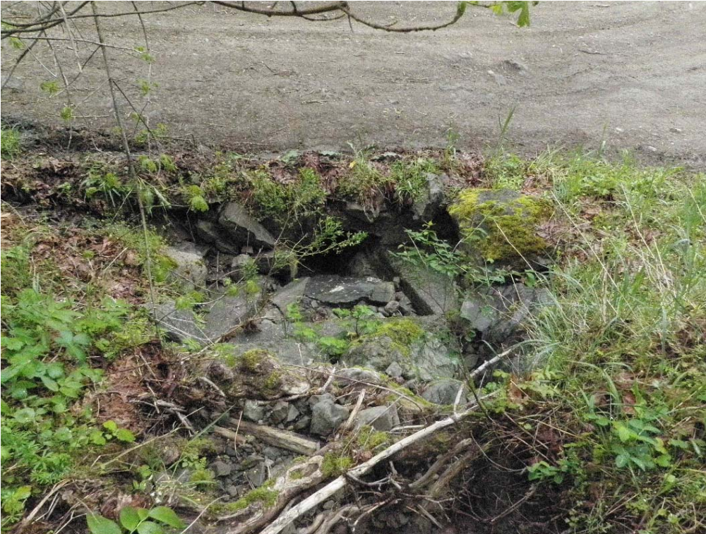
Photo 9 – View of SC #3 looking downstream at 30-inch diameter culvert inlet on Class II watercourse. The culvert inlet is slightly obscured by poorly place rock armor (Photo April 2016).
