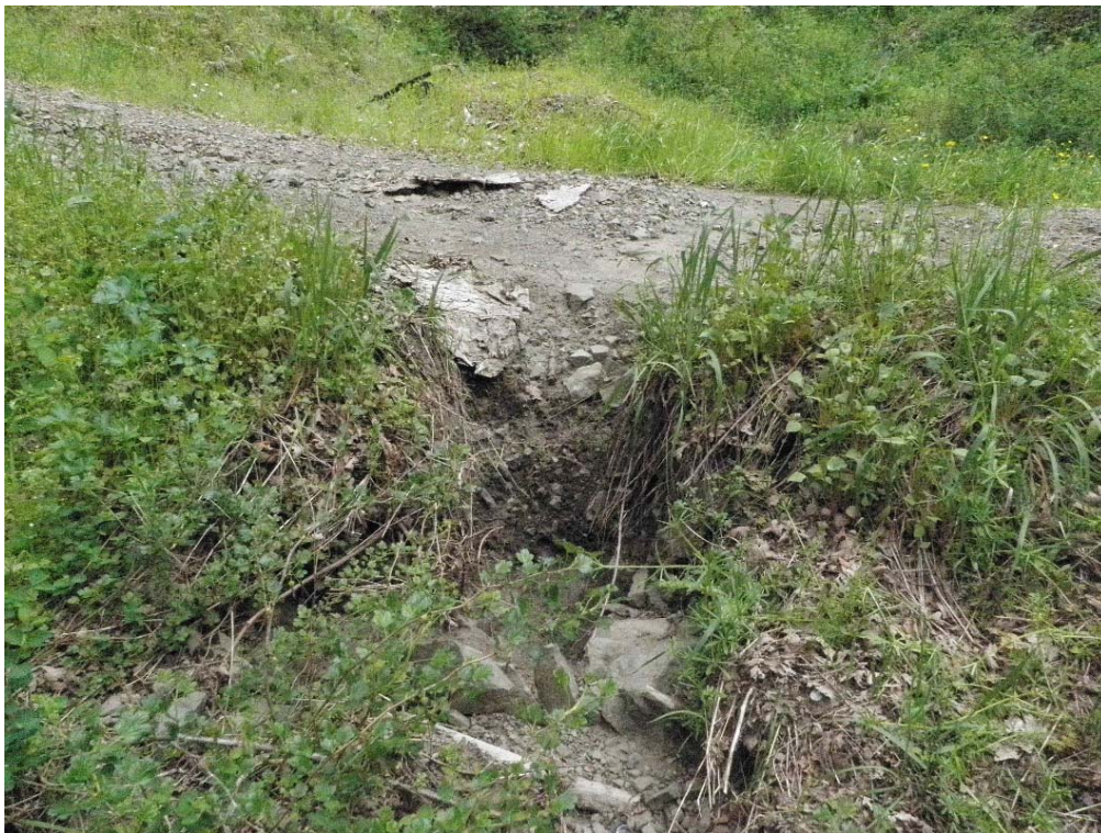
Photo 5 – View of SC #1- looking upstream at a headcut forming in the outboard road on Class III watercourse (Photo April 2016).
