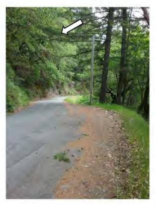
BMR MP 1.2, 15-ft wide asphalt surface with a longitudinal slope of 7%, and 3-ft. wide and 30-ft. long pullout allows for sight distance at utility pole at mile 1.17. Note white arrow showing location of utility pole (Photo 11).
