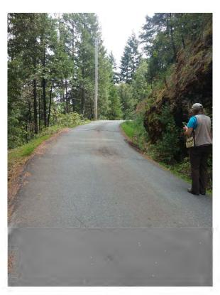
BMR PM 3.63, 18-ft. wide asphalt surface with a longitudinal slope of 11%, narrows to 11-ft. wide with no shoulder at a rock outcropping on the cutbank and proceeds for 250 feet at15-ft. wide. Visibility is limited to 120 ft. around the curve (Photo 26). Road resumes 18-ft. width past the curve.
