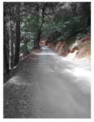
BMR PM 4.7 to PM 4.8, 13-ft. wide gravel surface with a longitudinal slope of 7% at end of asphalt surface. Trees limit visibility (Photo 28).
