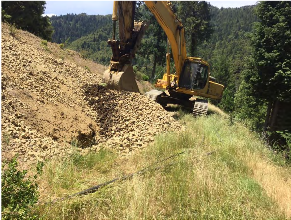
Photo 1: Excavating dry well
