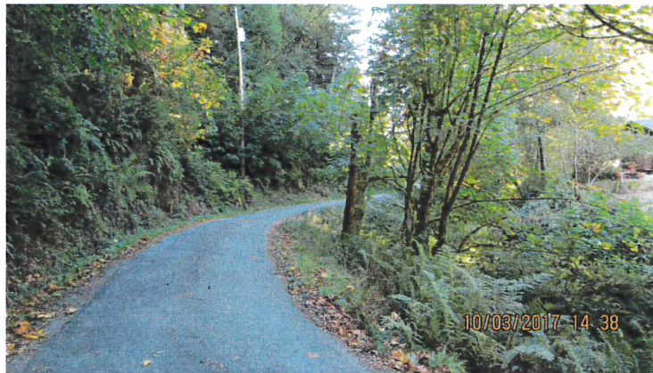
Photo 1664. Milepost 0.69. Single-lane section. Inadequate sight distance on S-curve owing to maple trees along Essex Gulch Creek.
