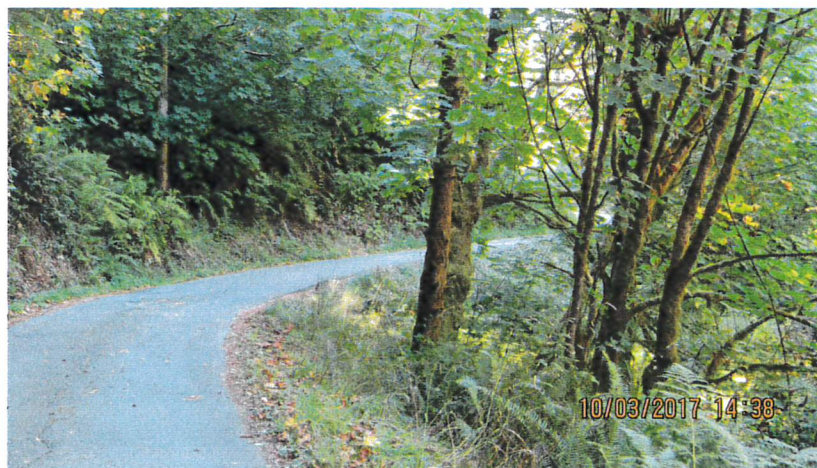
Photo 1665. Milepost 0.69. Single-lane section. Inadequate sight distance on S-curve owing to maple trees along Essex Gulch Creek.
