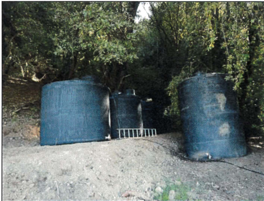
Figure 2. Current on site poly tank water storage. Approximately 30,000 gallons of storage.
