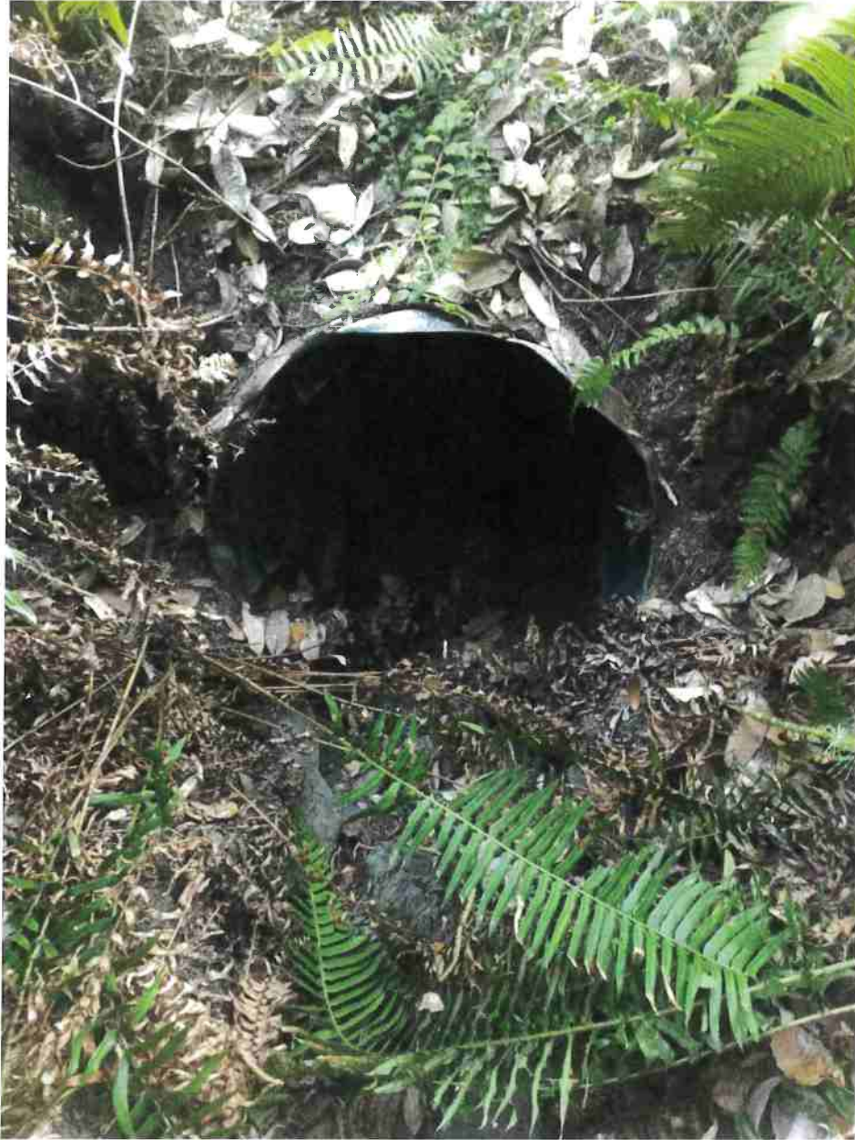
Photo 6: Crossing #1 inlet. Photo date 9-8-16
