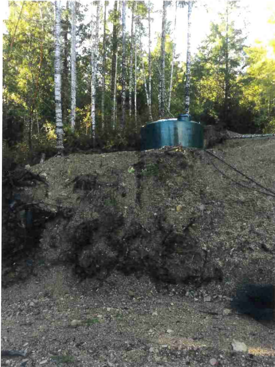
Photo 14: Erosion on fill slope of pad for 5,000 gallon water tank (Map Point F).
