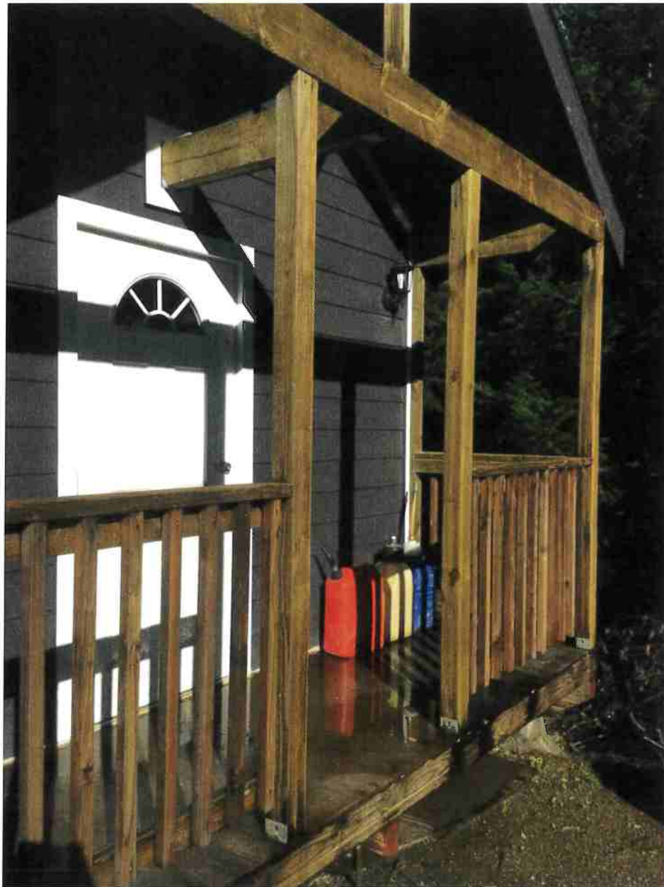
Photo 15: Petroleum storage. Photo date 1-24-17
