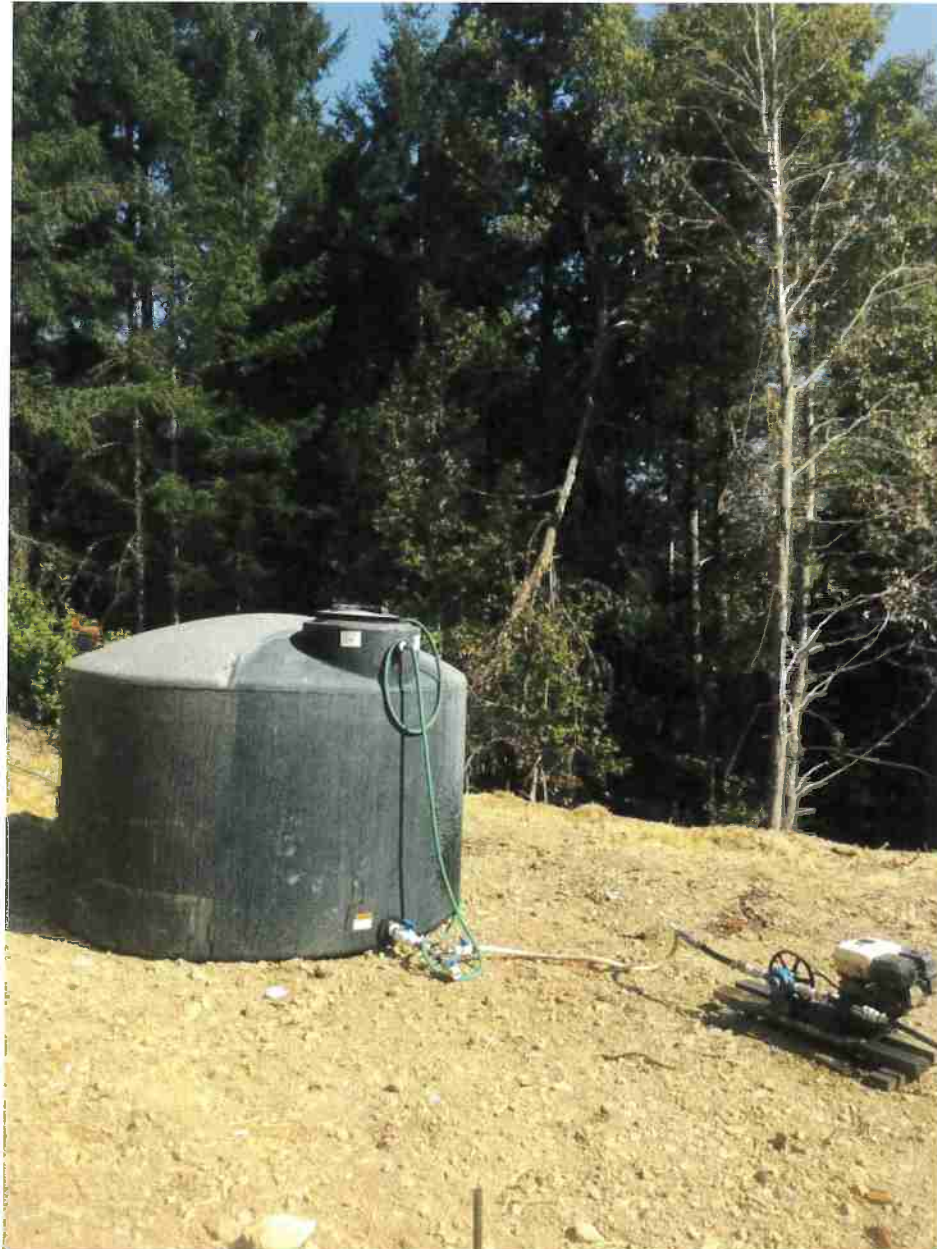
Photo 12: One 1,550 gallon poly storage tank. Photo date 9-8-16
