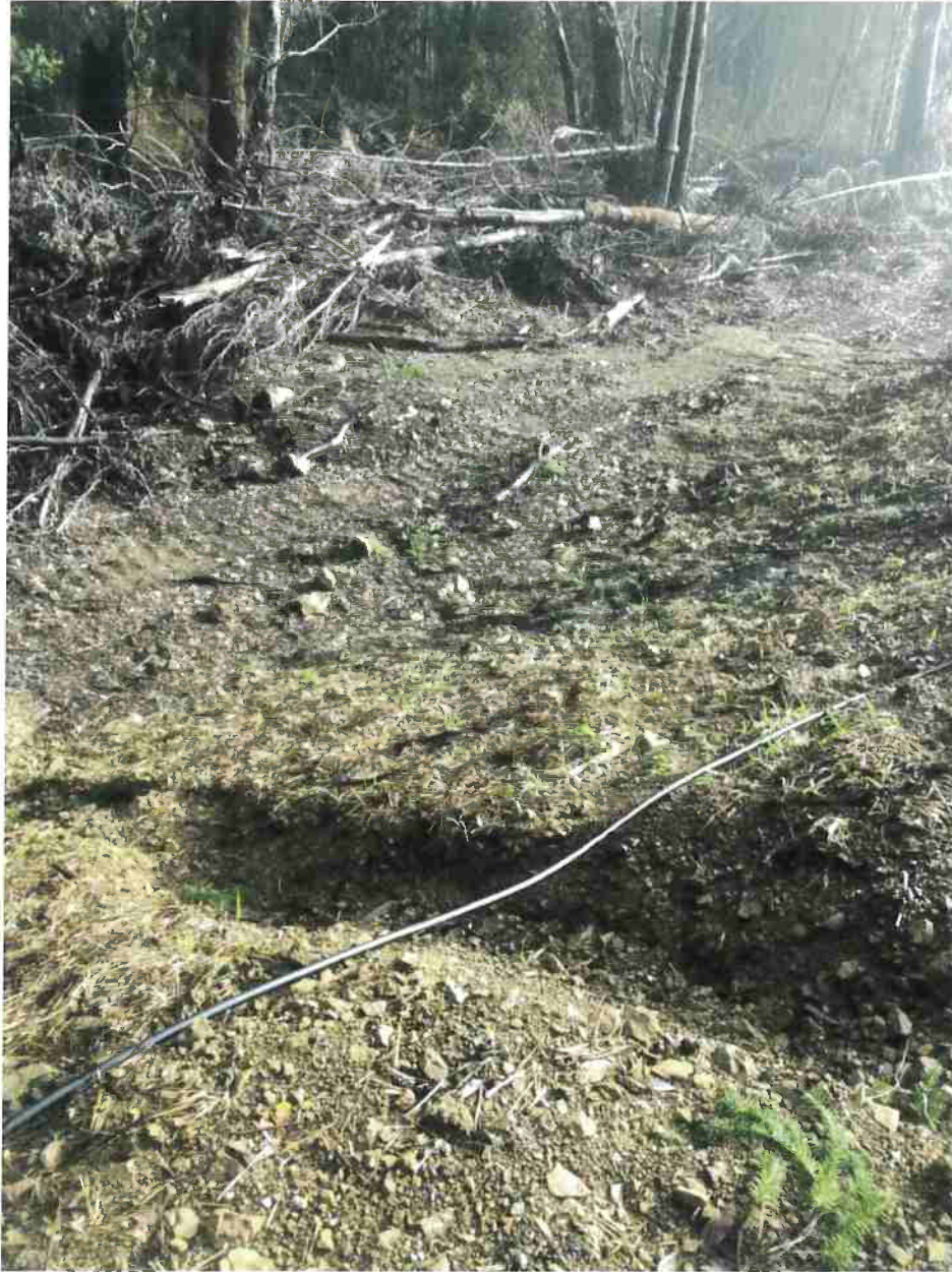
Photo 3: Erosion of fill slope of outdoor cultivation pad (Map Point C). Photo date 1-24-17
