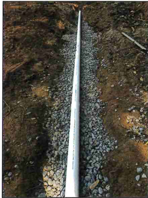
Figure 9 & 10: Septic Trench Length and Design
