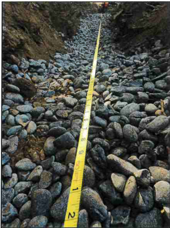
Figure 9 & 10: Septic Trench Length and Design
