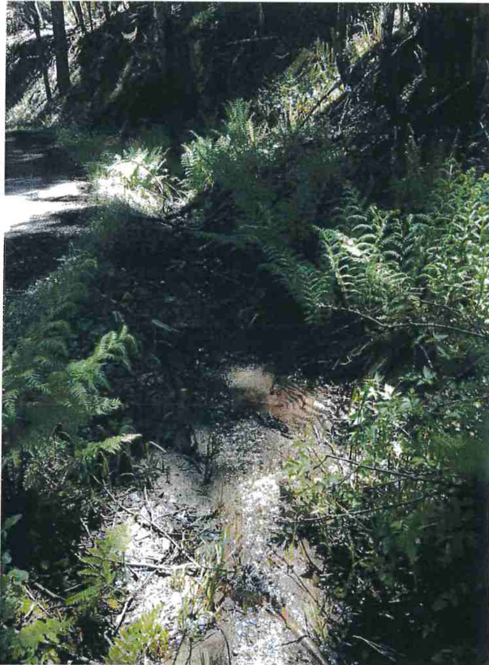
Picture 12: Inside ditch leading to the culvert at Crossing #1. The northern-most spring-fed Class II watercourse is intercepting the ditch at the bottom of the photo and flowing southerly to the 18-inch diameter aluminum culvert. This notification proposes to maintain the existing drainage pattern, but requires rock armoring of the inside ditch extending down to the new crossing proposed at Crossing #1. Photo date 5-21-2016.
