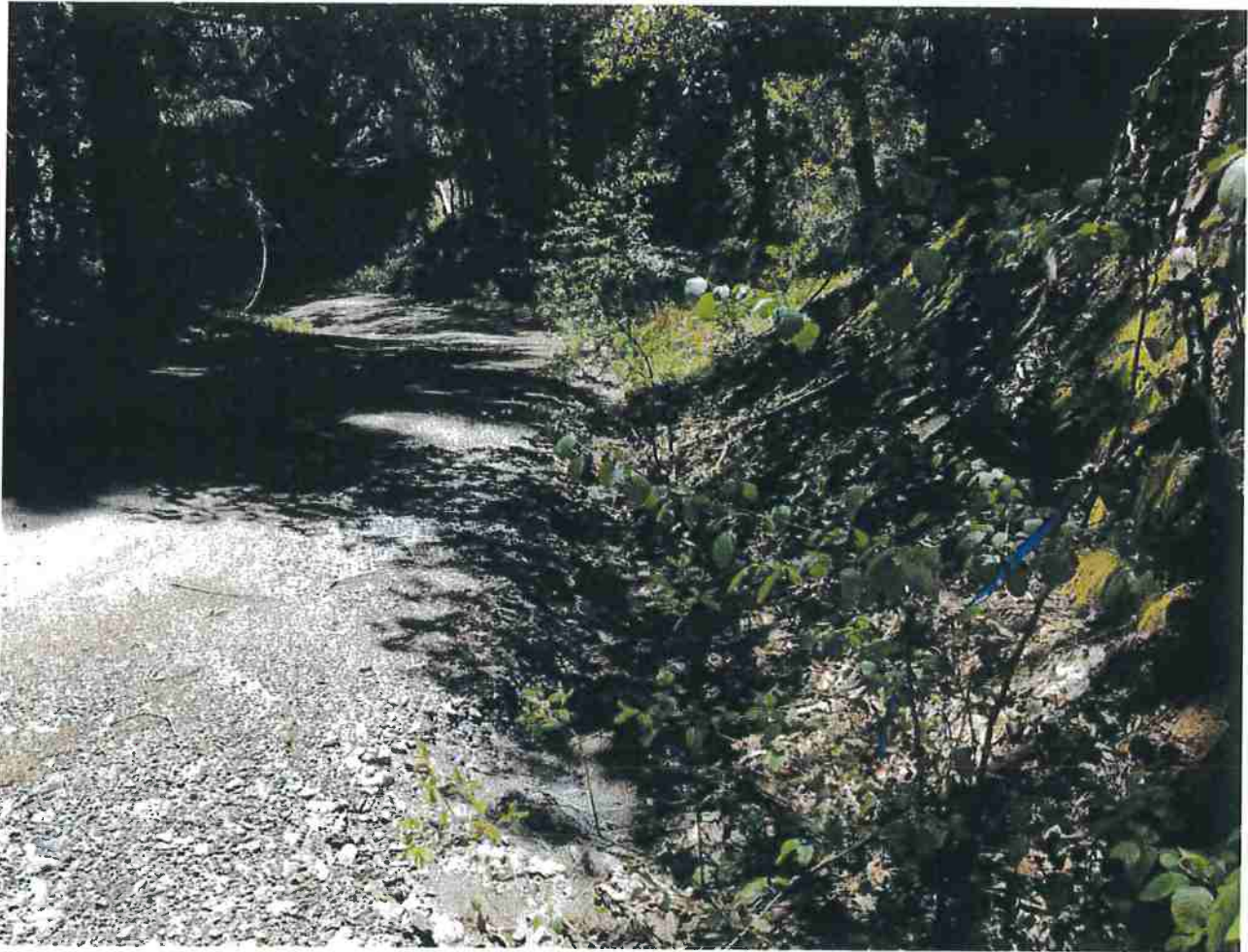
Picture 15: Inside ditch that is hydrologically connected to Crossing #1, which is in far distance. The blue flagging depicts the location of the inlet of DRC, which will disconnect the ditch from the watercourses. Photo date 6-15-2016.
