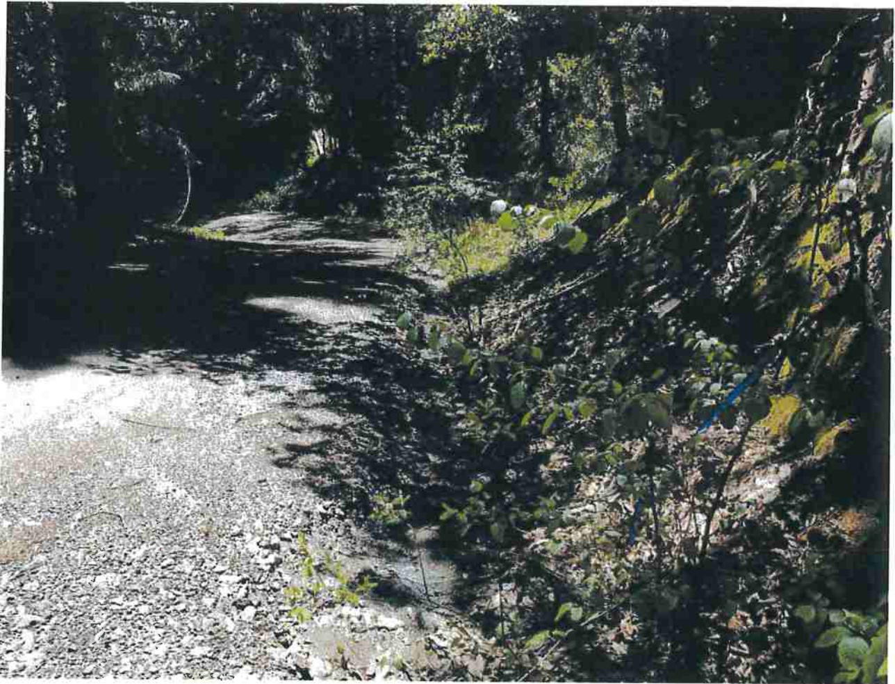
Picture 16: Inside ditch that is hydrologically connected to Crossing #1, which is in far distance. The blue flagging depicts the location of the inlet of DRC, which will disconnect the ditch from the watercourses. Photo date 6-15-2016.
