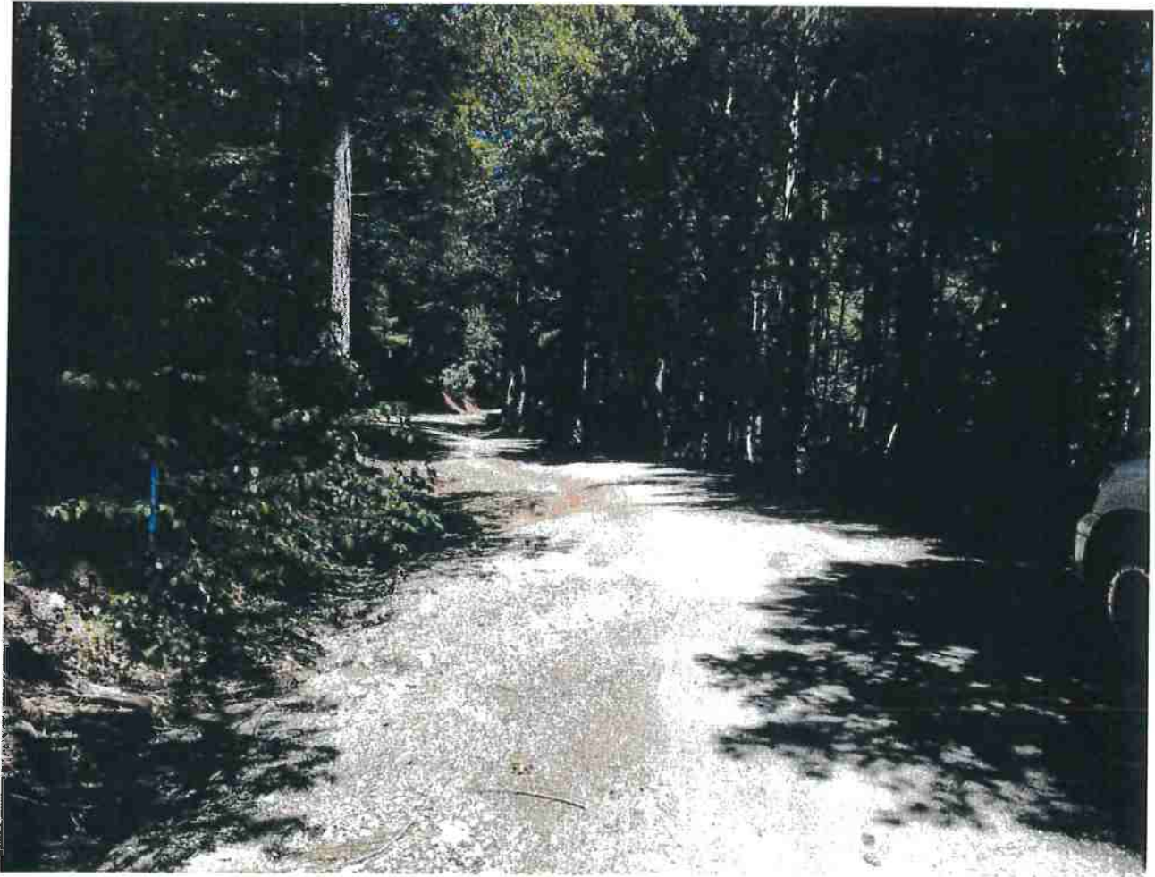
Picture 17: Inside ditch that is hydrologically connected to Crossing #1. This ditch extends northerly, unbroken for 500+ feet. The blue flagging depicts the location of the inlet of DRC, which will disconnect the ditch from the watercourses. Photo date 6-15-2016.
