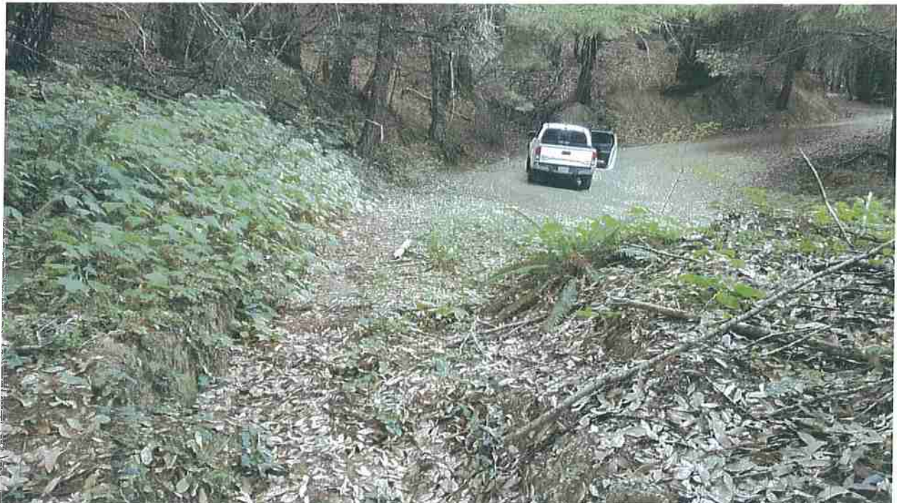
Looking up grade at Site 06. This leadout ditch and associated inside ditch has become filled with debris and sediment resulting in the diversion of ditch flows out of the ditch and further down grade, resulting in further erosion.
