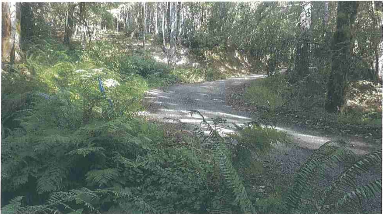
Looking up grade from the inlet of the watercourse crossing at Site 03. The existing culvert at this site will remain in place and the associated inside ditch draining to the inlet will be filled in to prevent diversion into the existing culverts inlet.
