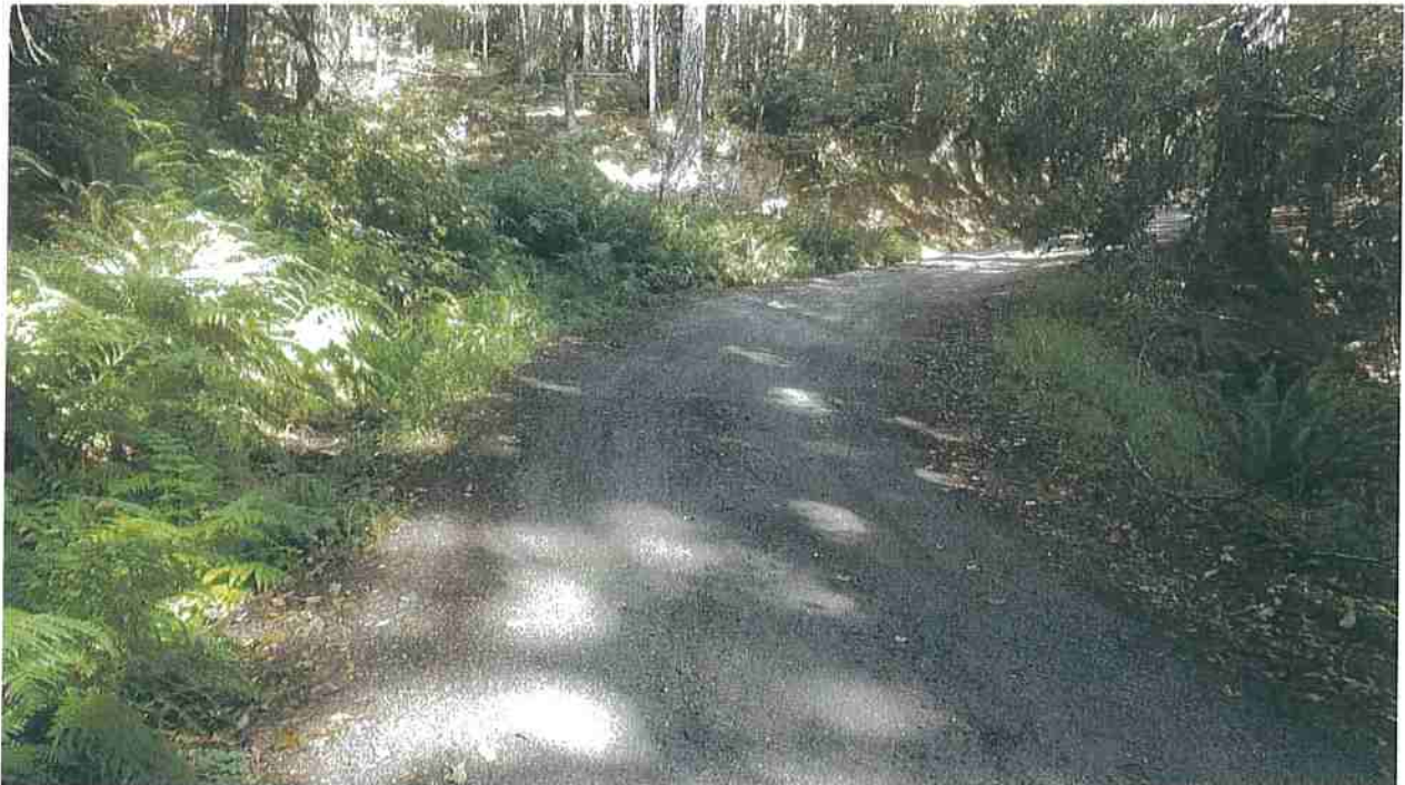
Looking up grade from Site 03 towards Site 02. A spring and associated flows (Class II watercourse) intercept the vegetated inside ditch in the upper left of the photo. The current condition is acceptable and does not require treatment. The inside ditch from where the Class II watercourse intercepts the inside ditch to Site 02 will be cleared of debris and sediment to ensure total capture of the watercourse.
