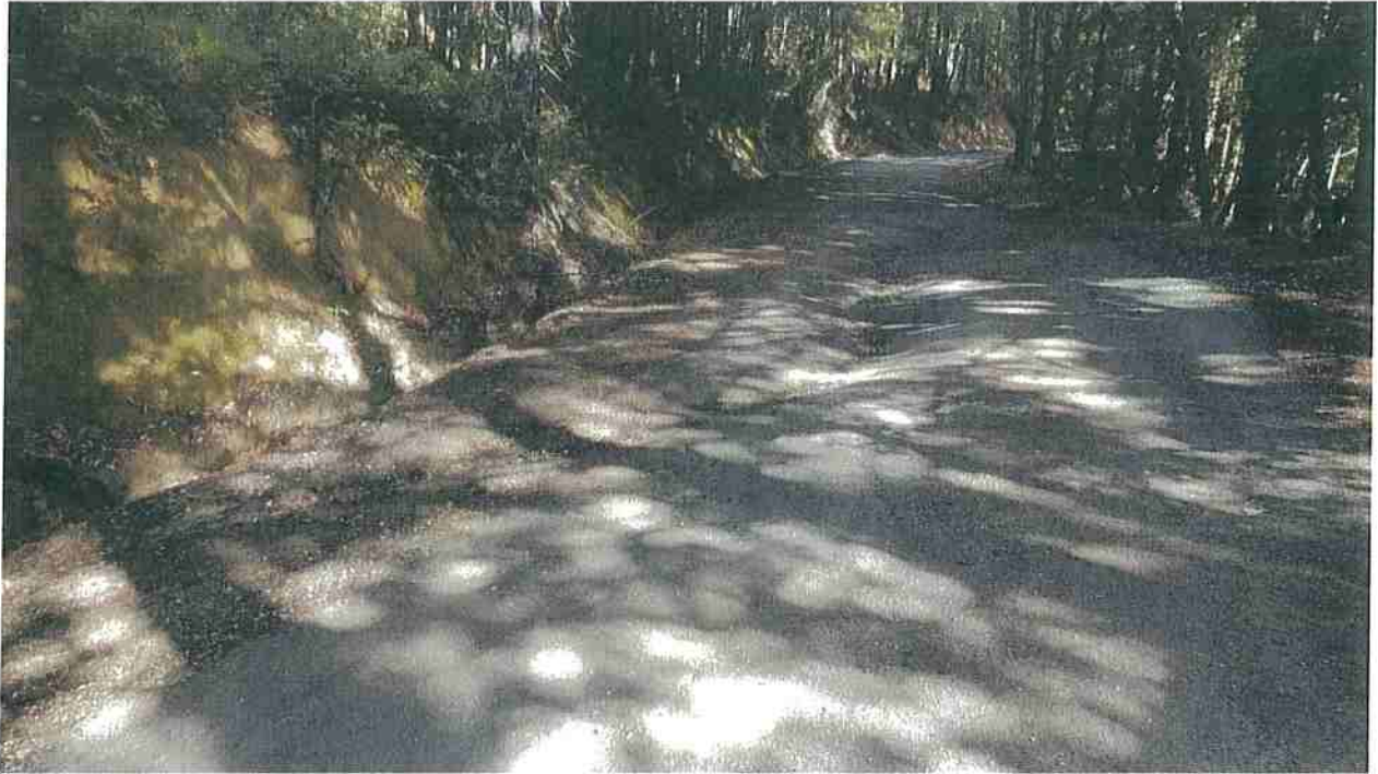
Looking up grade from Site 02. Note road surface erosion.
