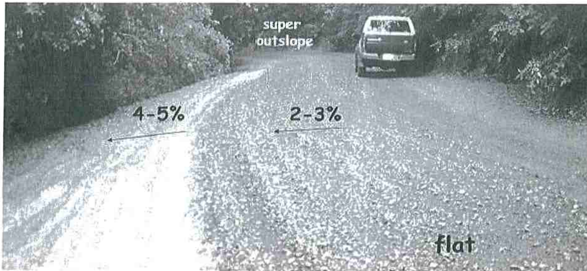
FIGURE 29. Road shape changes as the road travels through the landscape. For example, an out-sloped road will have a steep or "banked" outslope through inside curves, a consistent outslope through straight reaches and a flat or slightly insloped shape as it goes through an outside curve. The road may have an outslope of 2-3% across the travel surface while the shoulder is more steeply outsloped to ensure runoff and sediment will leave the roadbed.
