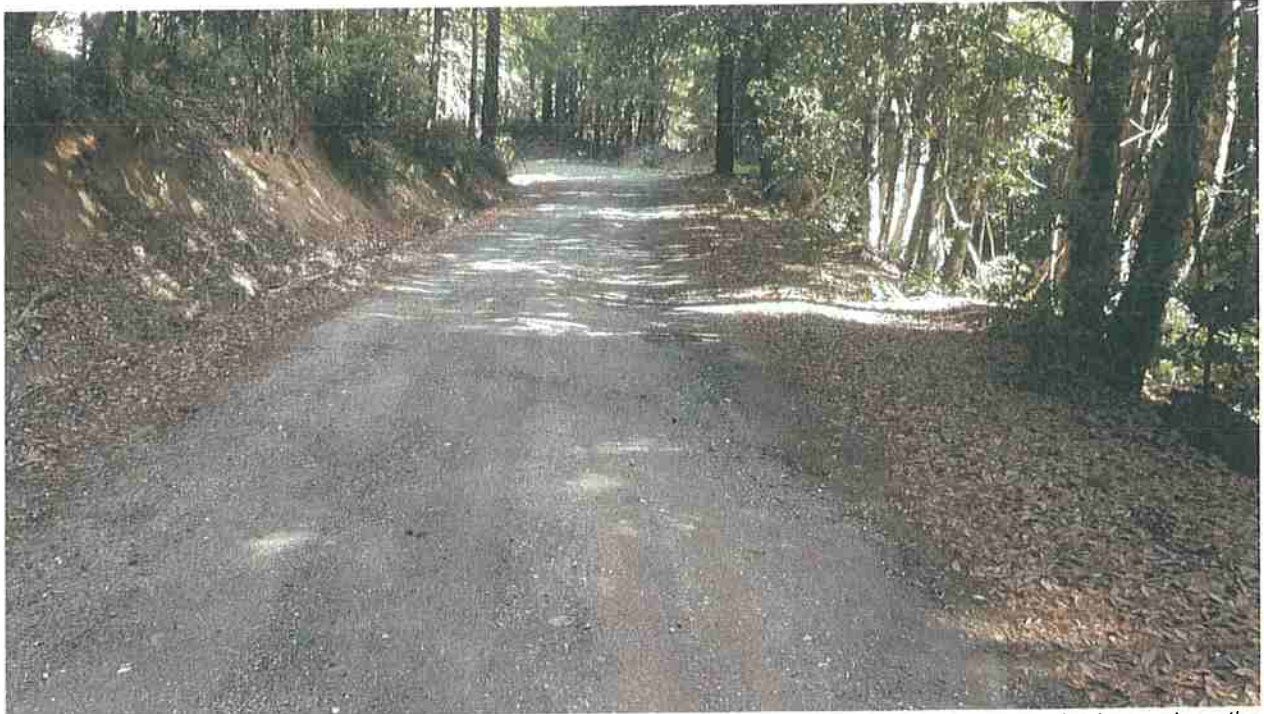
Looking up grade of Site 01. Road surface runoff is being constrained to the road tread path by the berm along the outboard edge of the road, resulting in road surface erosion here and further down grade along with sediment discharge to surface waters.
