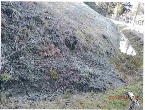
Figure 11: Cutbank slide depositing sediment into the ditch. Photo taken facing south.
