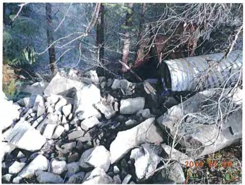
Figure 8: Outfall of STX-10. 22" corrugated metal culvert.
