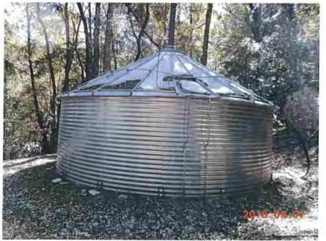
Figure 12: Restoration Site #1. 1,400 ft<sup>2</sup> graded flat containing 25,000-gallon rainwater catchment tank.
