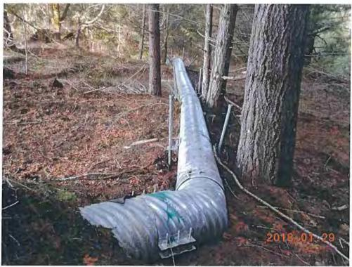
Figure 7: Downspout of STX-10. The downspout is approximately 105 feet long.
