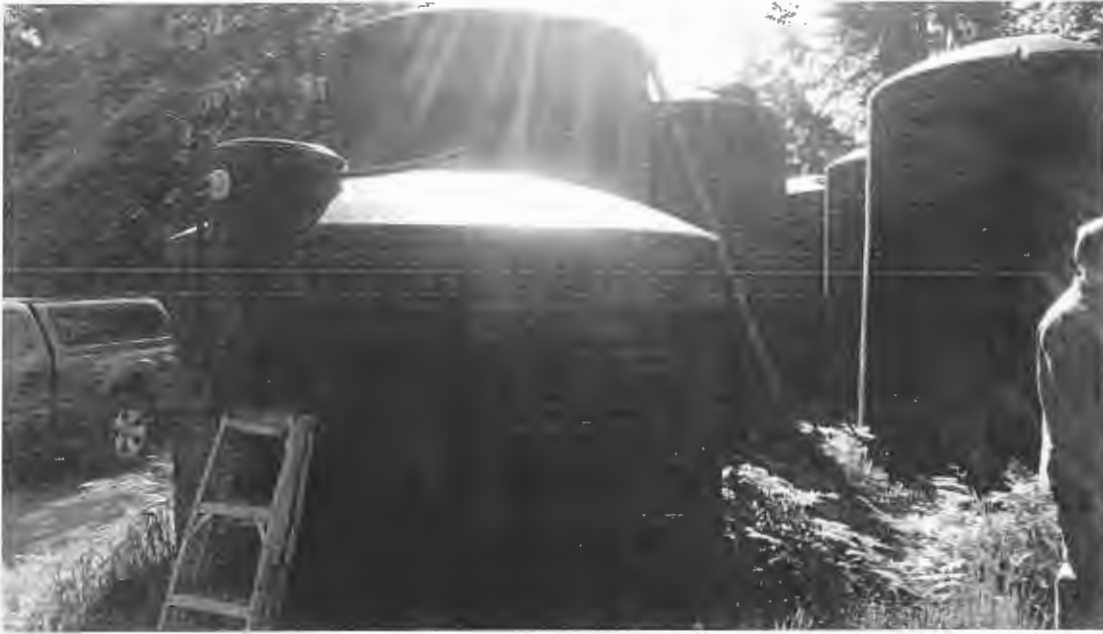
Water Storage: 2,500-gallon hard plastic water tank.
