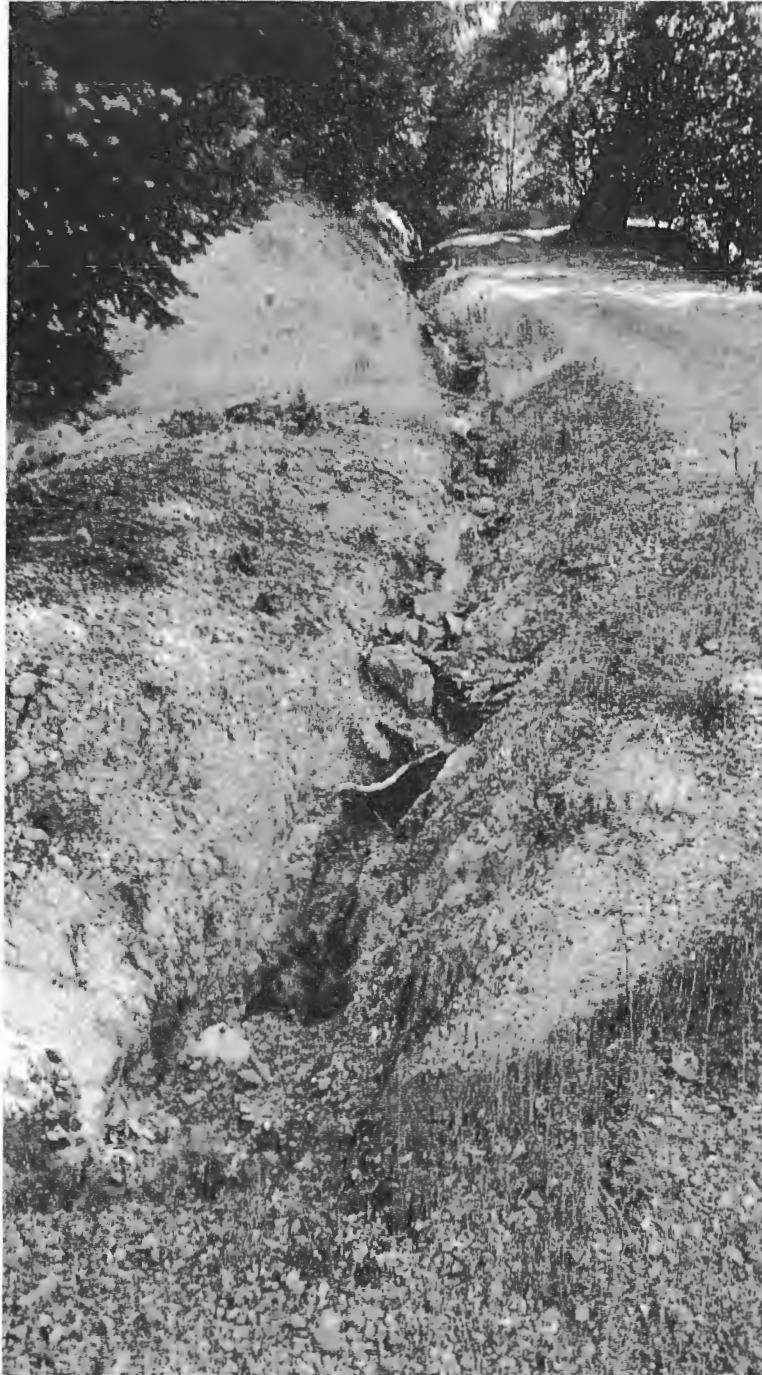
Inside ditch: Looking upstream at the inside ditch on the seasonal road, this feature drains the road from Site 03 to Site 06.
