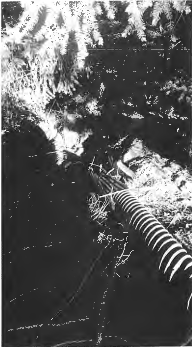
Site 11: The outlet of the inside ditch relief culvert from the seasonal use road.
