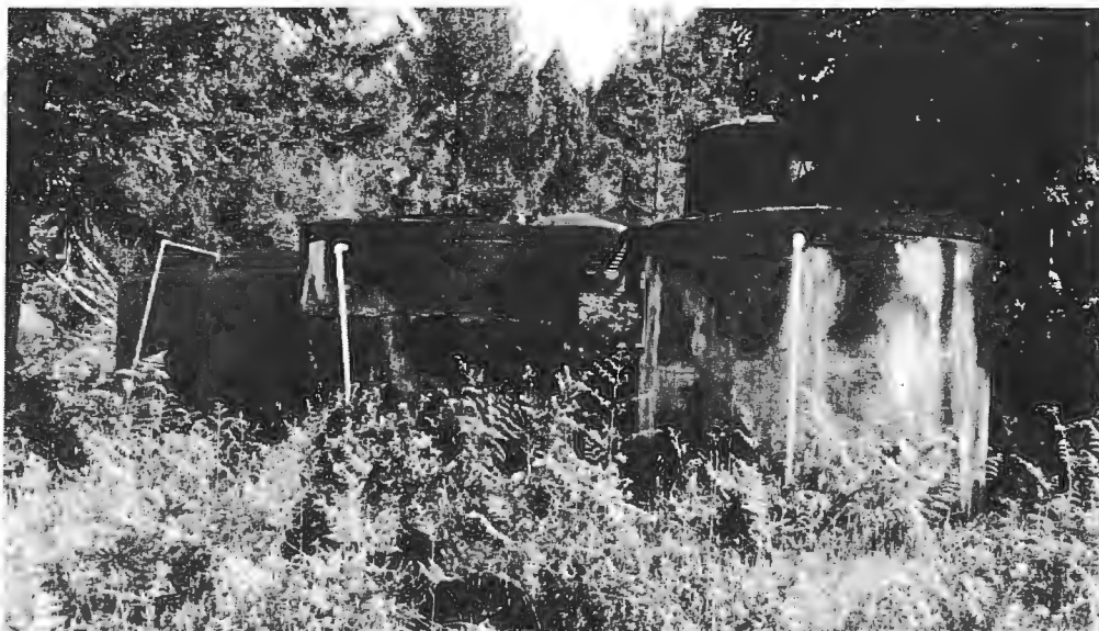
Water Storage: Two 1,300-gallon cement & two 500-gallon plastic water storage tanks.
