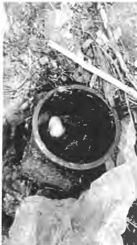
Point of Diversion: POD 10" diameter by 12" long plastic perforated bucket plumbed with a 3' long 3" PVC pipe that transitions into a 1 ½ "polyline.
