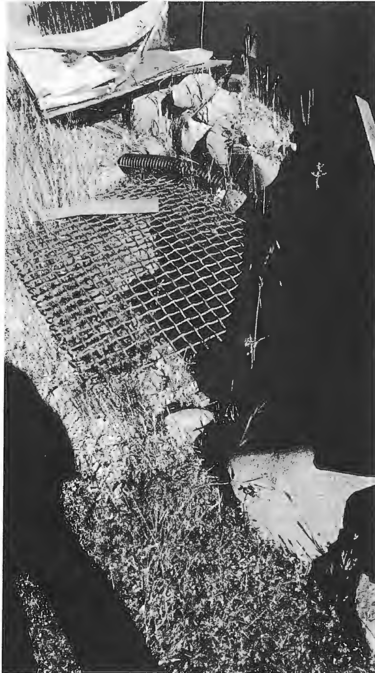
Site 06: Imbedded 2' x 3' cement structure that transitions the ditch relief culvert into a 12" diameter 40' CMP culvert located at the southwest corner of the 20,000-gallon water storage structure.
