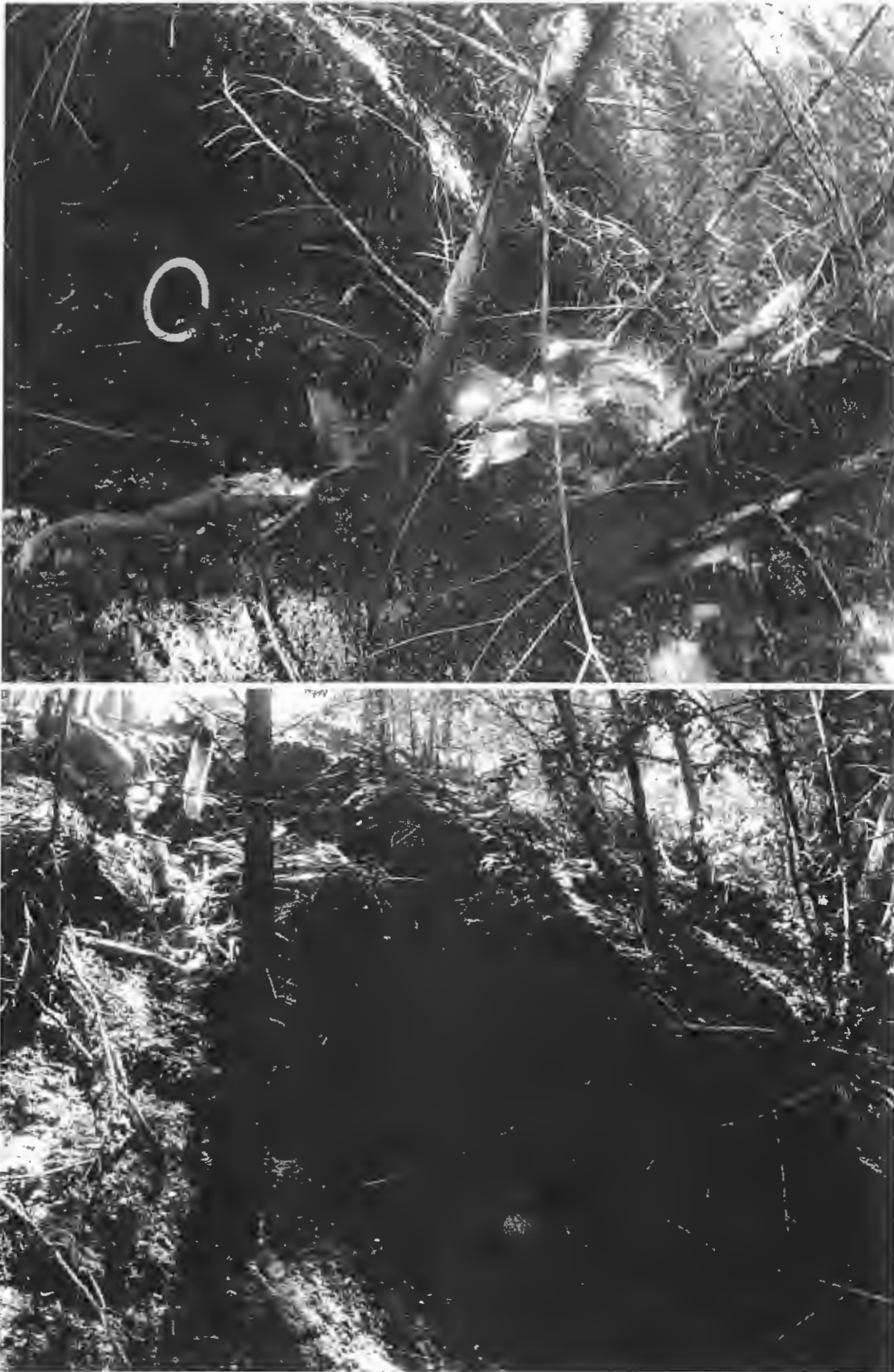
Site 11: This gully feature is created by a DRC that drains approximately 600ft of inside ditch. Multiple ditch relief culvert locations have been recommended which will de-water this feature. All loose debris and car chassis within the gully feature shall be removed.
