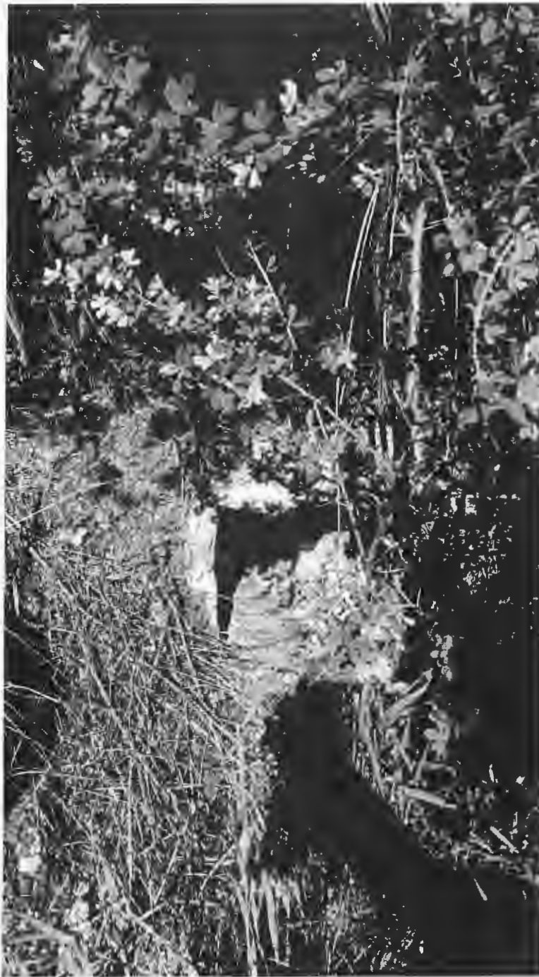
Site 07: The inlet of the 12" diameter by 6' long CMP culvert collecting surface runoff from the graded area around Site 06. This culvert shall be removed including the bank in which it lies. The road surface above the culvert shall have water bars installed to hydrologically disconnect surface runoff from the downstream Class III watercourse.
