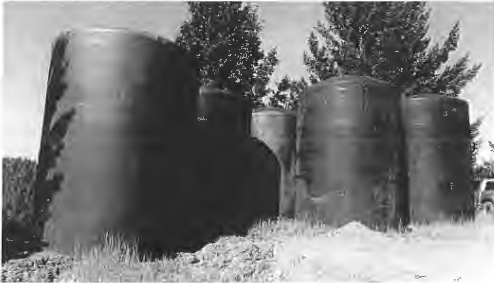
Water Storage: Five 5,000-gallon hard plastic storage tanks.
