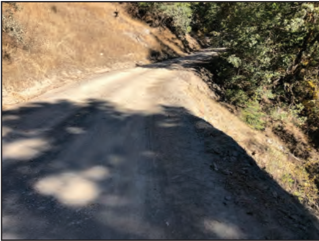
Photo #115 River Rd Looking East @ Narrowed Curve Area w/ Tire Tracks Over Eroded Area
