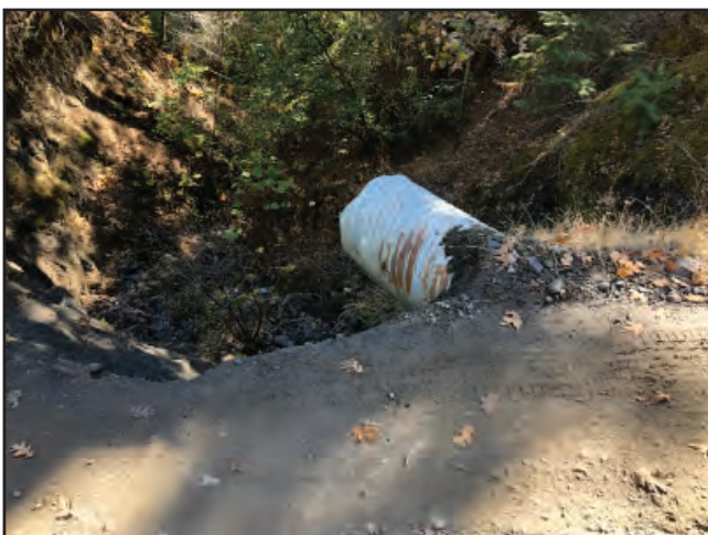
Photo #89 River Rd Looking @ 24" Culvert Out
