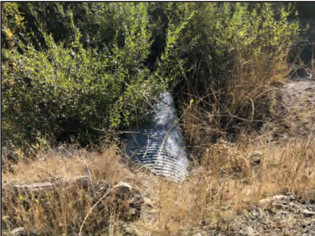
Photo #15 River Rd Looking @ 36" Culvert In
