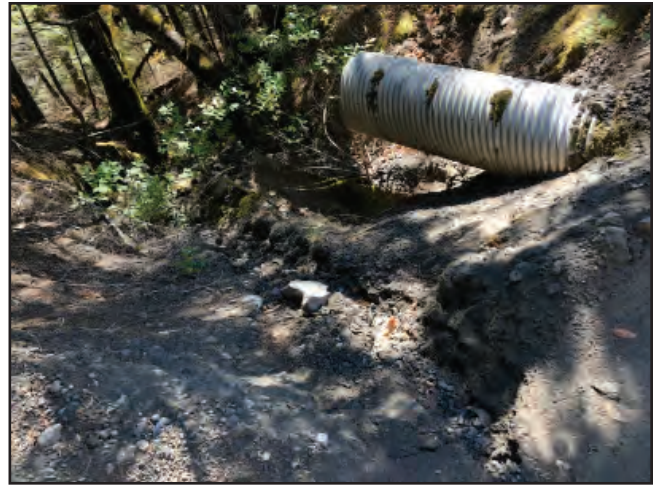
Photo #110 River Rd Looking @ 36" Culvert Out
