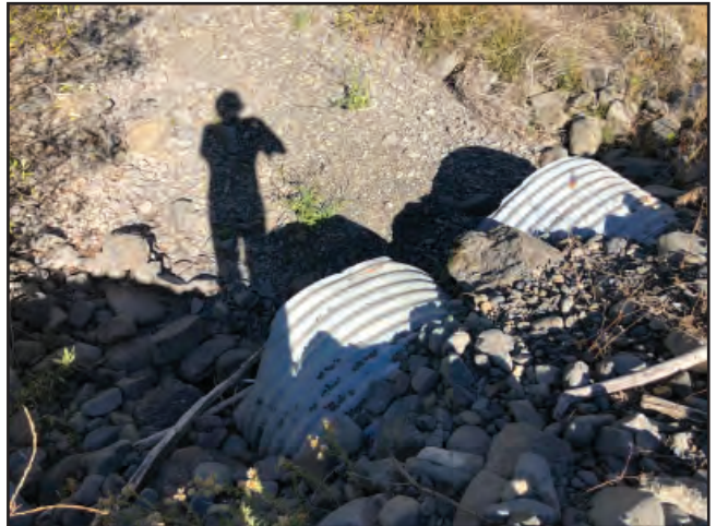
Photo #16 River Rd Looking @ Dual 36" Culverts Out
