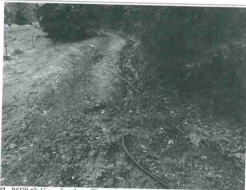
Photo 5, MP #2 - RSDP #2. View of road runoff becoming concentrated and forming a gully along Road 4 downslope from CA #2.
