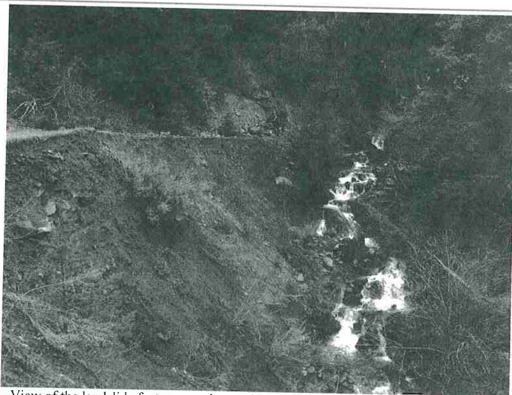
Photo 7, MP #3 –View of the landslide feature on a legacy landing with a probable blown crossing, at the end of Road 3. Note the Class II watercourse potential to scour and undercut the channel banks.
