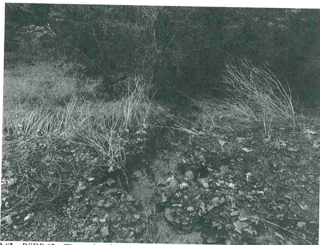
Photo 6, MP #2 – RSDP #2 – The road surface discharge point off Road 4 that originated from Road 3 (Photos 3-5 above). This gully discharges onto an area with a low risk of sediment delivery to surface waters.
