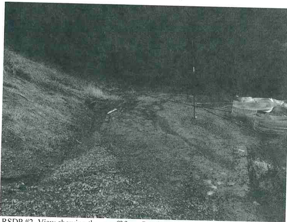
Photo 3, MP #2 - RSDP #2. View of gully coming down Road 3 and continuing onto Road 4, past Cultivation Area (CA) #1. The flow path appears to be originating primarily from the adjacent, upslope, and off parcel cultivation activities.
