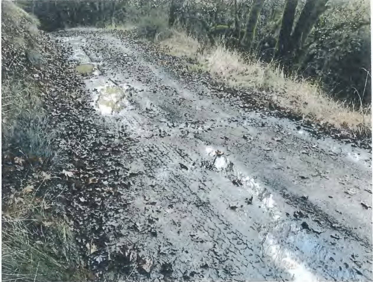
Photo #1: This image shows the surface erosion occurring on the main access road to the property. This main access road will have a fresh layer of crushed rock applied to the surface. Photo Date: 11/14/2017.
