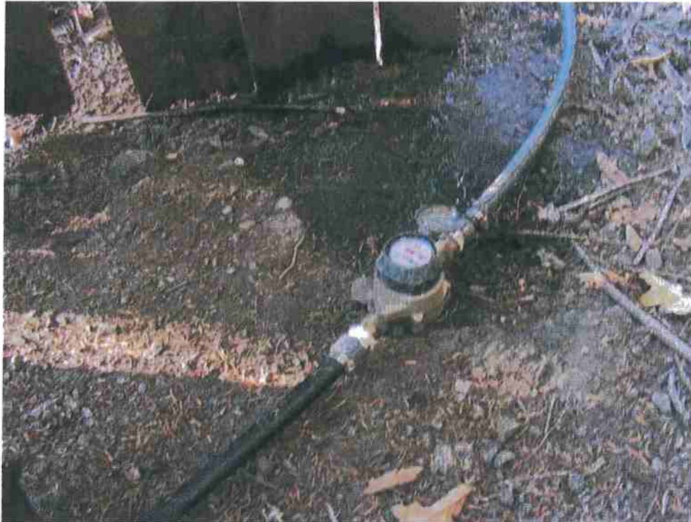
Watermeter in place at POD-1
