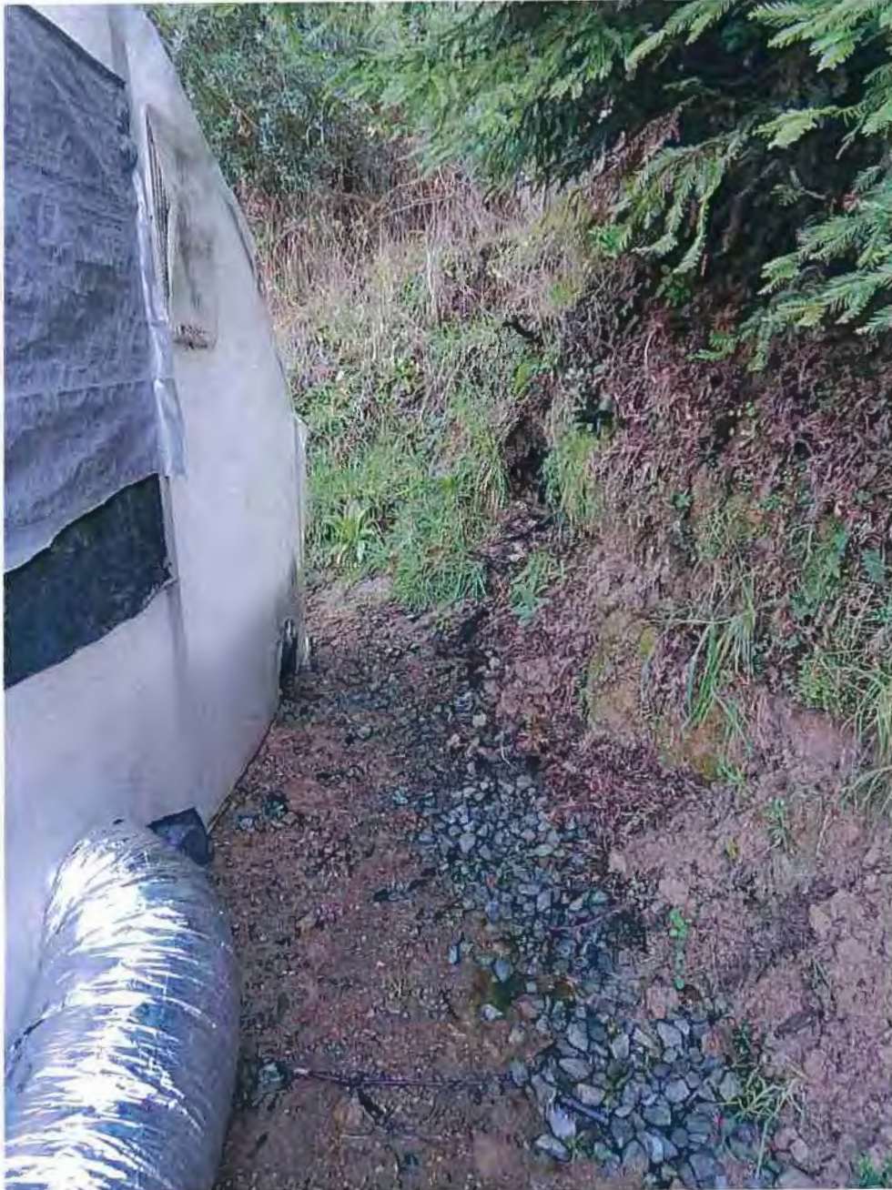
Picture 3. Seep daylighted in the southeast corner of second terrace
