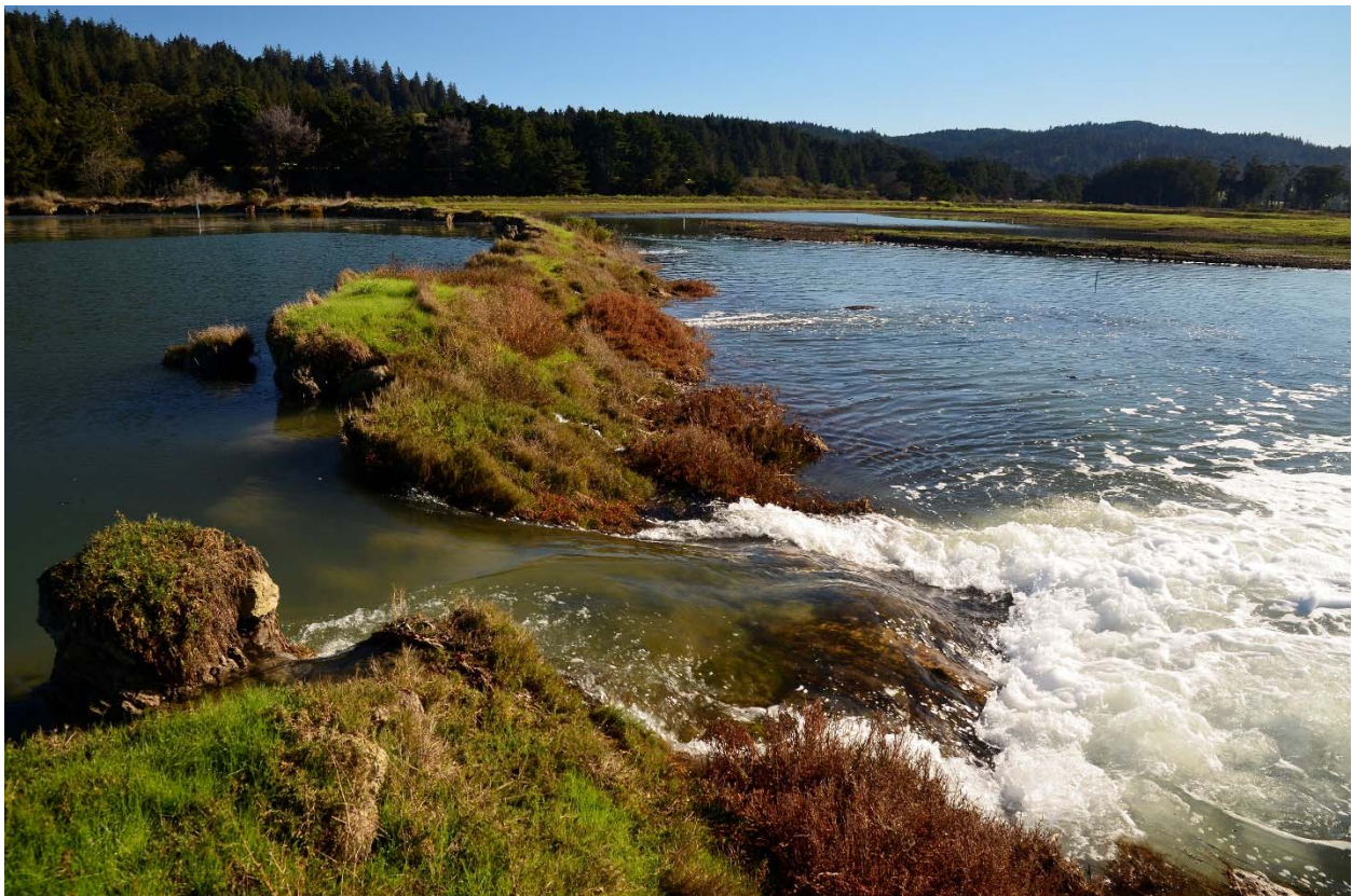
Figure 2. Dike overtopped during a king tide tidally inundating low-lying lands on South Bay.
