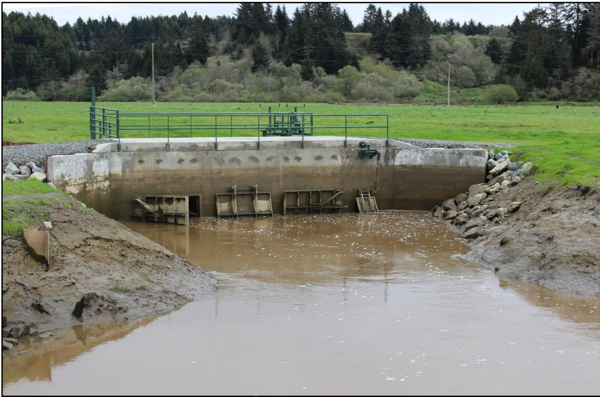
Martin Slough Tide gates, downstream side, showing the three 6' x 6' gates on the center and left and the 2' x 2' "habitat door" on the right.
