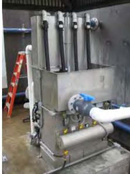
Figure B. Fluidyne™ Cloth Media Filter System with four media elements.
